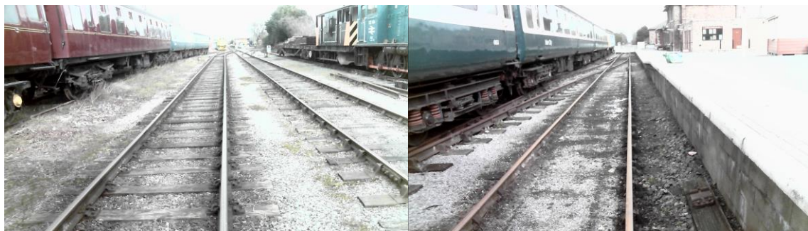
Figure 7. 25: Forward facing images of track sections exposed to sun (L) and a shaded sections towards the platform (R)
