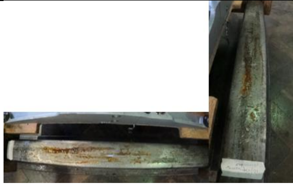
Figure 6. 23: Example of railhead images for rust day5 + water spray. Horizontal with camera-railhead distance \approx 1450\text{mm} (L) and vertical with camera-railhead distance \approx 1000\text{mm} (R) (10-05-22)
