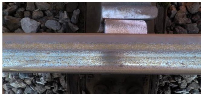
Figure 6. 35: Example of railhead image capture in-field
