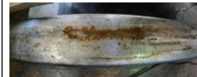
Figure 6. 19: Example of railhead images for rust day3 + reduced water spray. Horizontal with camera-railhead
