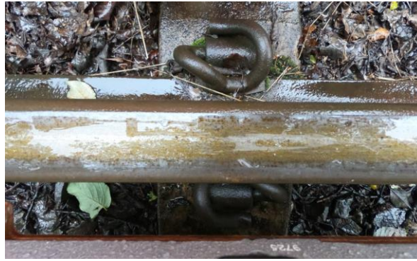
Figure 6.36: Image of wet railhead captured in field
