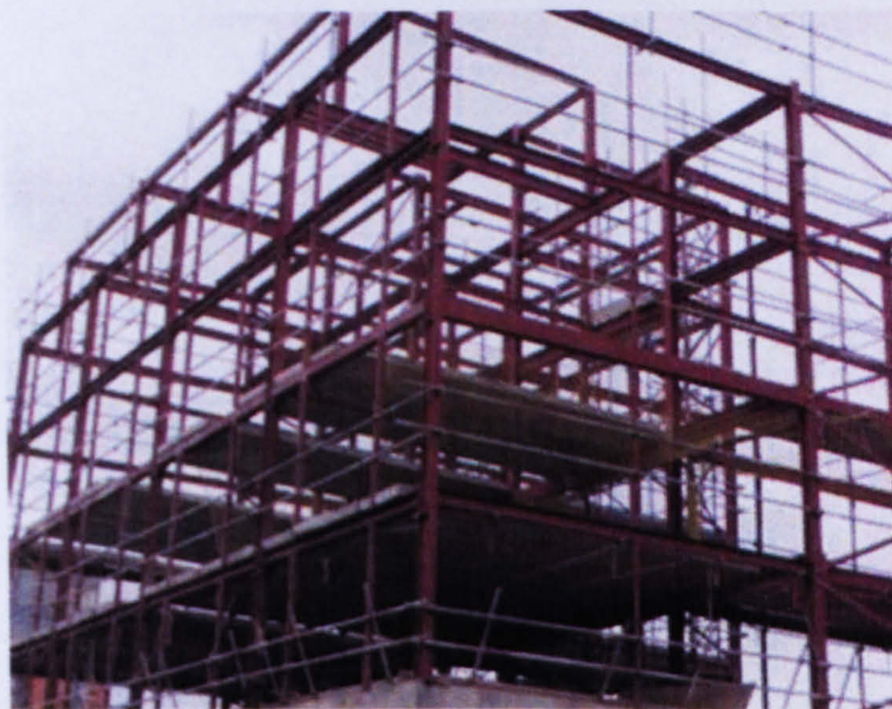
Figure 5-2 Construction Site b -Sheffield (photographed in 2004)
