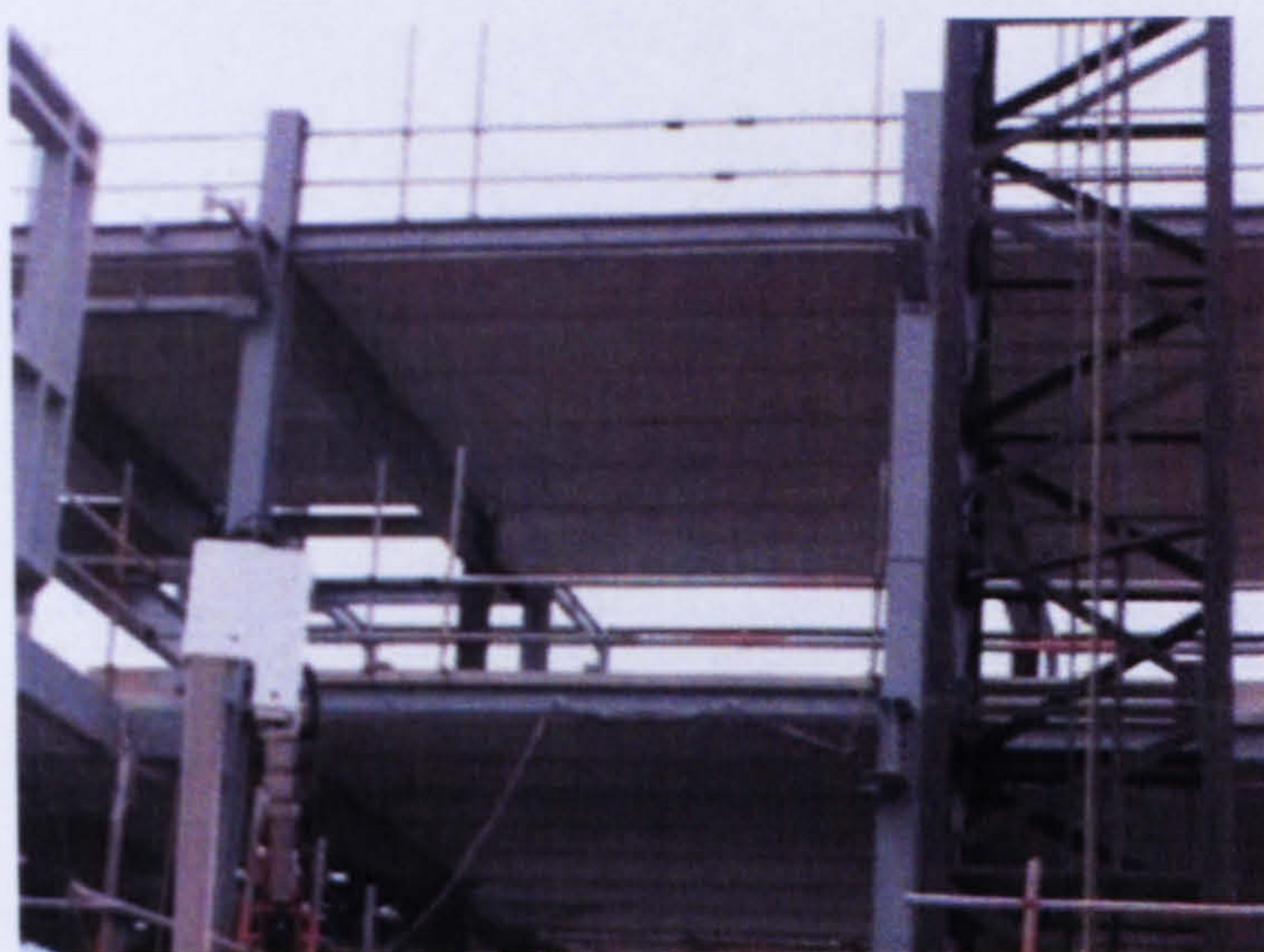
Figure 5-1 Construction Site a -Sheffield (photographed in 2004)
