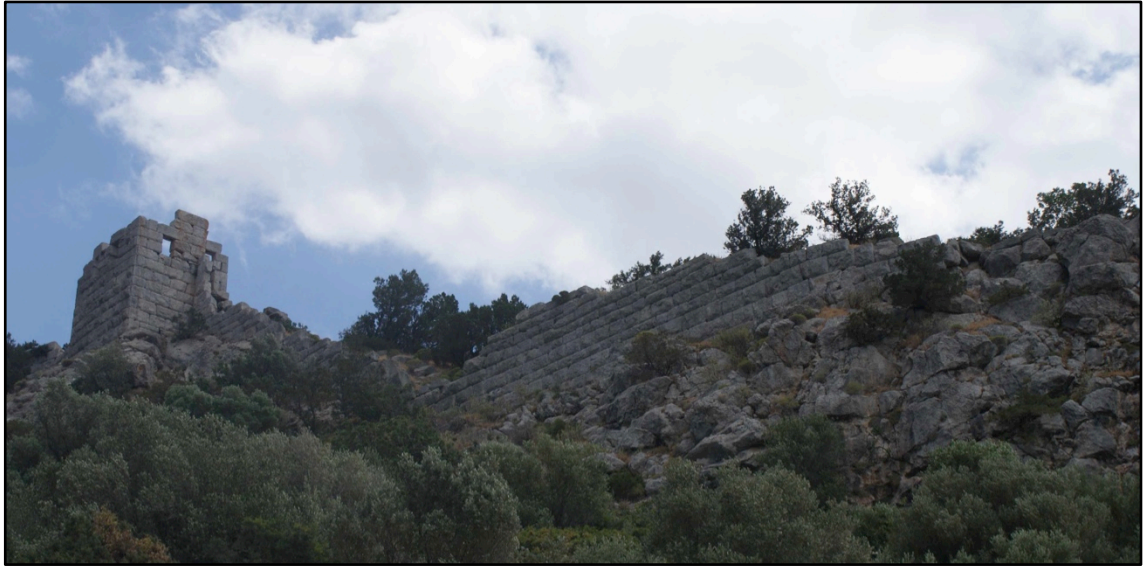
Fig. 2.1: Siphai, view of fourth-century walls from the west
