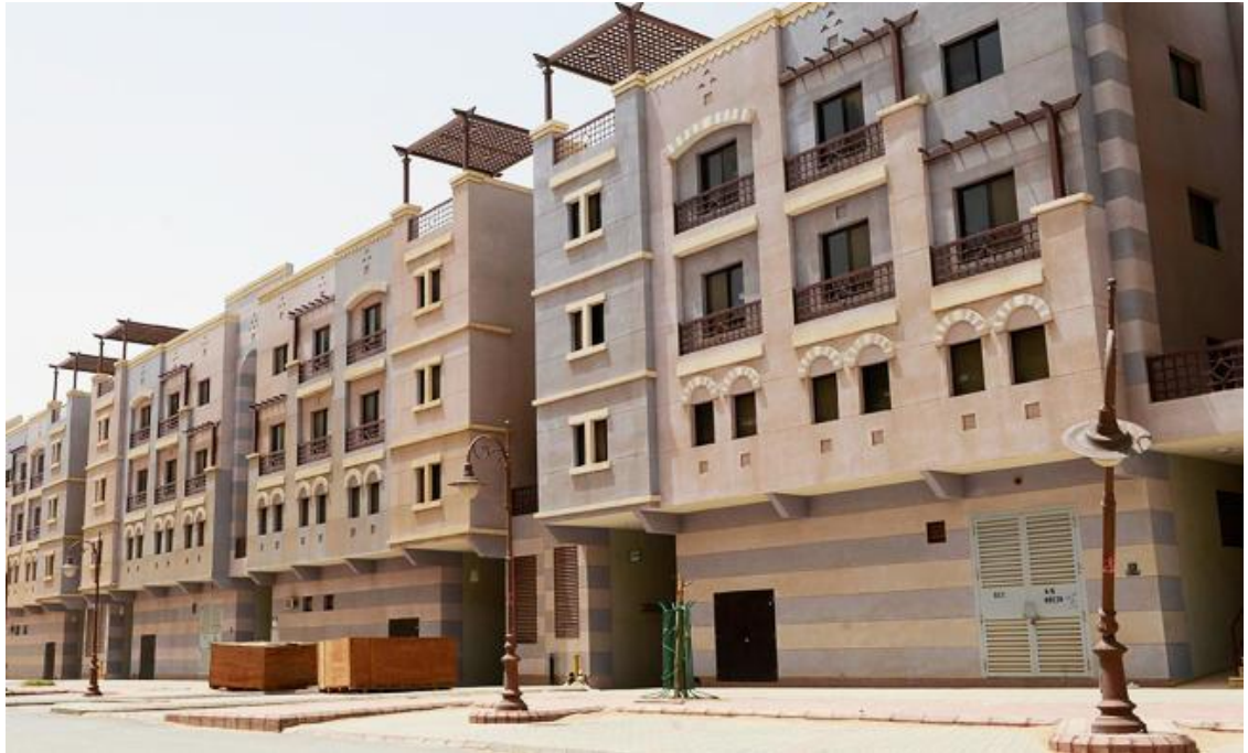
Figure 3-11 Typical apartments in Saudi Arabia (Arab News, 2020)
