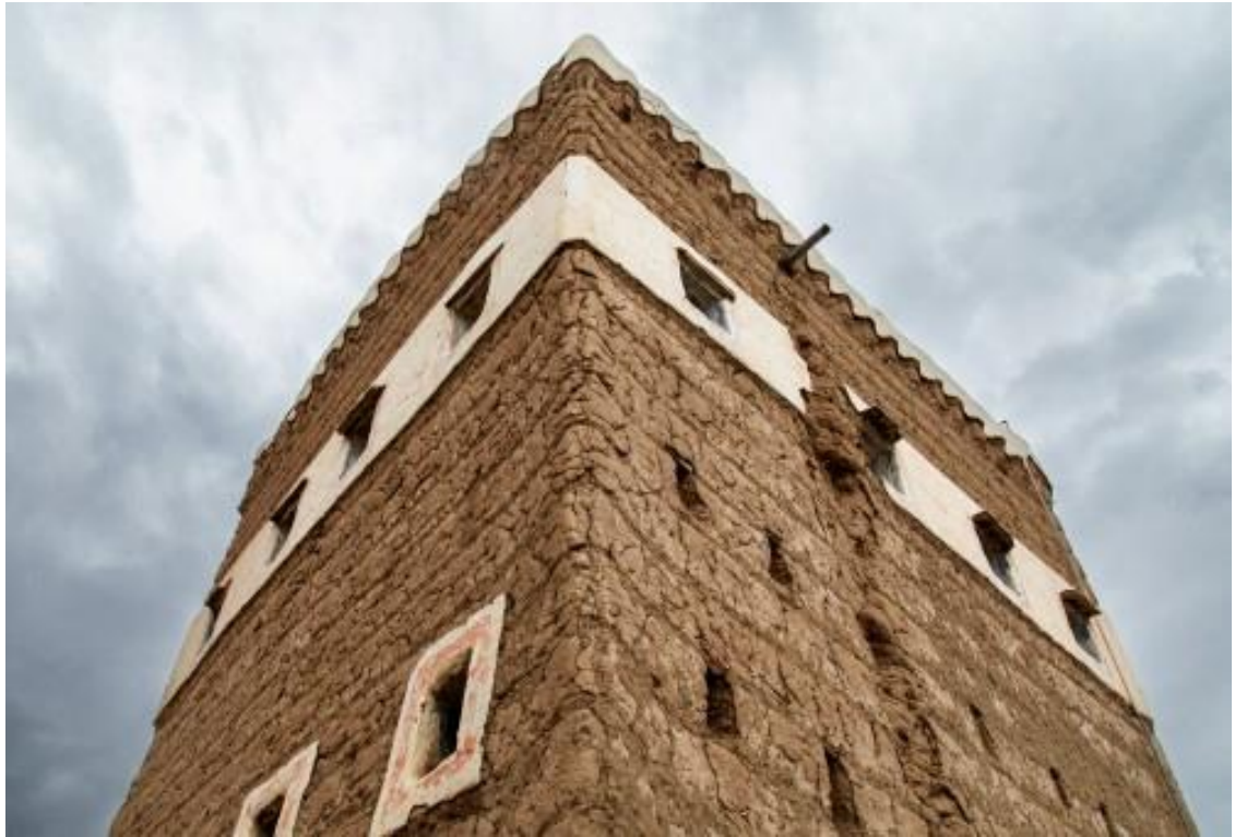
Figure 3-10 Asir Region Building Materials Stone and Mud Wall (Altaledi, n.d)
