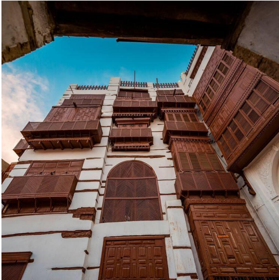
Figure 3-4 Vernacular Architecture Style of Hijaz Region (World Heritage Convention, n.d)
