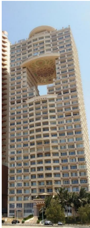
Figure 3-13 Typical high residential building in Saudi Arabia (Susie of Arabia, 2017)
