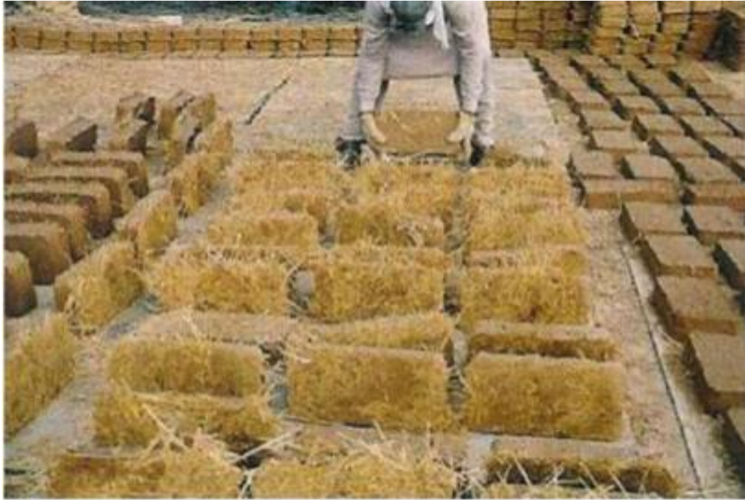
Figure 3-9 Najd Region Building Materials (Mortada, H., 2016)
