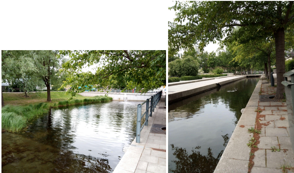
Figure 25 and 26. Storm water basin and channel with filtration to the Hammarby Lake
