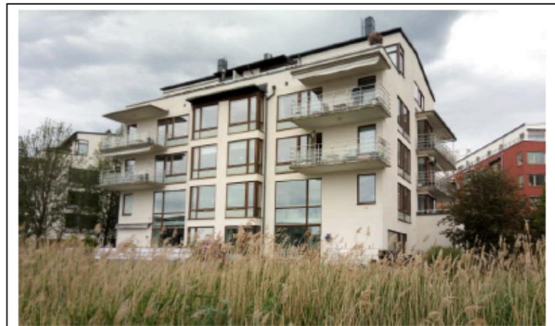
Solar cell on the roof of JM's block, Fjarden, providing electricity used in the communal areas.
