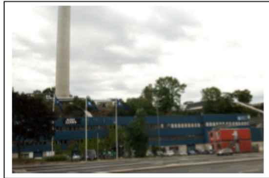
Biogas Production Facility.
