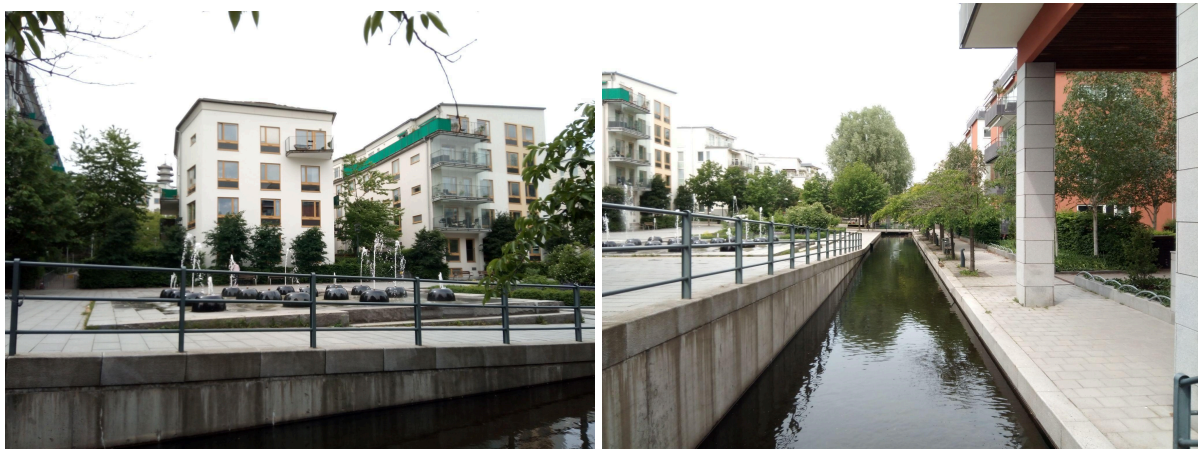
Figure 23 and 24. Green roofs and yards to collect rainwater; and channel to collect stormwater
