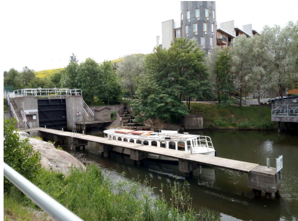
Figure 20. Salmon ladder and lock
