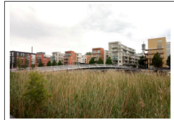
Footbridge made from stainless steel for long term durability.
