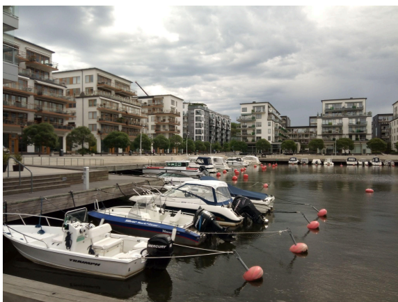
Figure 19. Restored quay to form a footpath and cycle route
