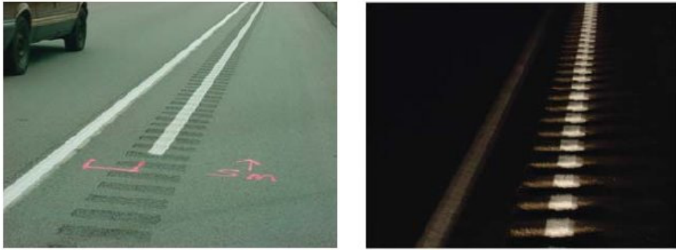
Figure 2.6 Night-time visibility of line marking within the rumble strip, taken from (FHWA, 2015).
