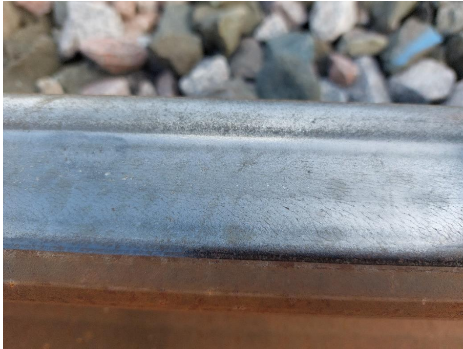
Figure 43: Condition of HP335 rail surface prior to grinding action at Drax Power Station, showing snakeskin-like asperities on the rail head.
