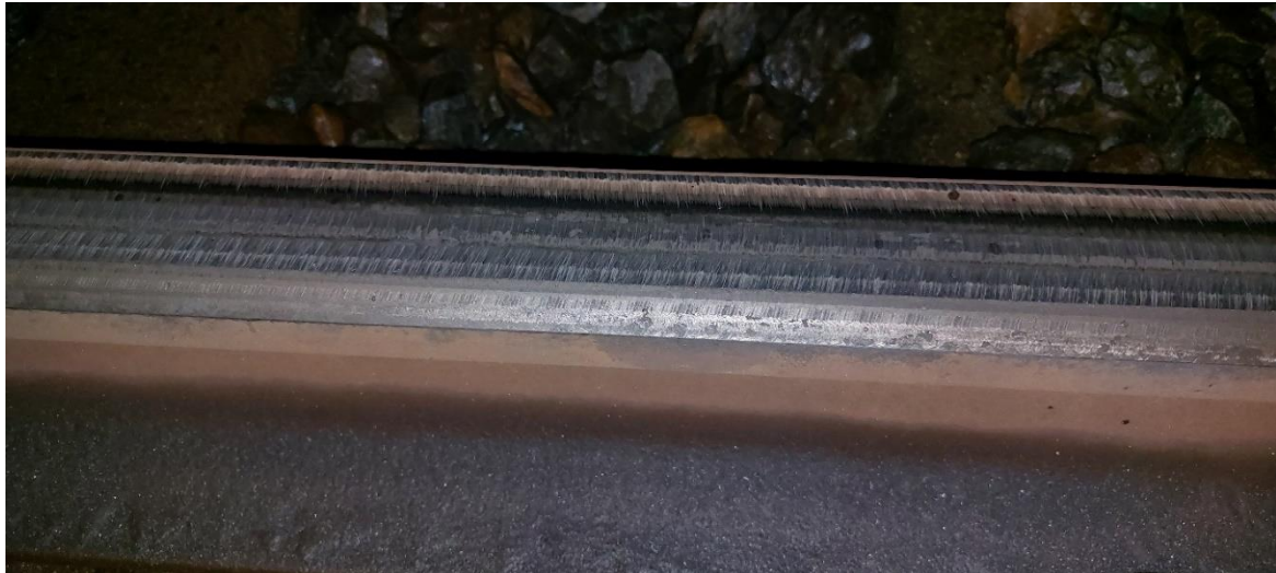
Figure 39: The mid-grind condition of the railhead during the grinding operation at Metro dé Medellín.
