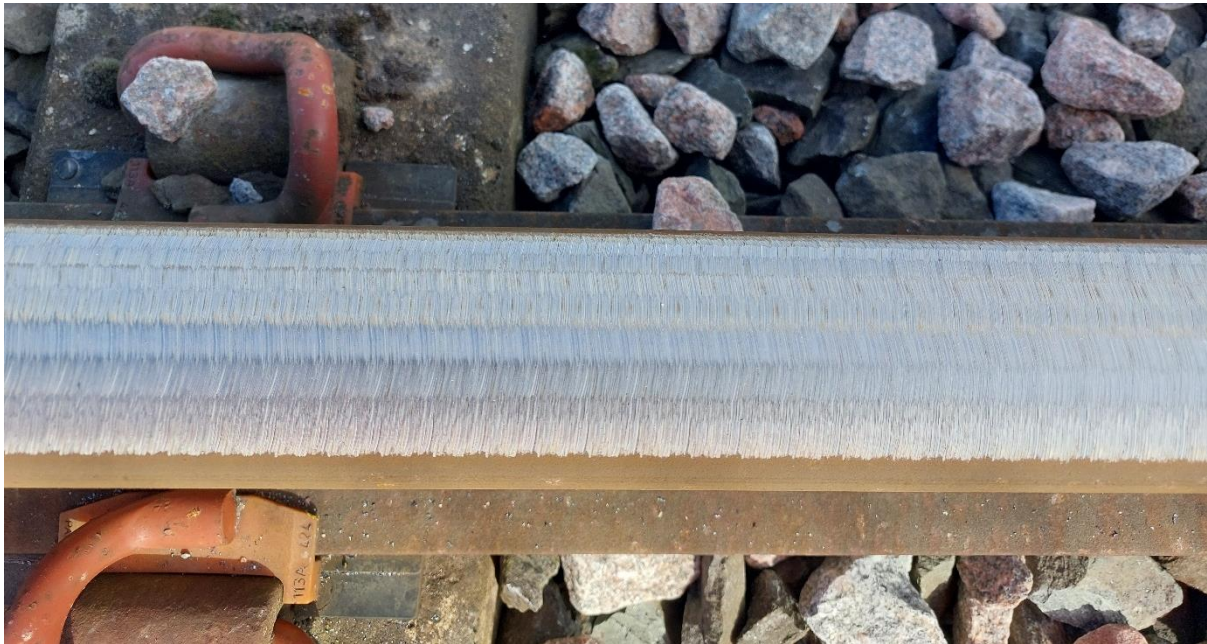
Figure 48: The post-grind condition of a section of the rail which was ground during the Grinding Campaign at Drax Power station.
