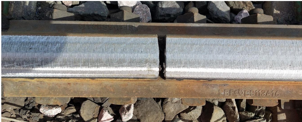
Figure 5: Post-grind conditions of two sections of rail
