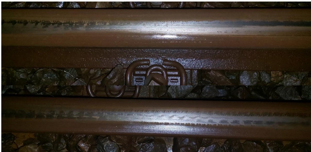
Figure 38: Initial rail surface conditions of rail prior to grinding operation on the Metro dé Medellín tracks.
