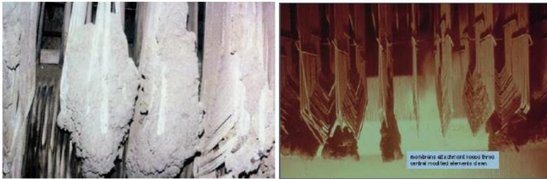
Figure 1-2: Slagging formation on a pulverised fuel boiler [25].
