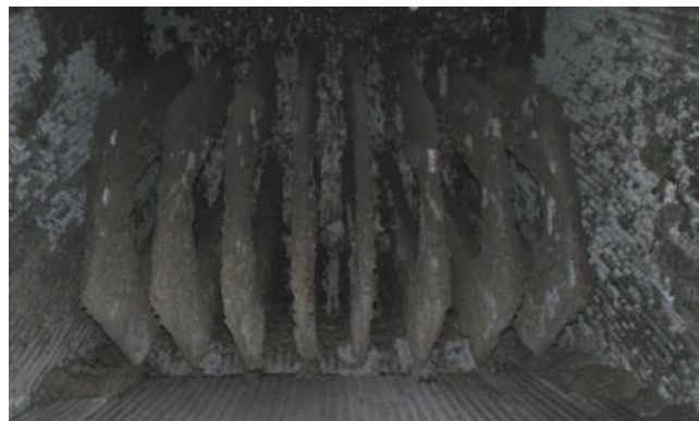
Figure 1-4: Ash deposits on superheater in top furnace during straw firing at Masnedø CHP plant [41].
