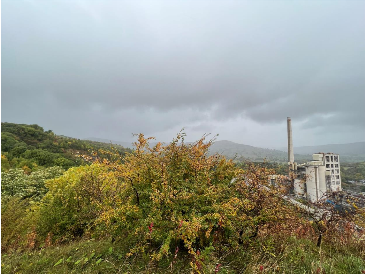
Figure 5-9: Cement Plant building and the former area of mineral extraction now reinstated with a vegetation of mature small trees and shrubs. Example for the renaturalisation of the quarry area as envisaged for the remainder of the extraction areas. Source: photo by M. Tenzer.
