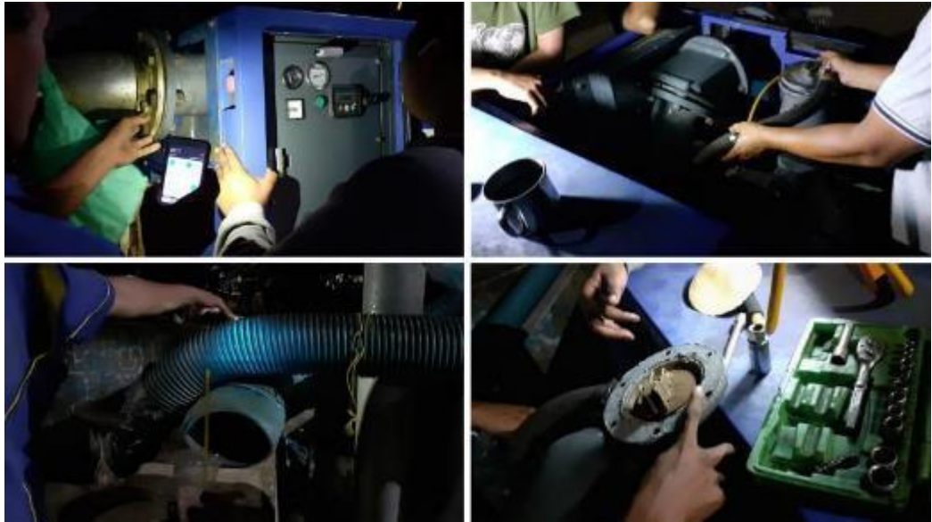
Figure 193 Repairing water pump during the night, by author, 2021/02/26..
