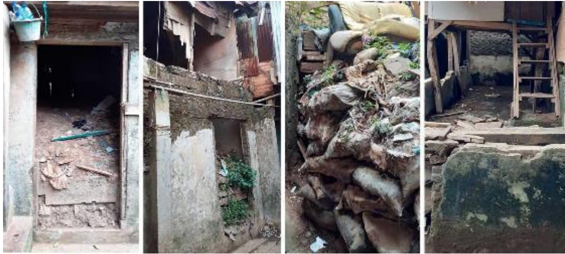
Figure 168 Mud sediments from the floods accumulated in the landscaping of the 'ground' of the abandoned houses, by author, fieldwork in Jakarta, on 2021/07/17.
