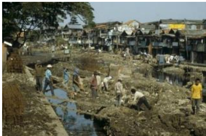
Figure 68 'Kampung Verbetering'/Kampung Improvement in making drainage and dredging occupied riverbanks, 1993, public domain, Tropenmuseum Collection.
