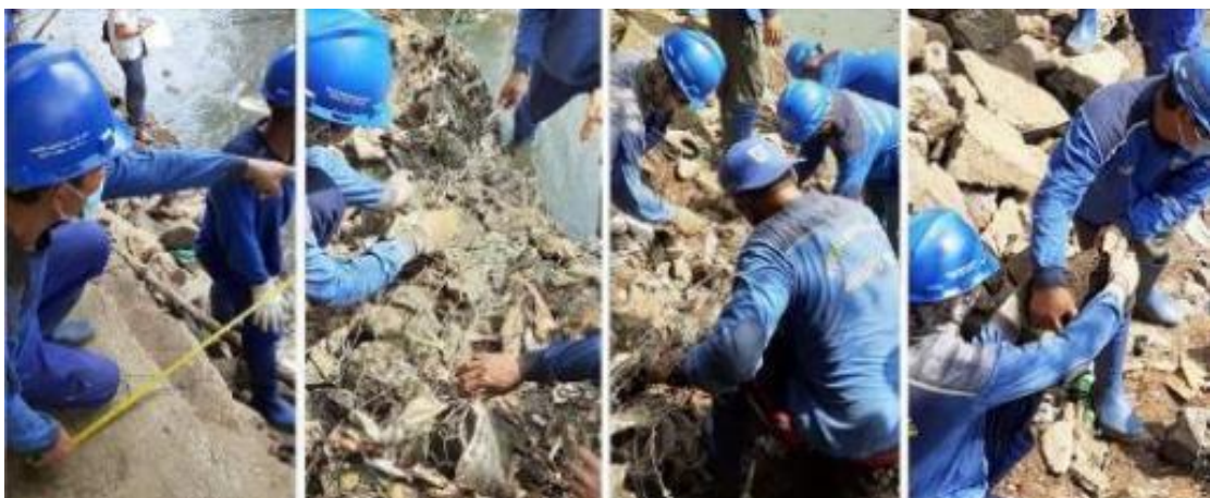
Figure 189 Repairing 'temporary repair' of eroding riverbank in Kali Cipinang, by author, 2021/03/03.
