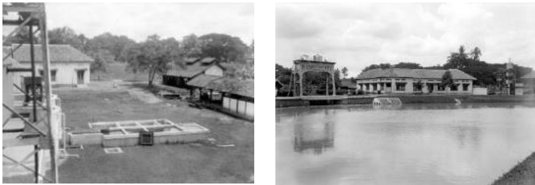
Figure 66 Infrastructure for water supply showing slow filter installation and water purification in Manggarai, date unknown, public domain, Tropenmuseum Collection.
