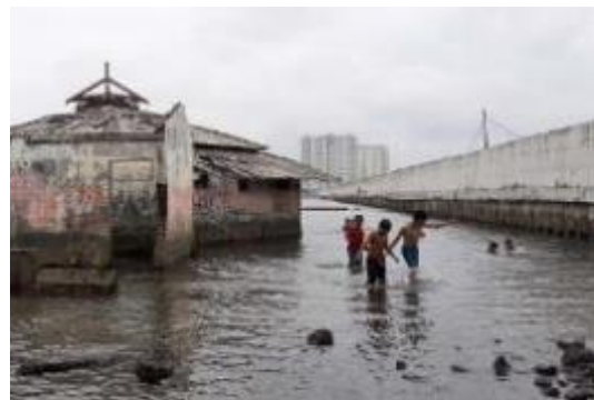
Figure 230 Children swam on the waterfront of seawall in Muara Baru, by author, fieldwork 2021.
