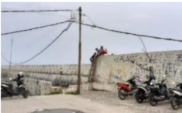
Figure 229 Children climbed the sea wall in Muara Baru, by author, fieldwork 2021.
