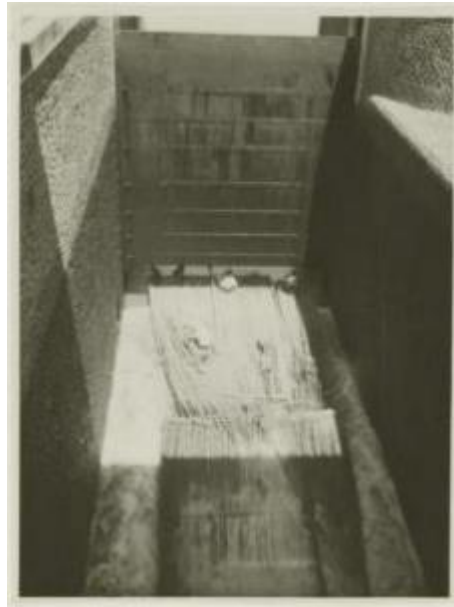
Figure 60 Bamboo raft passes through the opening floodgates in the sluice of Karawang Weir, 1931, public domain, KITLV.
