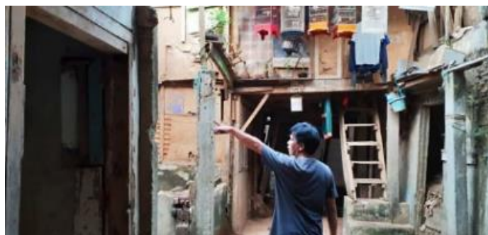
Figure 202 Agus, Dea's assistant in RW 5, pointed to ruined abandoned houses and occupied rental rooms at the upper ground level, by author, 2021/07/23.
