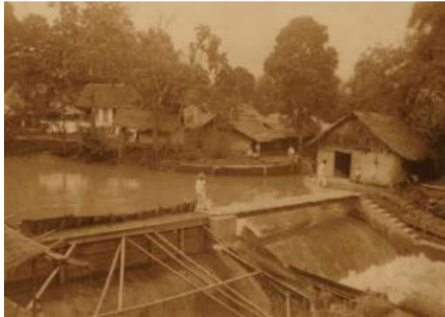
Figure 61 Dam in the river behind Beri-Beri Hospital di Buitenzorg, the upper part of Katulampa Dam, 1897, public domain, KITLV.
