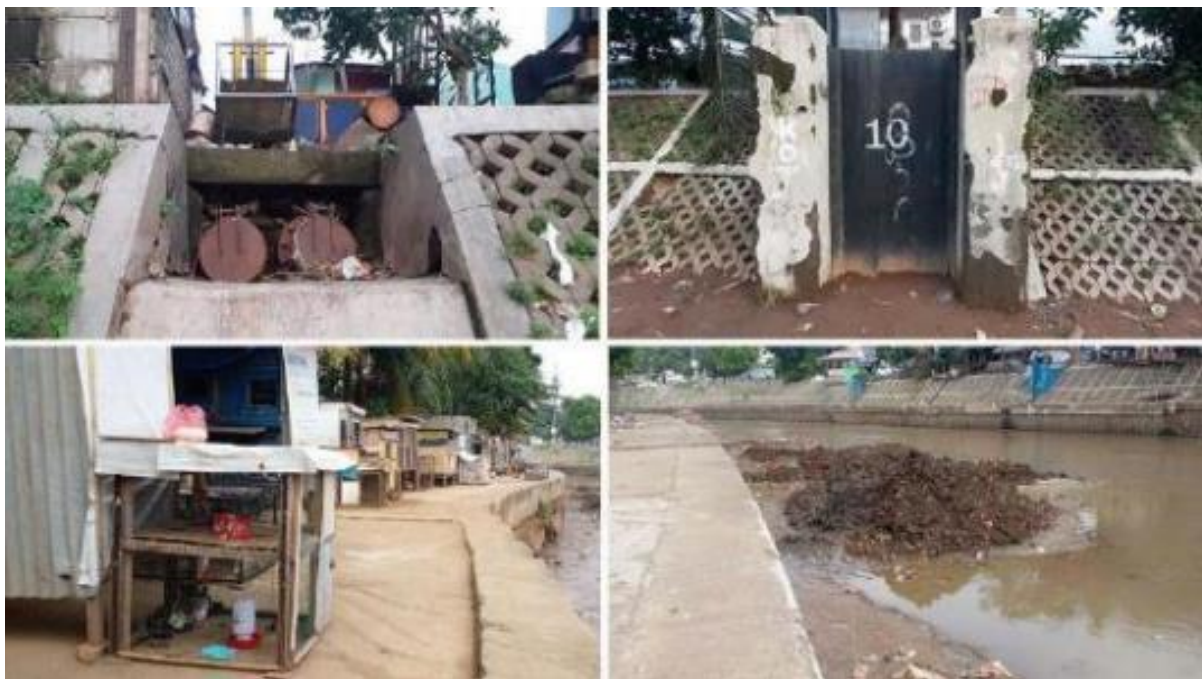
Figure 149 Abandoned floodgate, occupation of embankment, and piled sediments, by author, fieldwork on 2021/08/04
