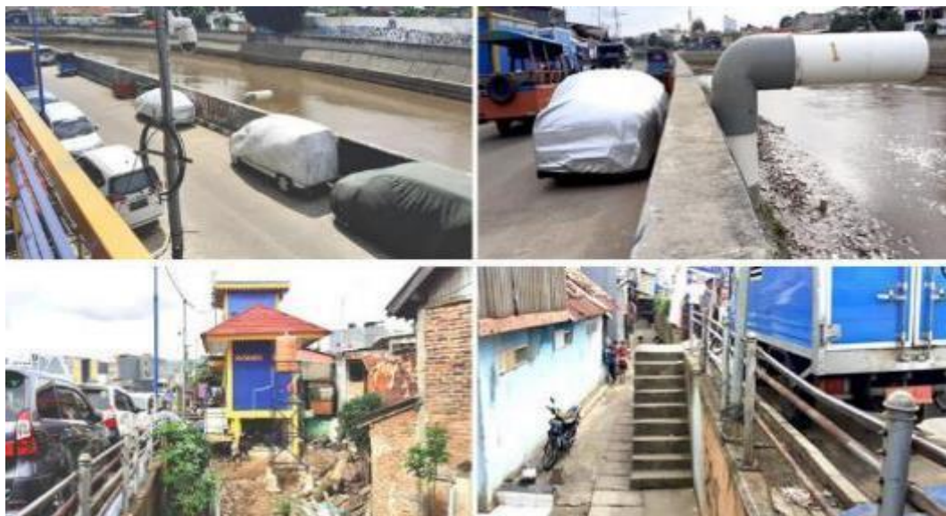
Figure 192 The emplacement of road embankment, water pipes, flood monitoring station, and diesel generators set the elevation of dry land to step from the low-lying riverine settlement, by author, 2021/02/21.
