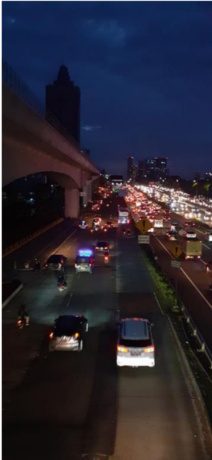
Figure 234 Starting the night time shows the flows of traffic on the main roadway and toll road with emplacement of the elevated Light Rapid Transit (LRT) in Cawang Ciliwung, covering the river beneath them (Photo by author, 04/01/2021).
