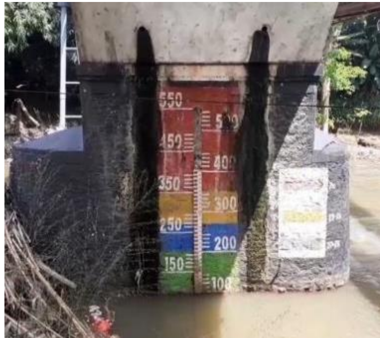
Figure 31 Sunlight fell upon flood marking painted on a concrete-stone pile bridge for daily flood monitoring in Ciliwung on Depok City, by author, fieldwork in Jakarta, March 2021.
