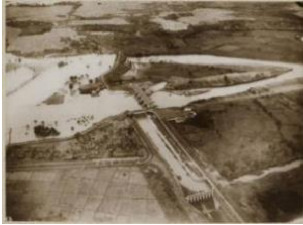
Figure 59 Assemblages of irrigation work and road development in Walahar Weir that serves agricultural settlements in Karawang, 1928, public domain, KITLV.
