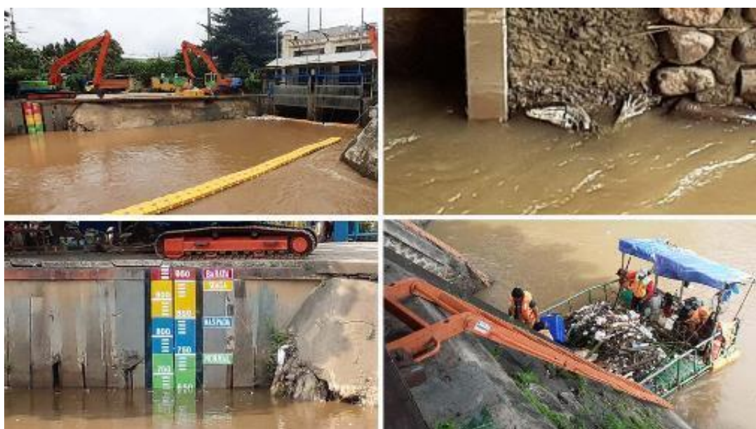
Figure 147 Manggarai Floodgate assembled floodgate, water monitor, waste collection, and hazard indicator, by author, fieldwork in 2021.
