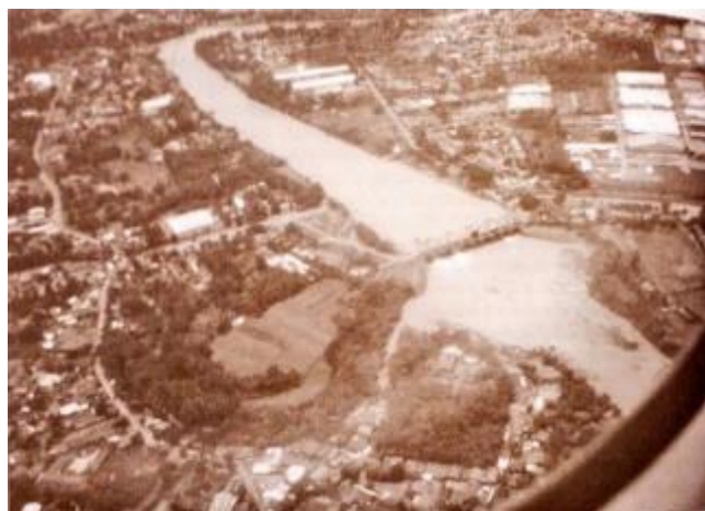
Figure 58 Weir in Cisadane River in Tangerang with urbanising settlements from road development, by Ravesteijn, 2018, used under copyright permission.
