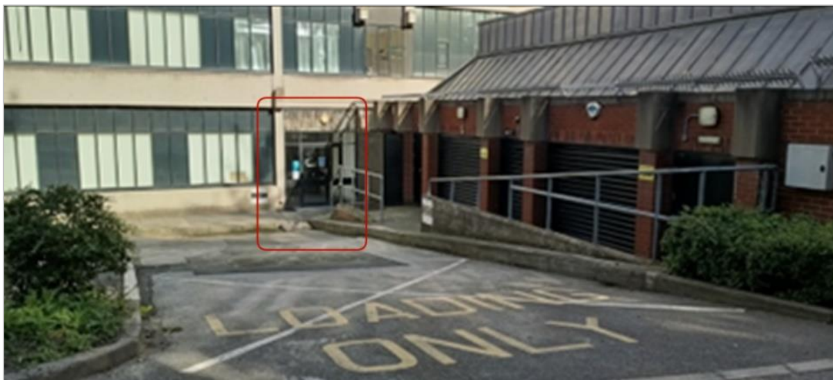
Figure 4.15. Area 6 – An entrance
