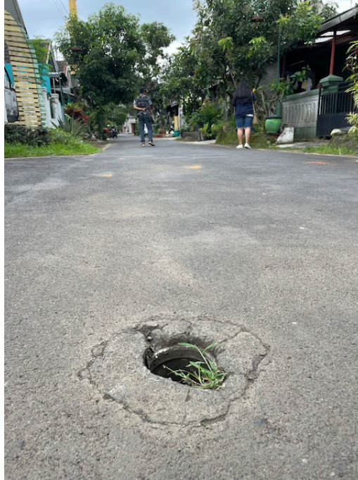
A biopore infiltration hole in the middle of the street of RW 05, Arjowinangun Village, Malang City. Source: Author (taken in December 2021)
