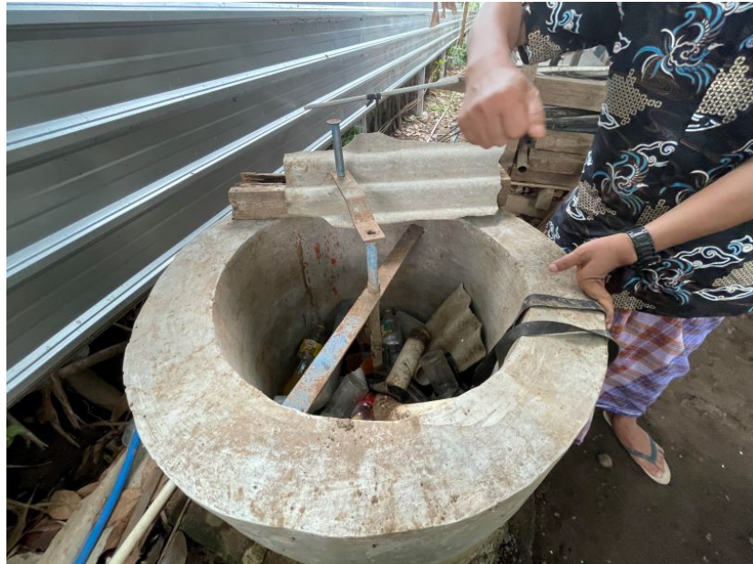
A broken bio-slurry unit due to earthquake. Source: Author
