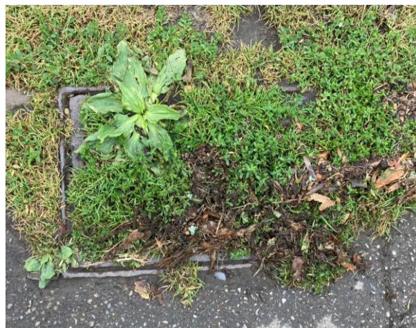
Figure 47. Gully blocked with vegetation at Endcliffe Park in which flood water spills from. Picture taken on 17th August 2022.
