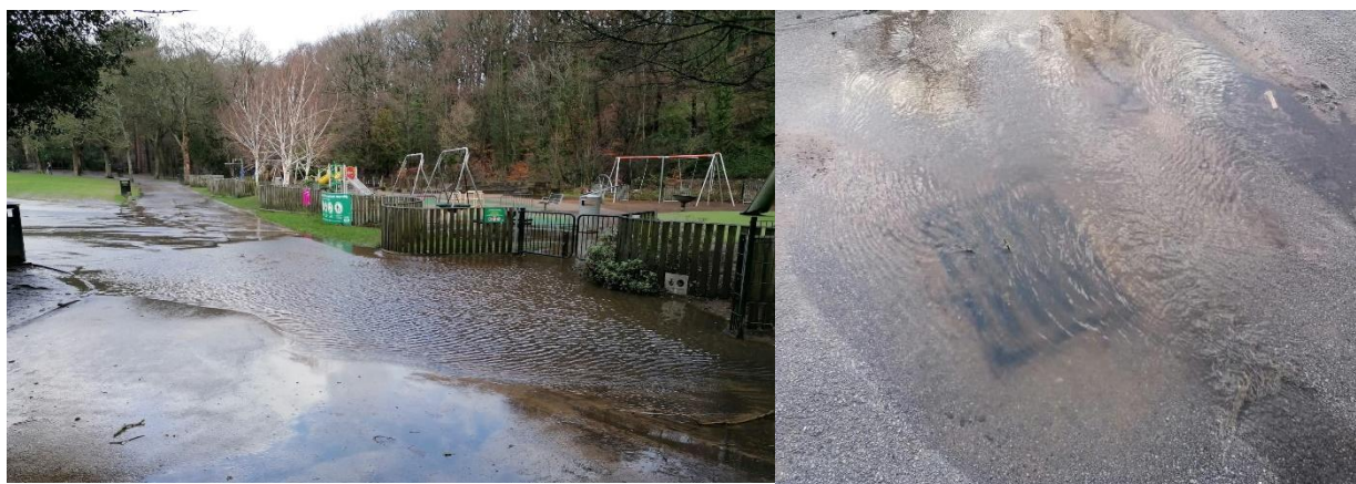
Figure 8. Sampling site at Endcliffe Park, with visibly surcharging gully during a visit after heavy rain in February 2022.
