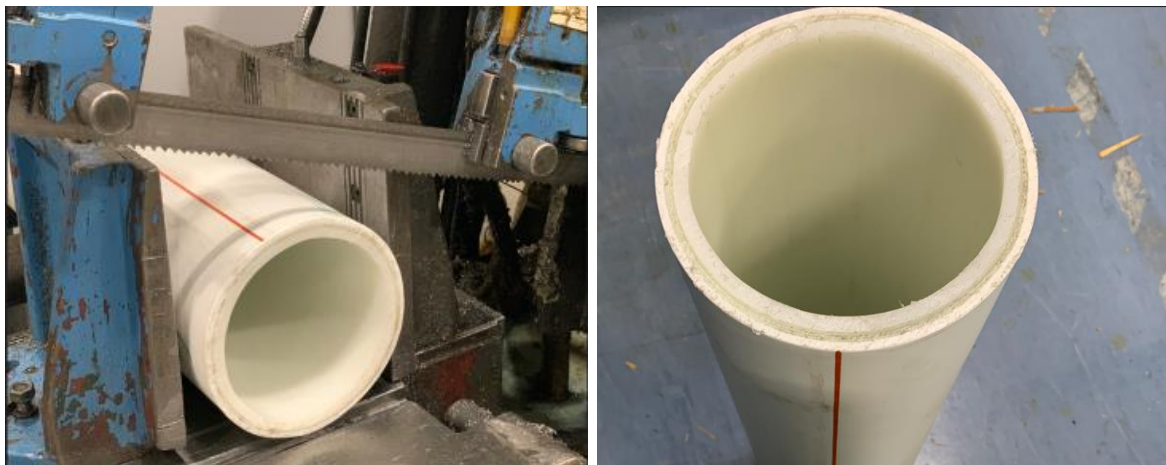
Figure 4-2 Cutting the pipe to square ends
