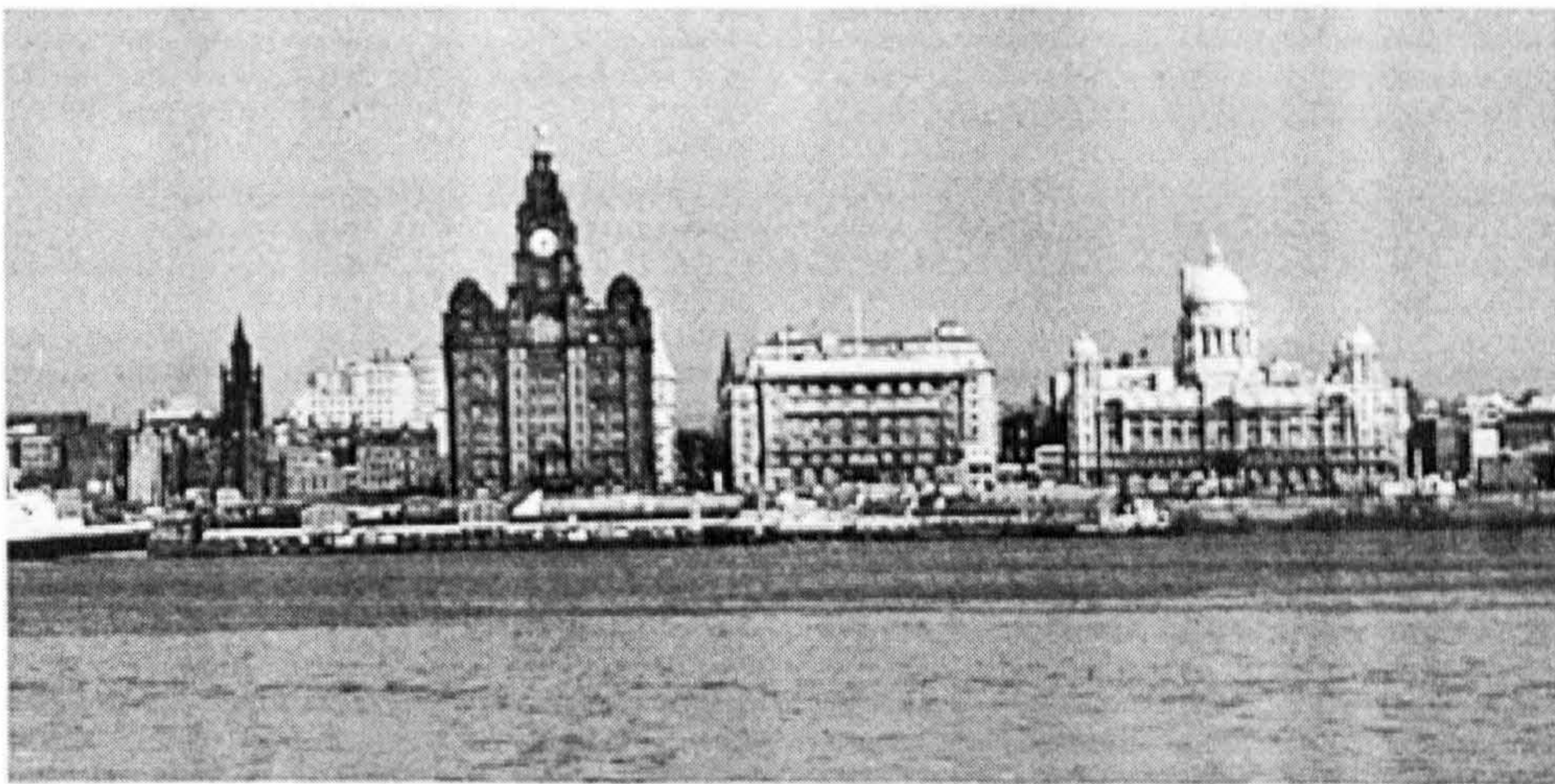
Figure 4.1.27. A view of the Pierhead looking north across the River Mersey.
