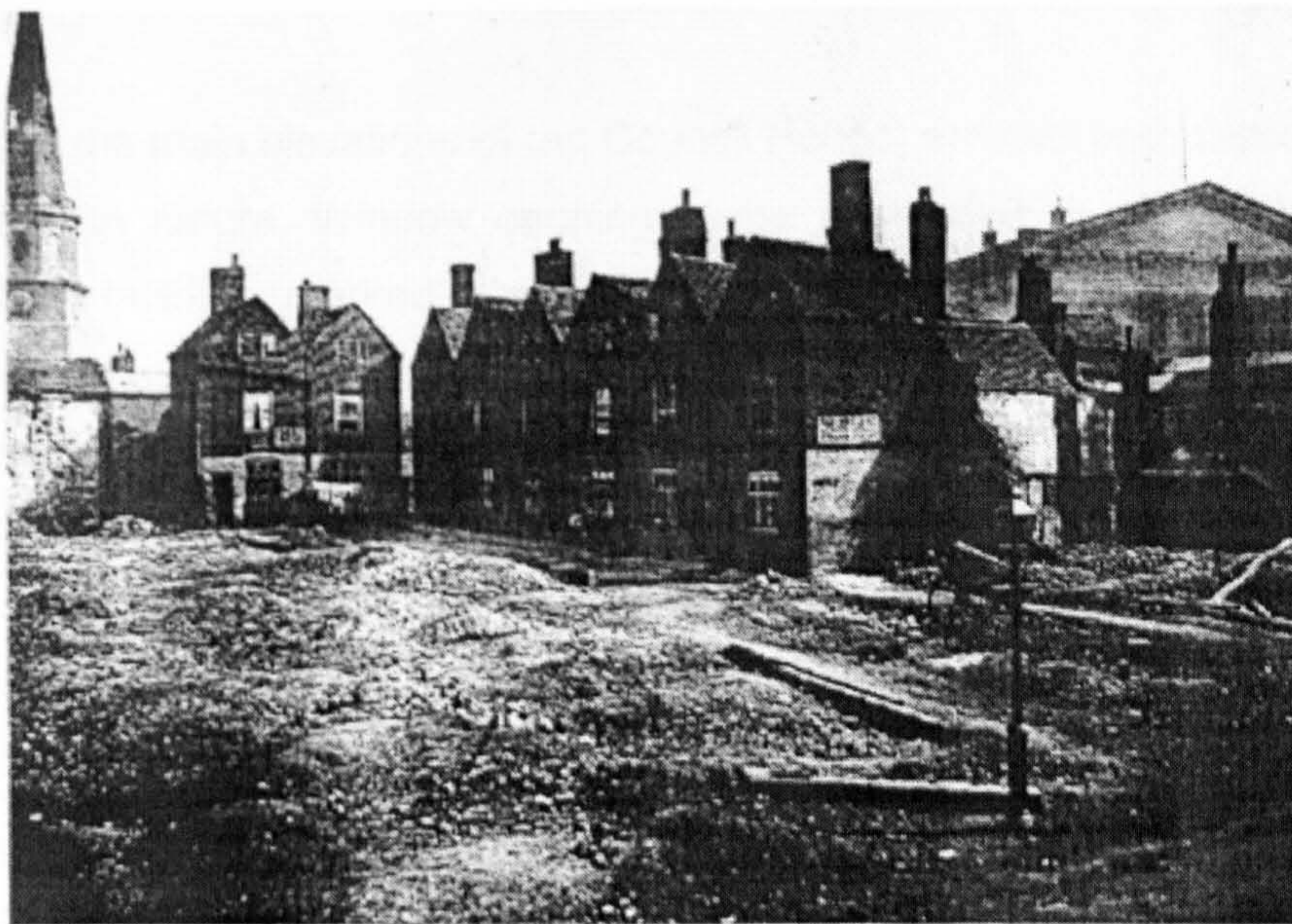
Figure 4.4.7. Buildings being cleared in about 1870 to make way for the new Council House. To the right of the photograph is the Town Hall.
