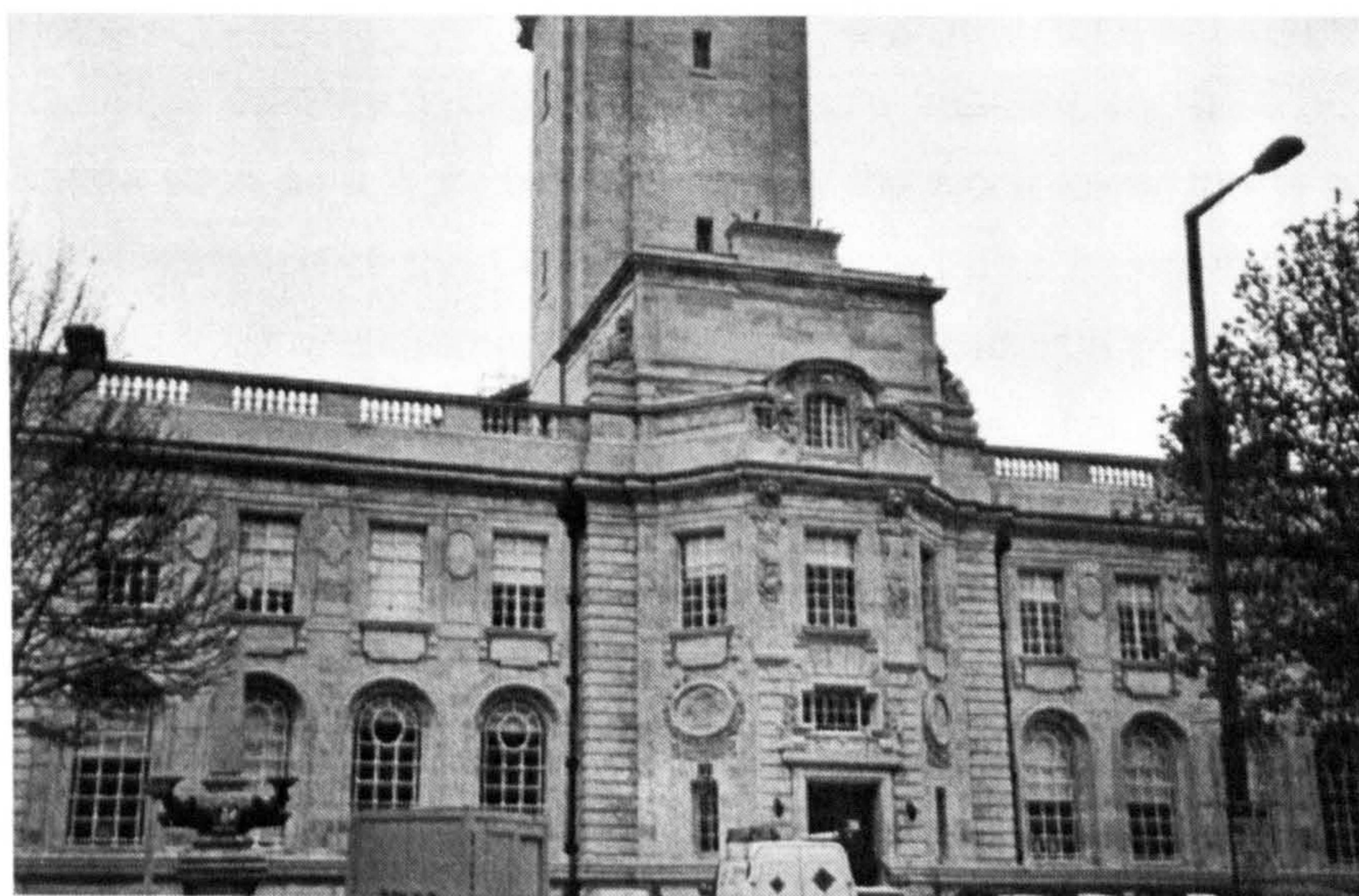
Figure 6.2.8. The side entrance of the City Hall. This entrance faces the Law Courts entrance across King Edward VII Avenue.
