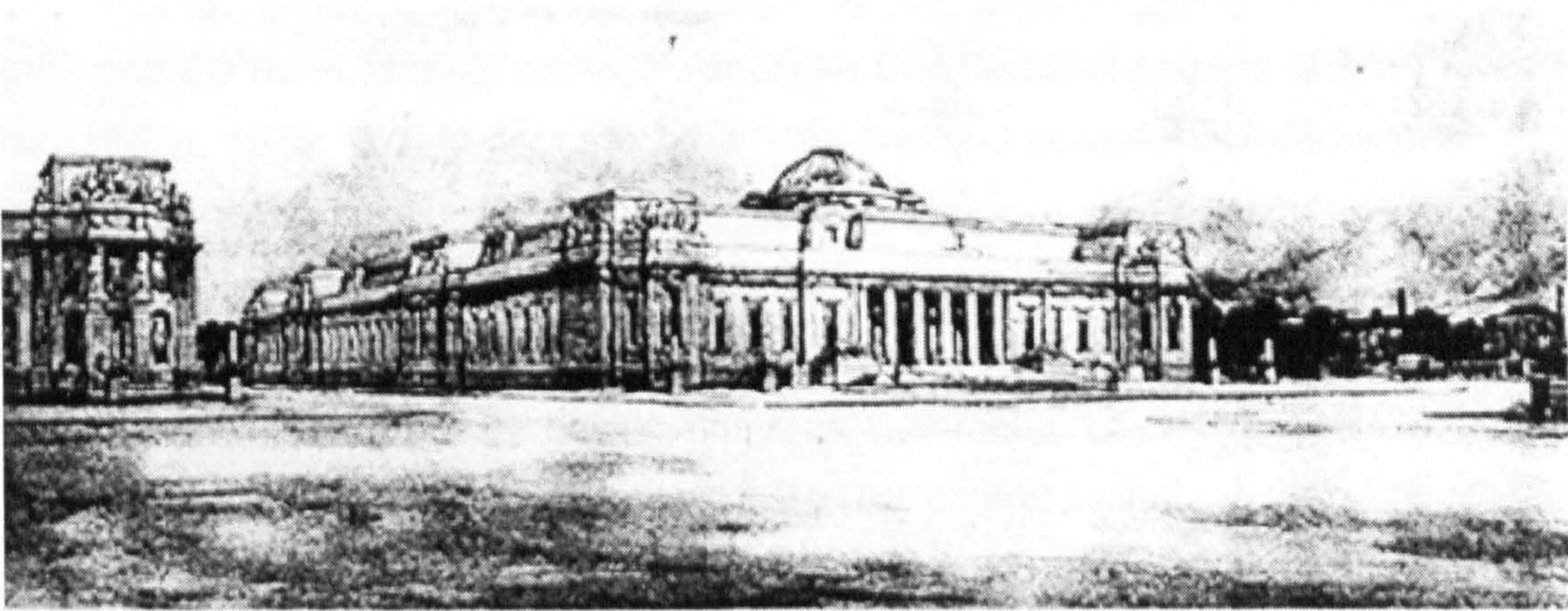
Figure 6.2.15. The National Museum of Wales (source: The Builder , 1910).
