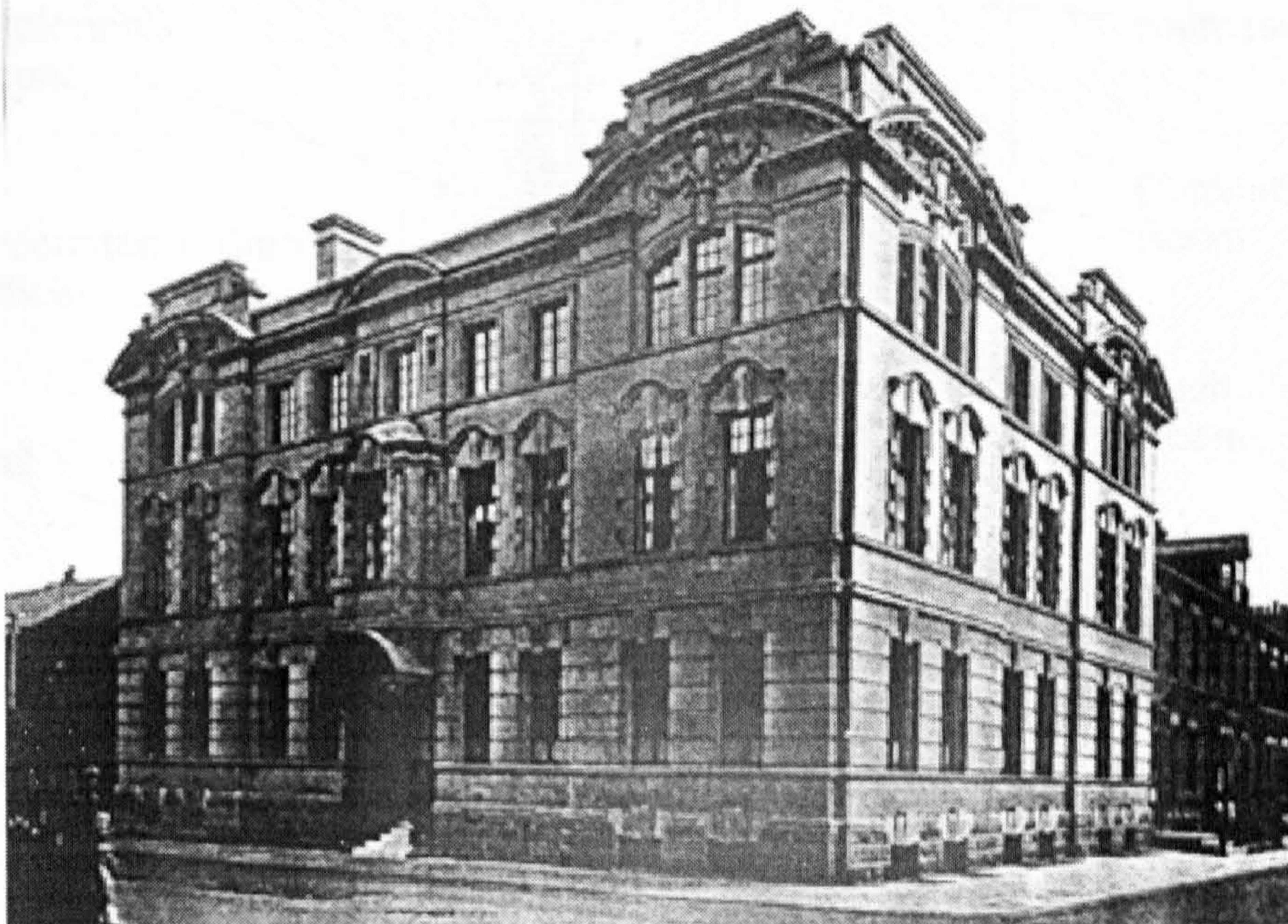
Figure 6.5.13. The front elevation of the River Wear Commissioners Office.
