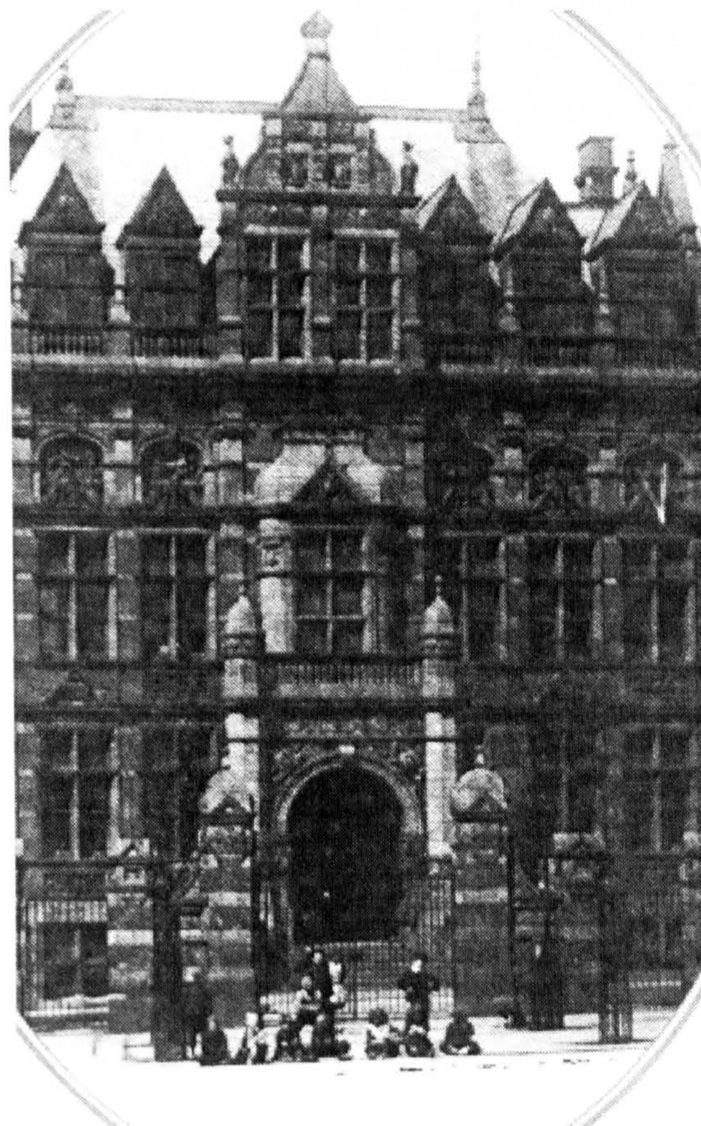
Figure 6.7.9. The main entrance of the Technical College in 1895 (source: De Gex, 1996).
