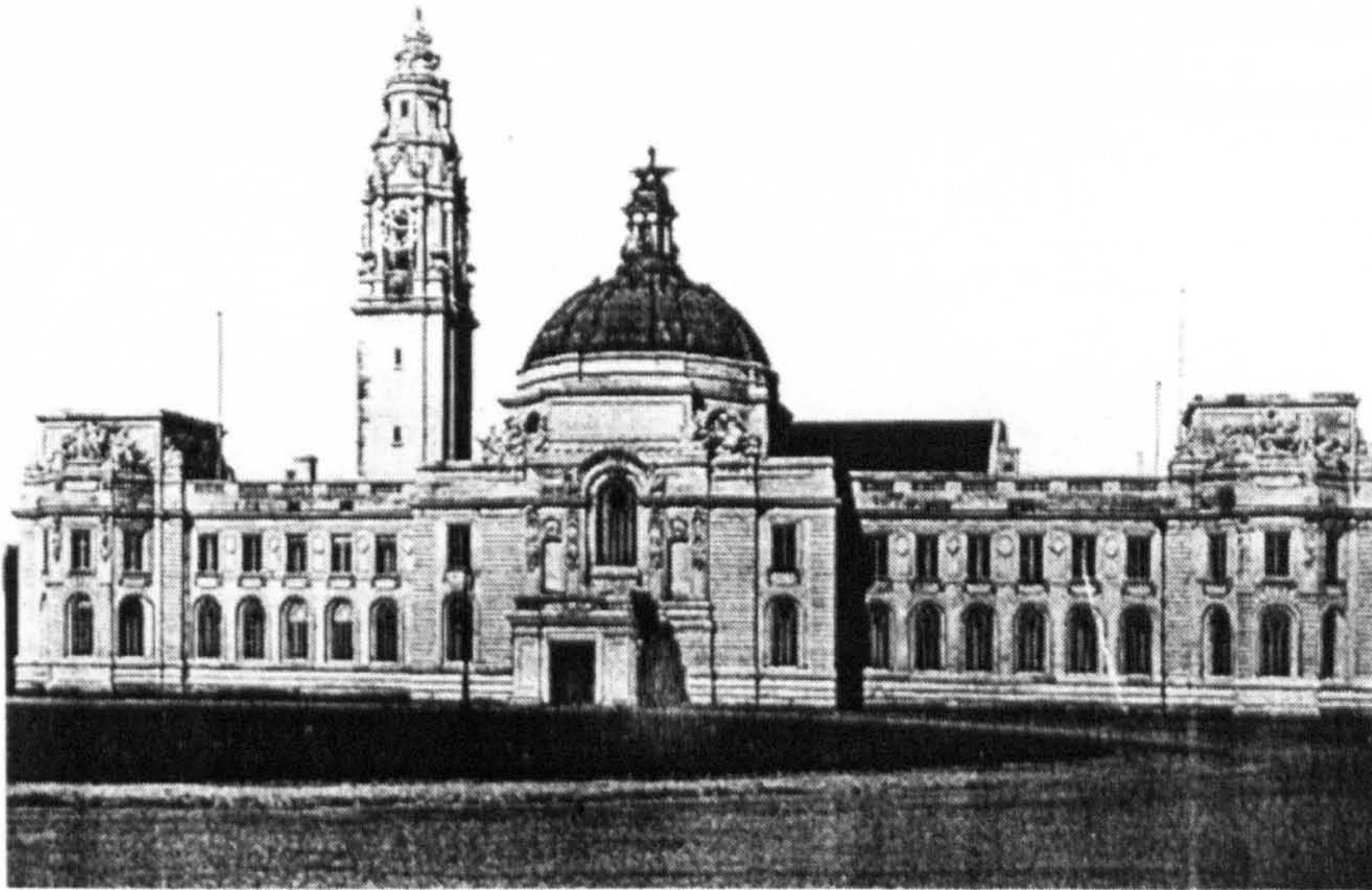
Figure 6.2.4. The main elevation of the City Hall.
