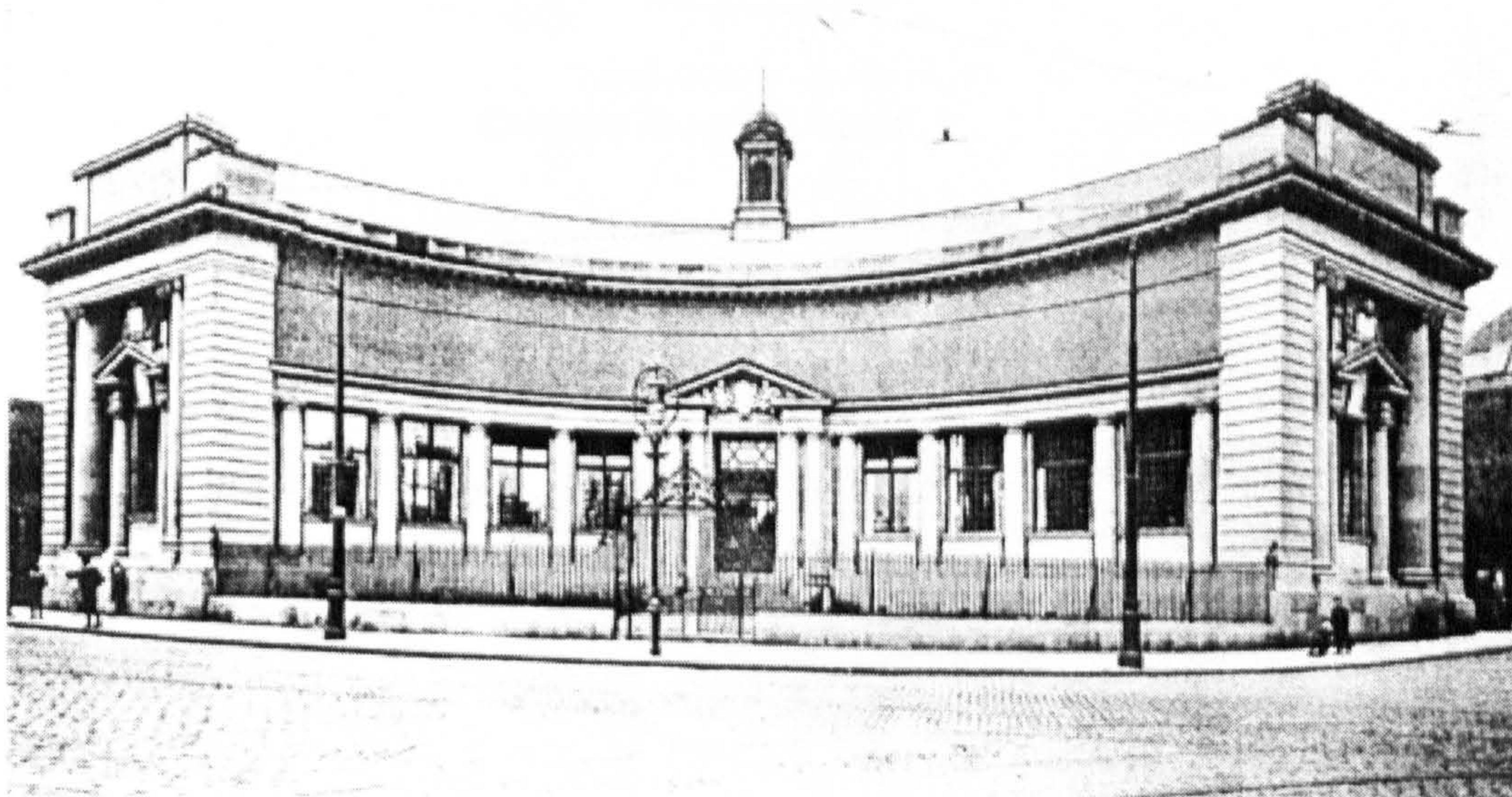
Figure 6.3.16. The Coldside Library.
