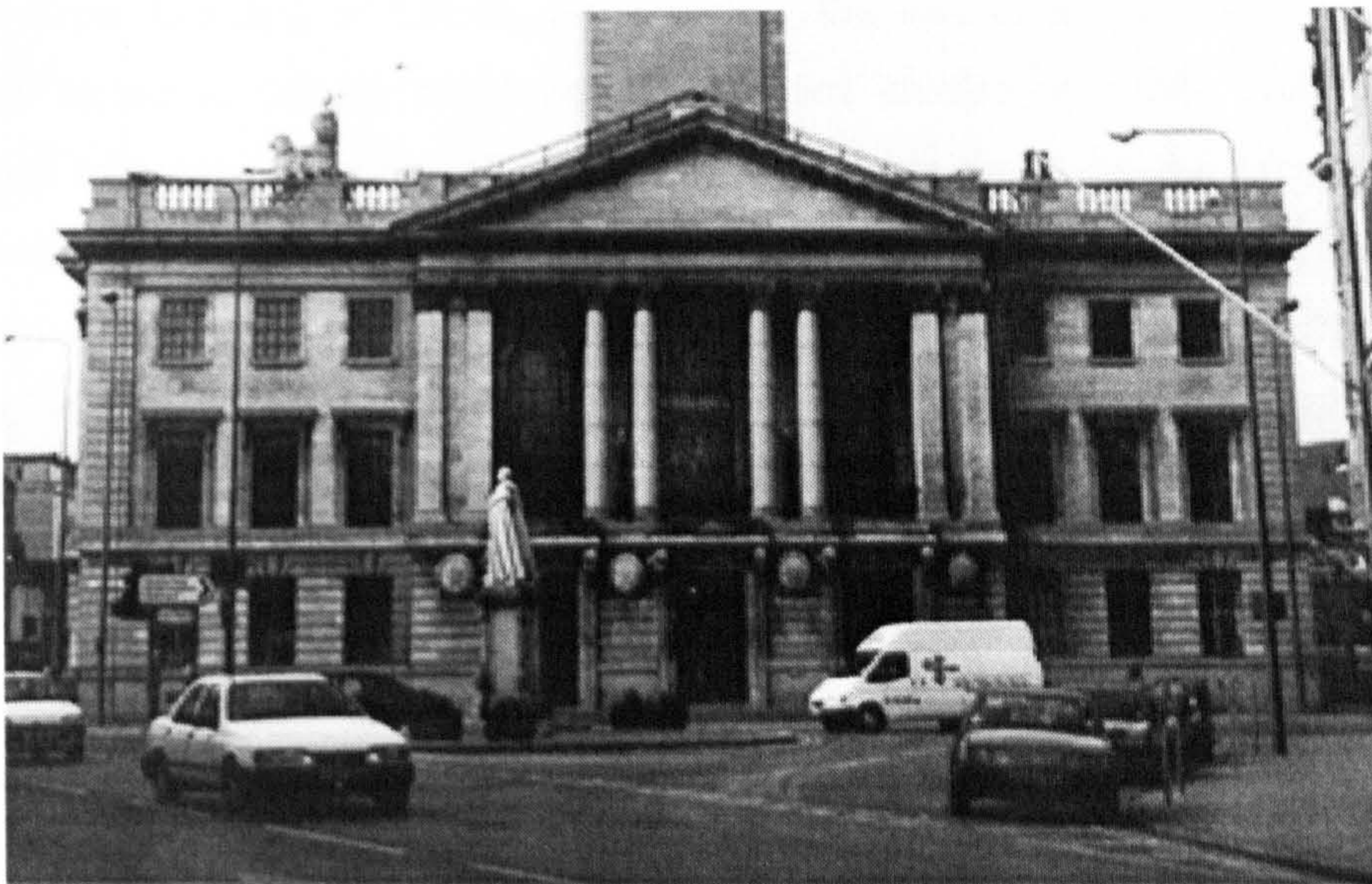
Figure 8.8. The principal elevation of the Guildhall, Hull showing the use of rustication.
