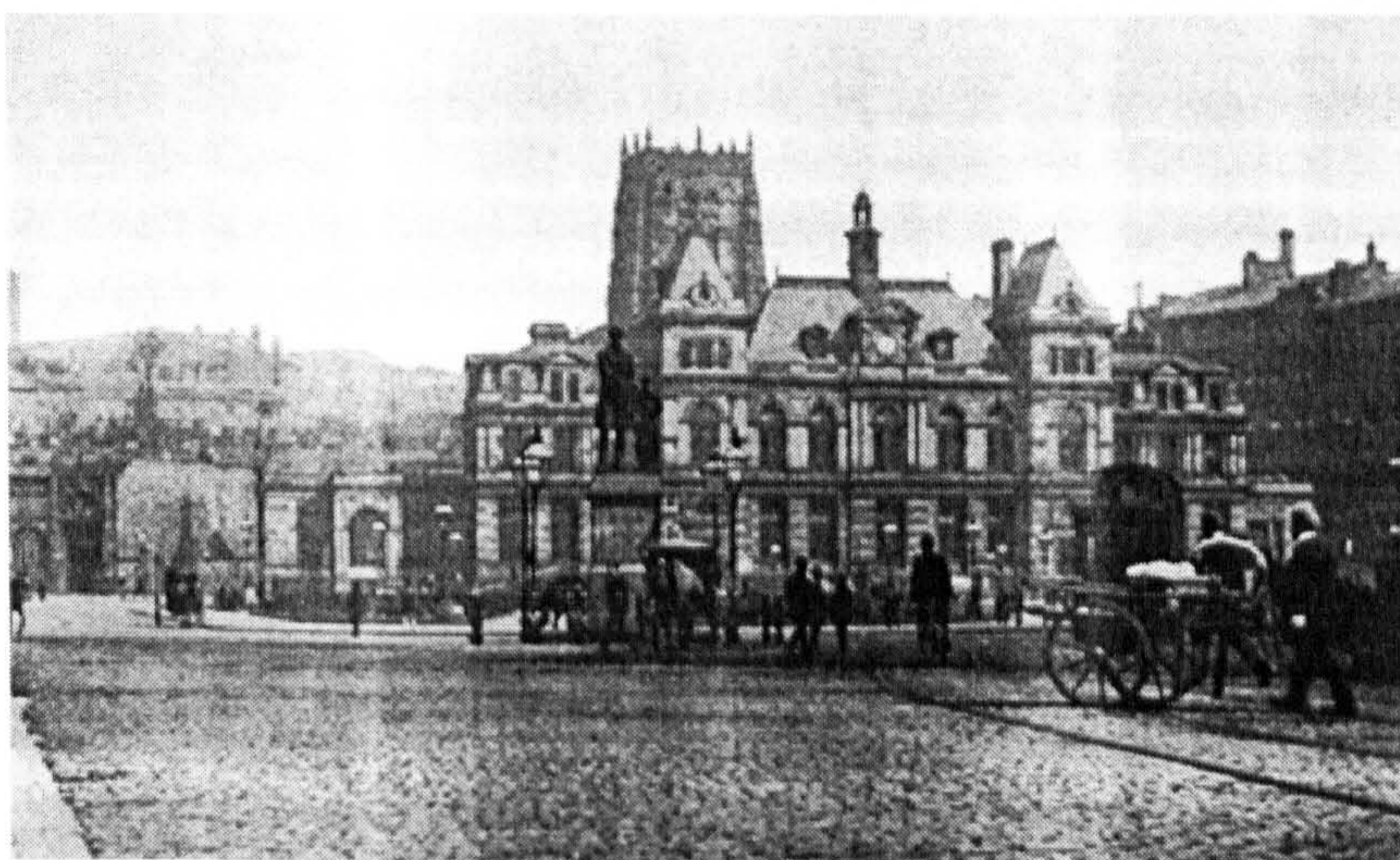
Figure 4.9.11. Eastwards view along Kirkgate in 1895 towards Forster Square.
