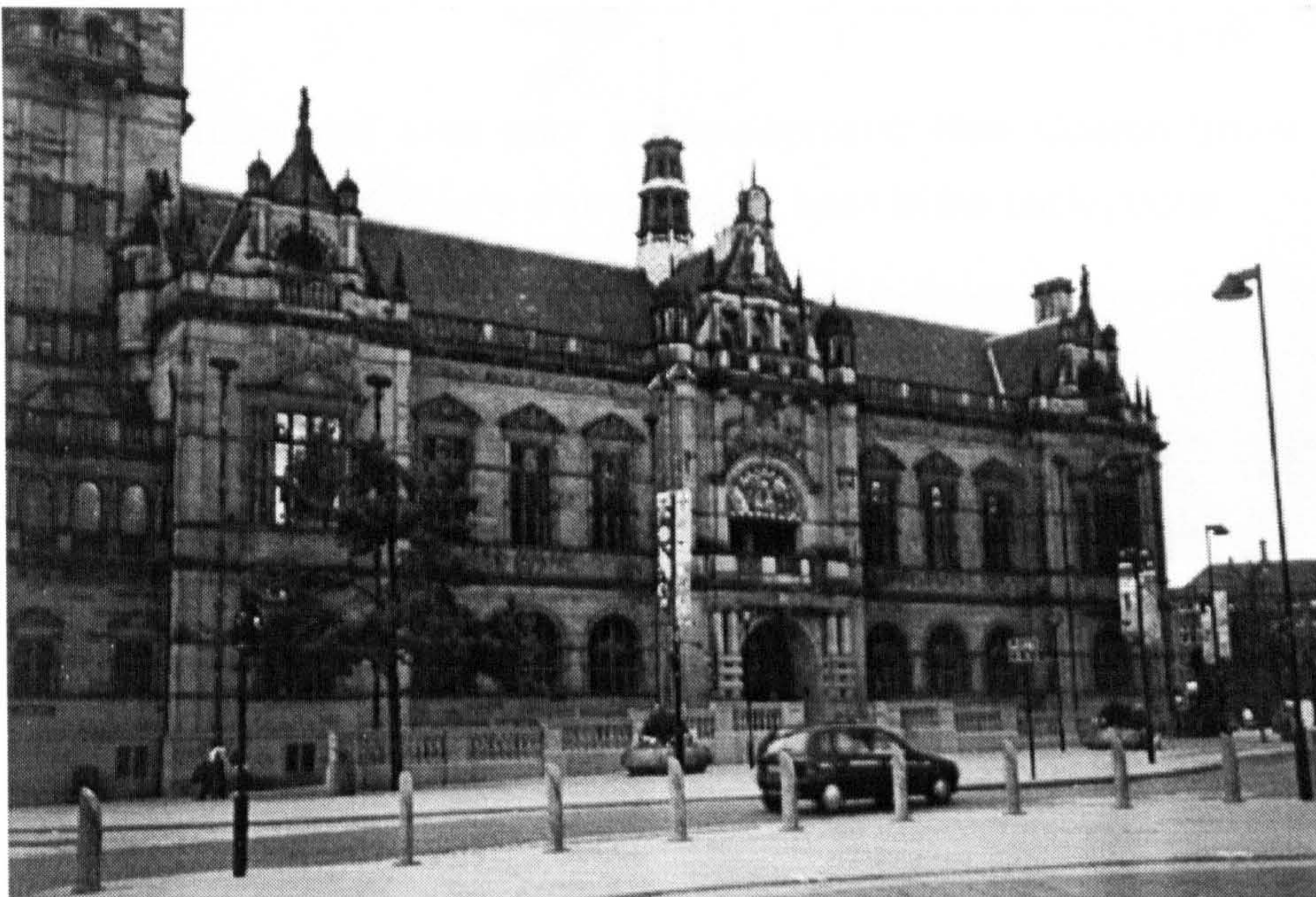
Figure 4.6.4. The Town Hall's front elevation as seen from Barker's Pool.
