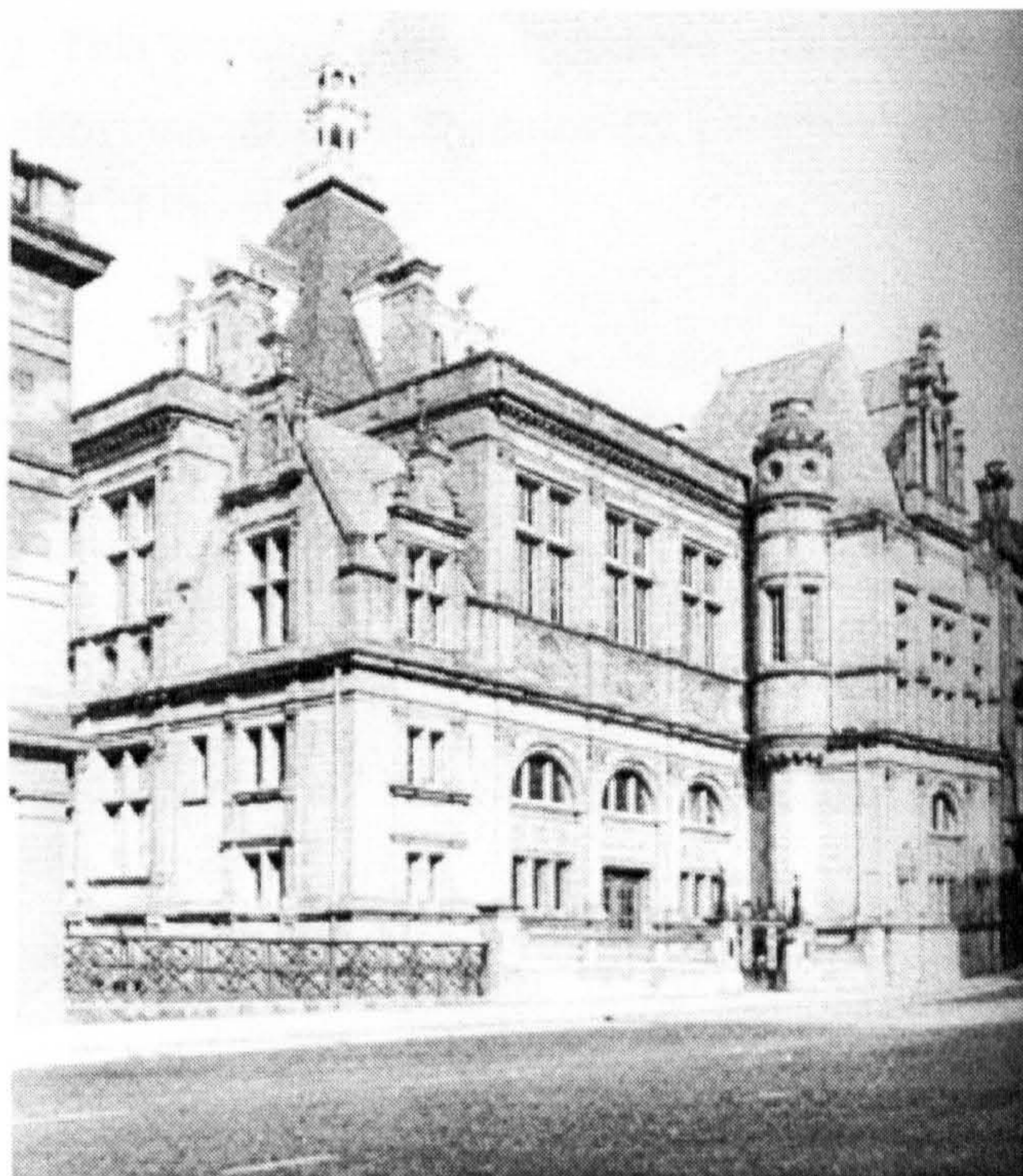
Figure 4.8.8. The Central Public Library building, Edinburgh.
