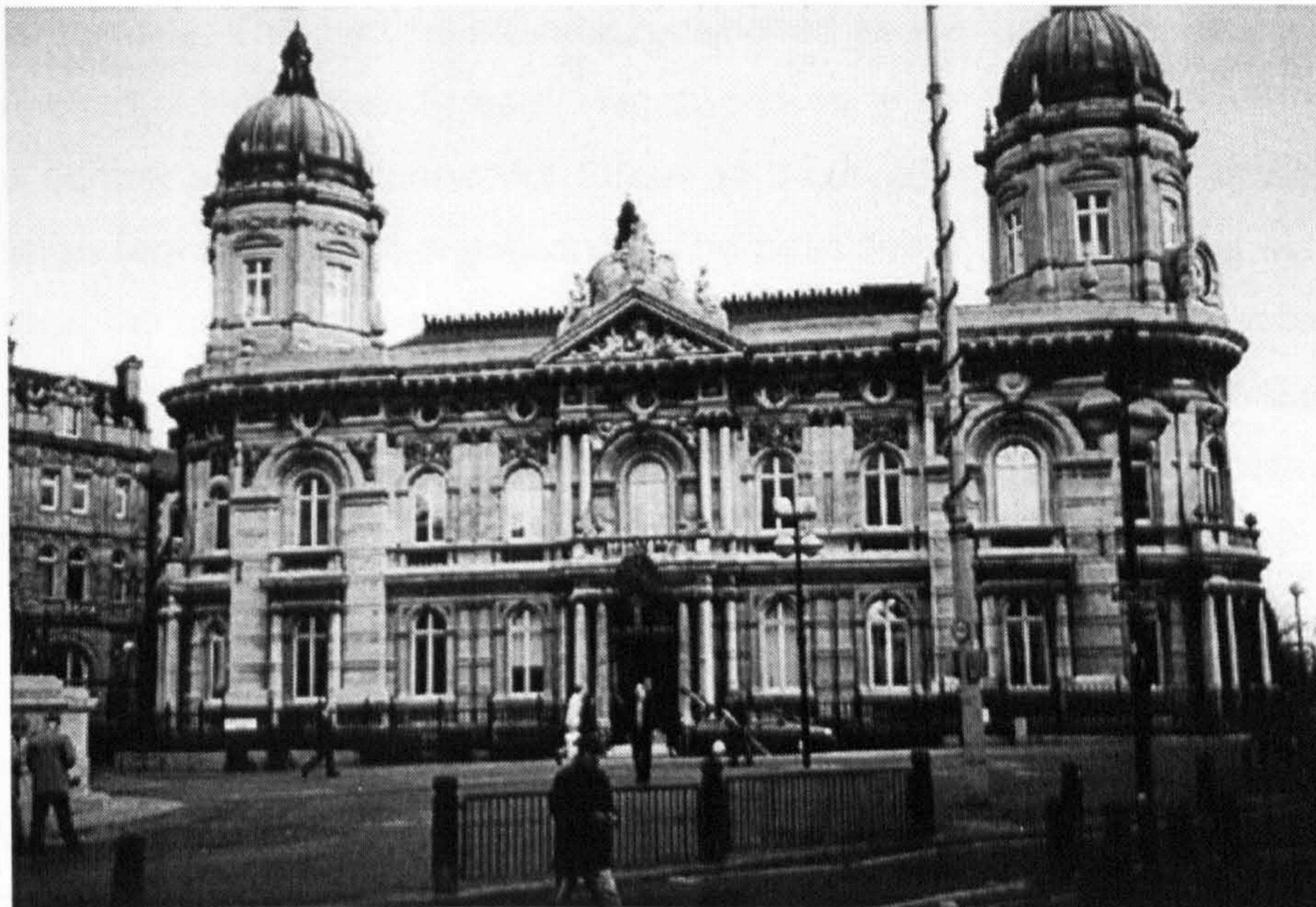
Figure 5.1.1. The front elevation of the Docks Office.
