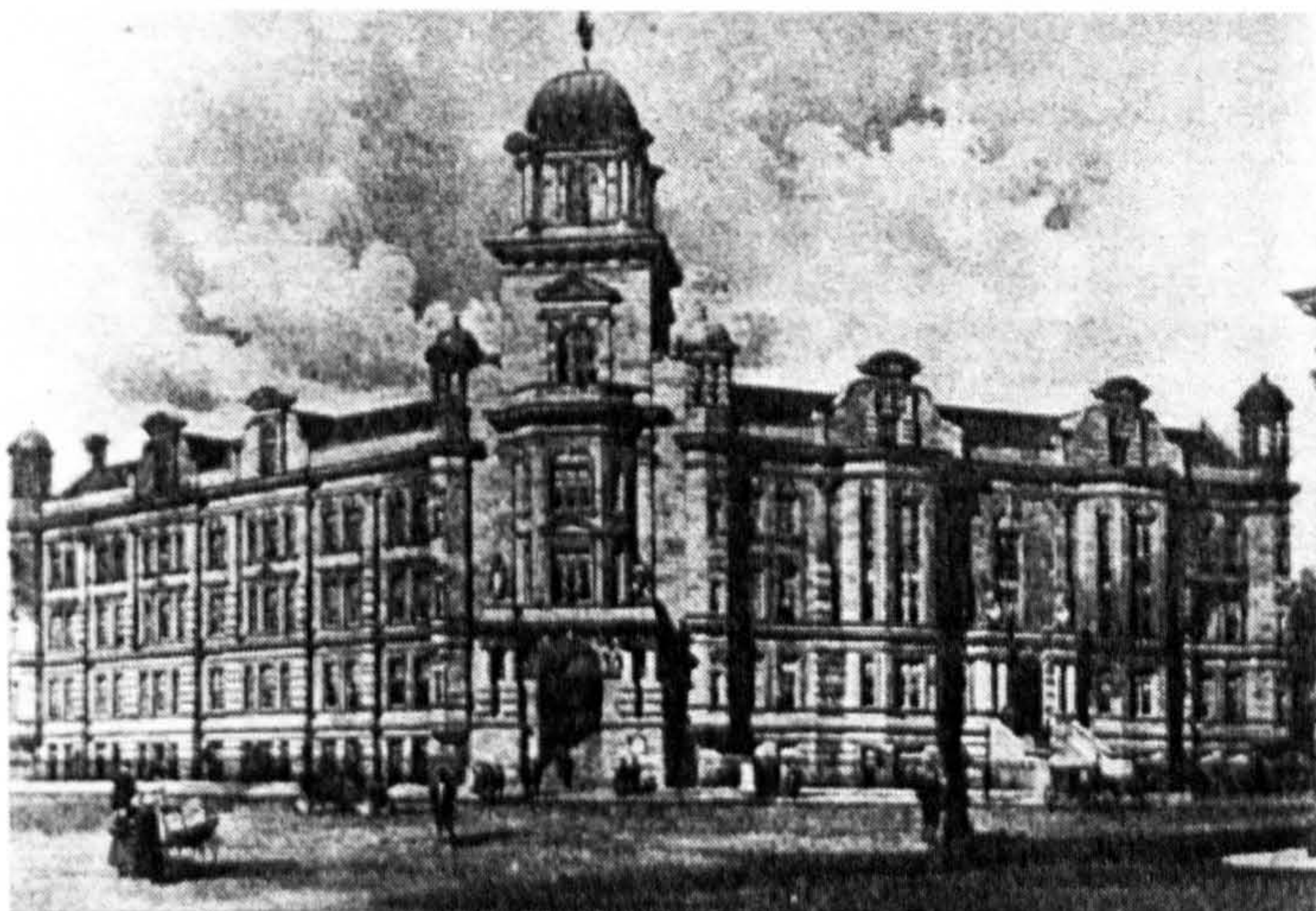
Figure 5.5.6. The front elevation of the Municipal College.
