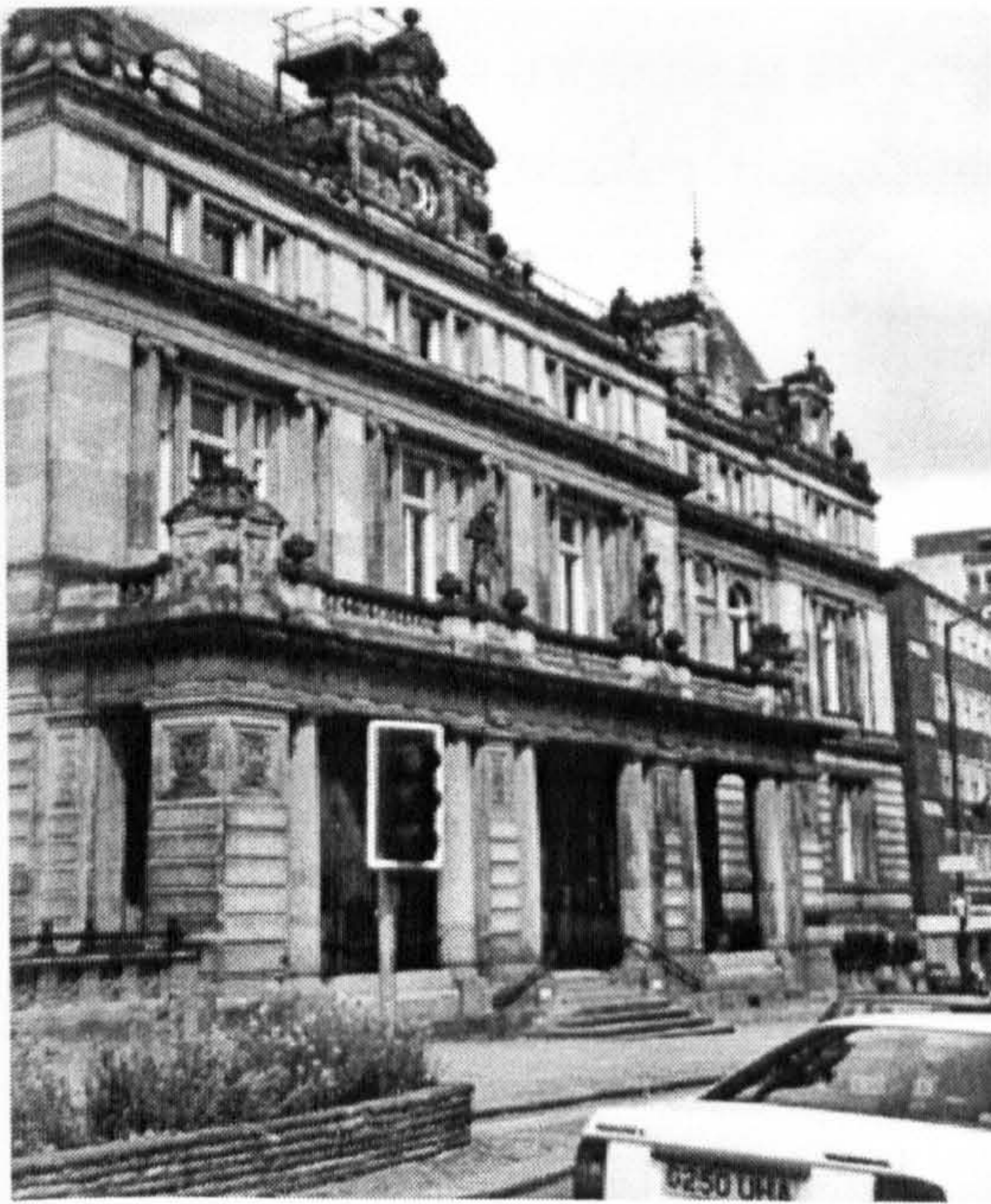
Figure 5.2.12. The central section of the front elevation of the Guildhall.
