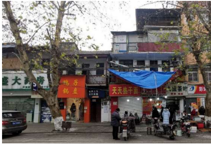
Figure 12 Poor construction and aging buildings
