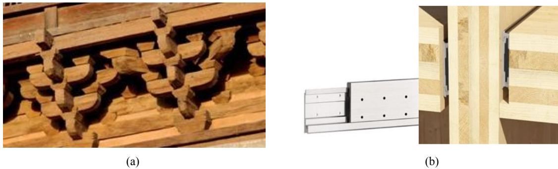
Figure 3.1. Interlocking connection system used in (a) yingxian wooden tower in 1056 AD [3.1] and (b) modern construction (LOCK Connector from Rothoblaas Ltd.)
