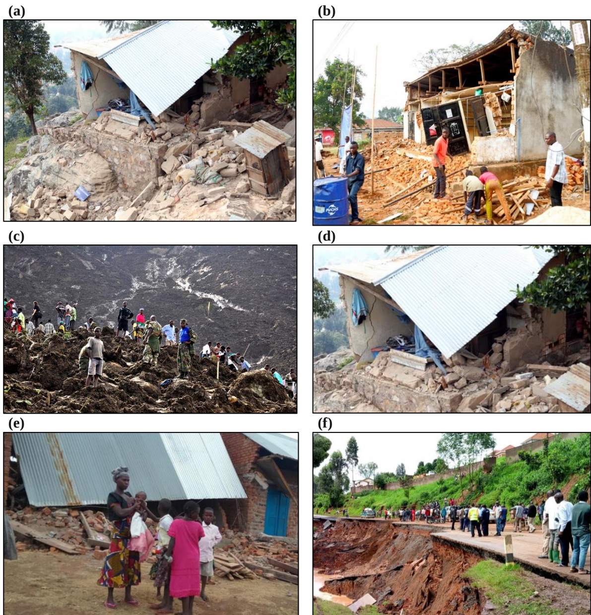
Fig 1.1 Damages to buildings, infrastructure and property across Uganda, due to past earthquake and landslide disasters: (a-b) 1994 Kisomoro earthquake, (c) 2010 Bududa landslide, (d-e) 2016 Bukoba earthquake, and (f) 2023 Kabale-Kisoro road landslide
