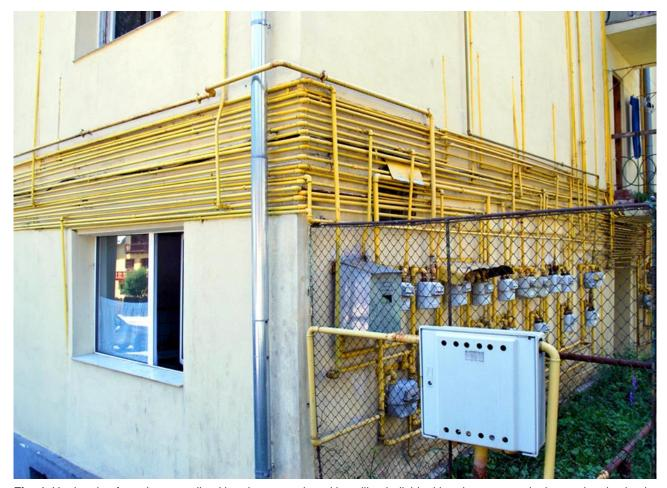
**Fig. 4.** Unplugging from the centralized heating network and installing individual heating systems in the newly privatized apartments from collective housing districts, Sinaia, Romania, 2011. Personal archive of the current author.
