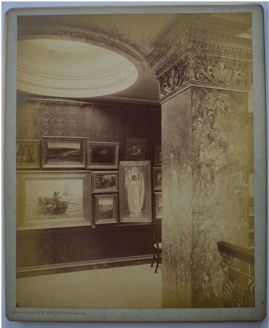
FIGURE 36: BALCONY, NEW GALLERY. SUMMER EXHIBITION, 1888. PHOTOGRAPH.
