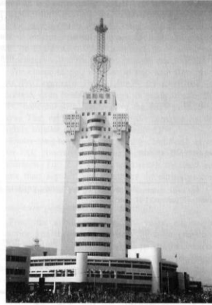
Figure 14: The Shenyang Long Distance Telecommunication Hub, which involved CSA concrete laid in as low as -20 °C, as detailed in Zhang et al. [175].
