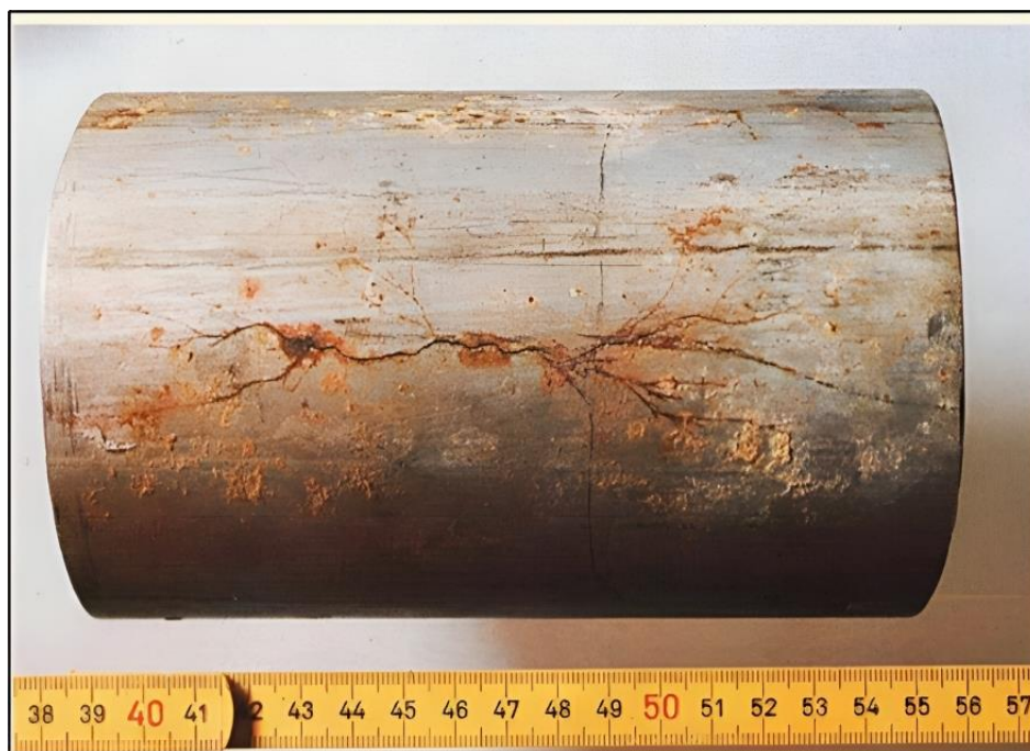
Figure 3-20: An illustration of stress corrosion cracking that took place in type 316 stainless steel that was subjected to thermal insulation in the temperature range of 50 to 60°C. The cracking was initiated by the presence of rinsing water containing 60 mg/kg of chloride, coupled with pre-existing residual stresses [114]
