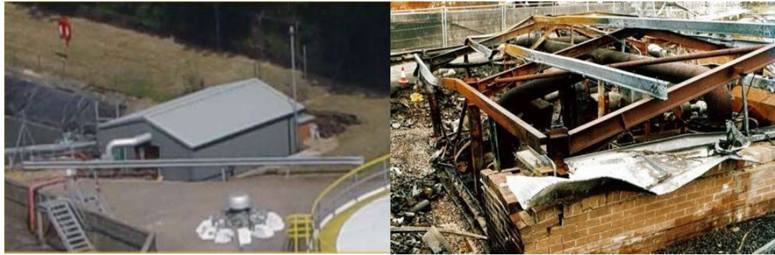
Figure 1 - Buncefield Emergency pump house before and after the explosion [12]
