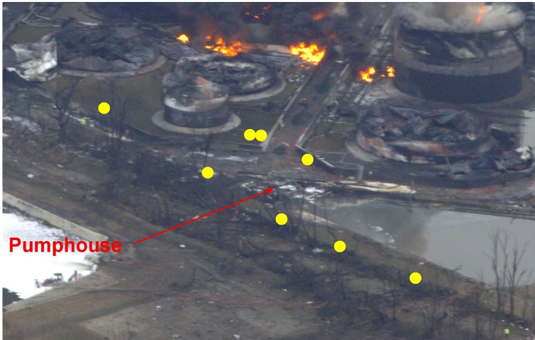
Figure 14 - Final location of cladding panels from the Buncefield pump house [84]
