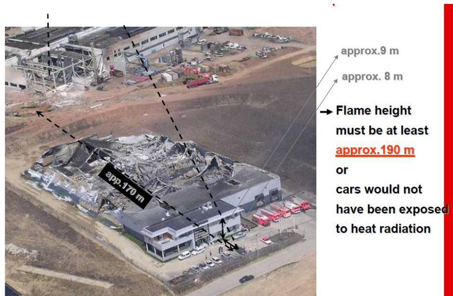
Figure 2-39 Damage to the building located to the west of the pipeline rupture.
