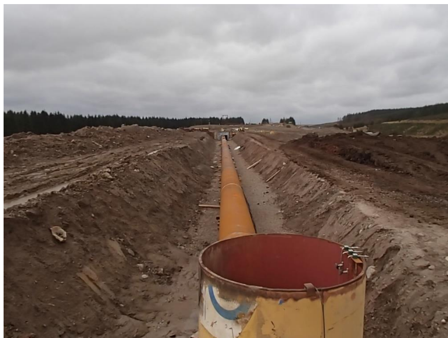
Figure 3-8 Eastern test section before being backfilled
