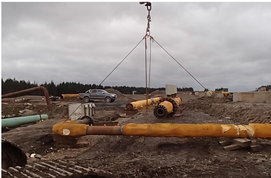
Figure 3-3 Installation of insulated recirculating loop
