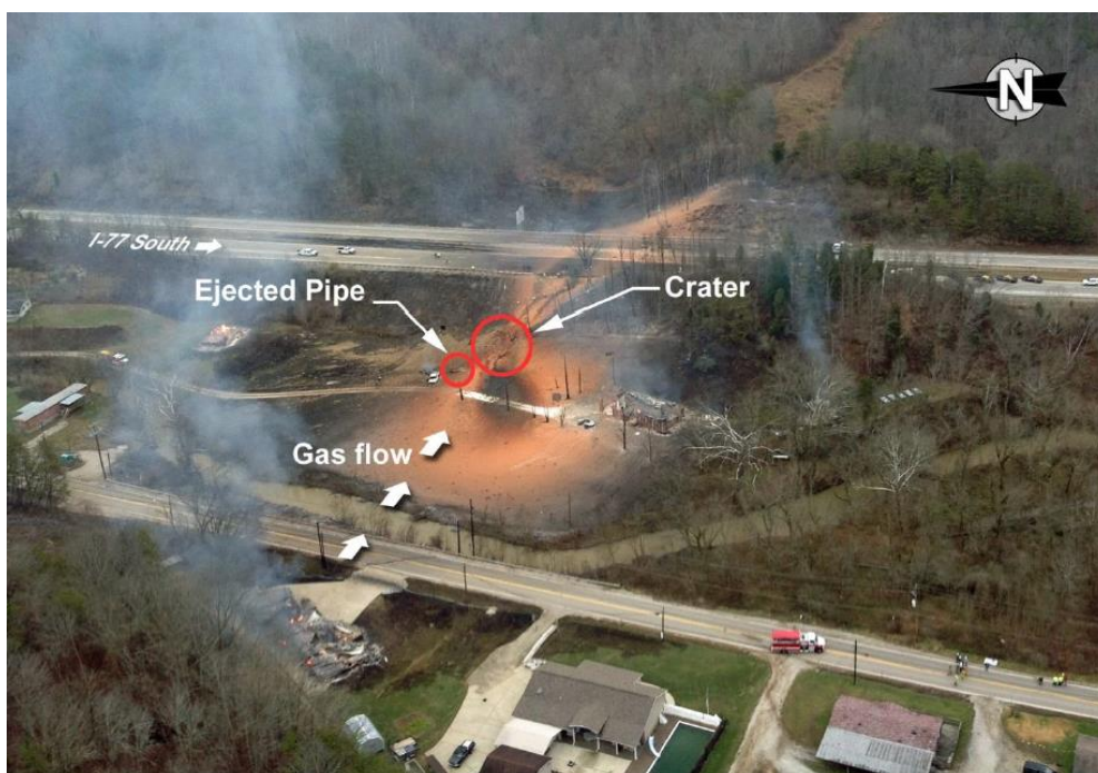
Figure 1-6 Damage following the Sissonville incident. Reproduced from (24)
