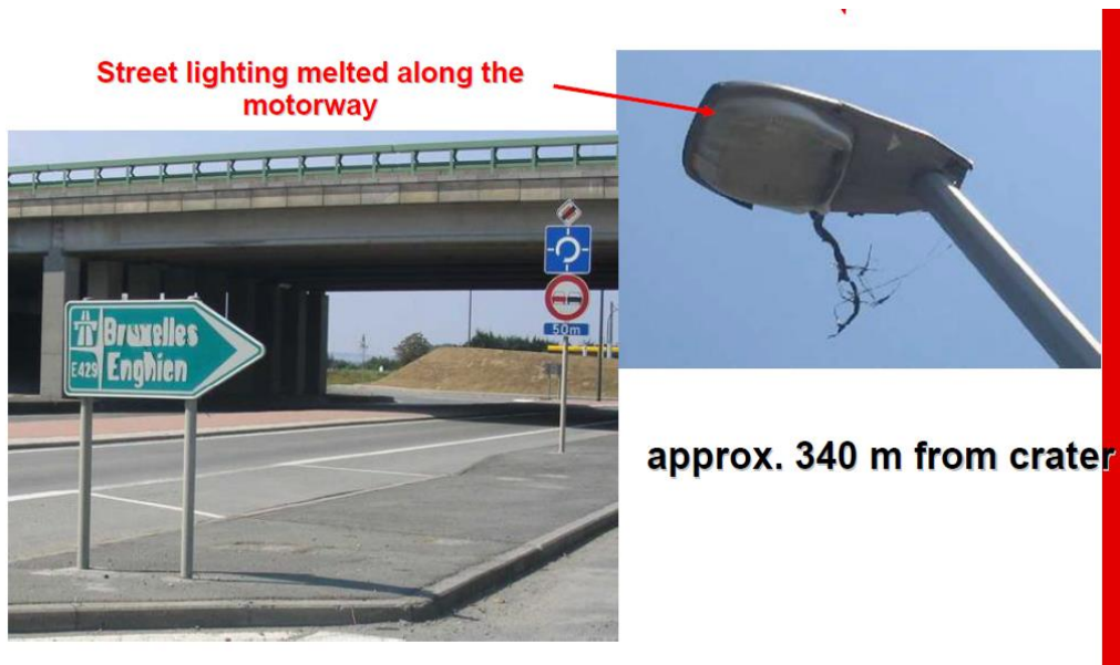
Figure 2-45 Damage caused to street lighting. Reproduced from (26)
