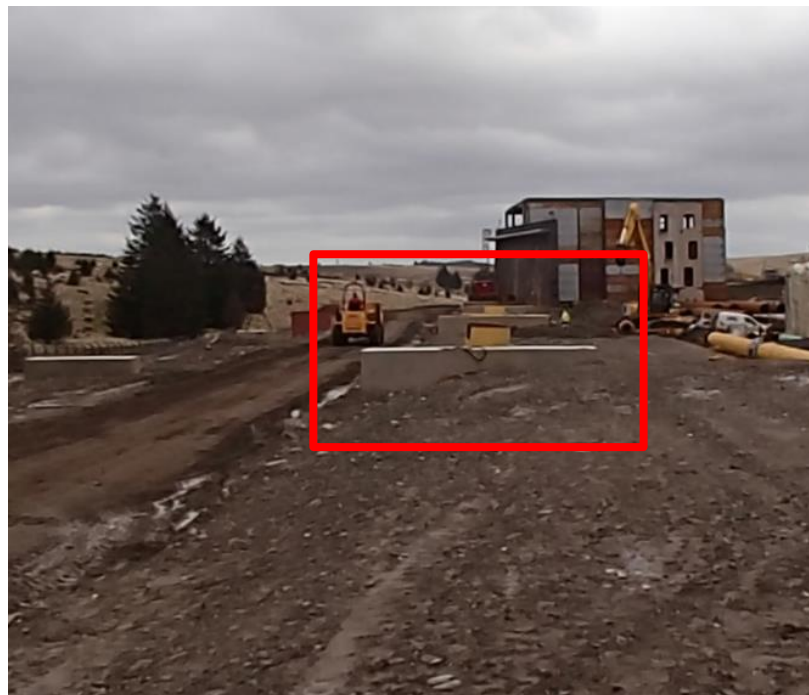
Figure 3-4 Photograph showing the top of concrete anchors installed around the reservoir
