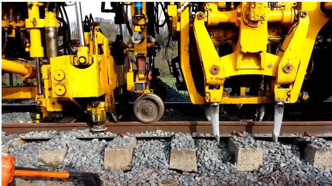
Figure 2.5 Ballast tamping machine
