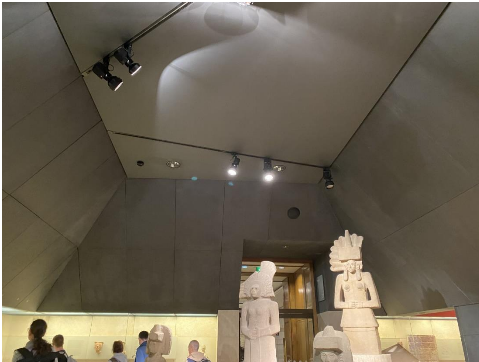
Figure 8: View of corbelled roof.
