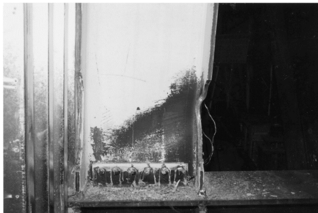
Figure 2.13: Typical plastic zone of the composite RBS specimen tested (Chen and Chao, 2001).
