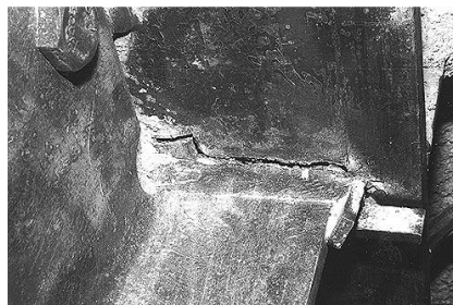
a) Fracture at fused zone.
