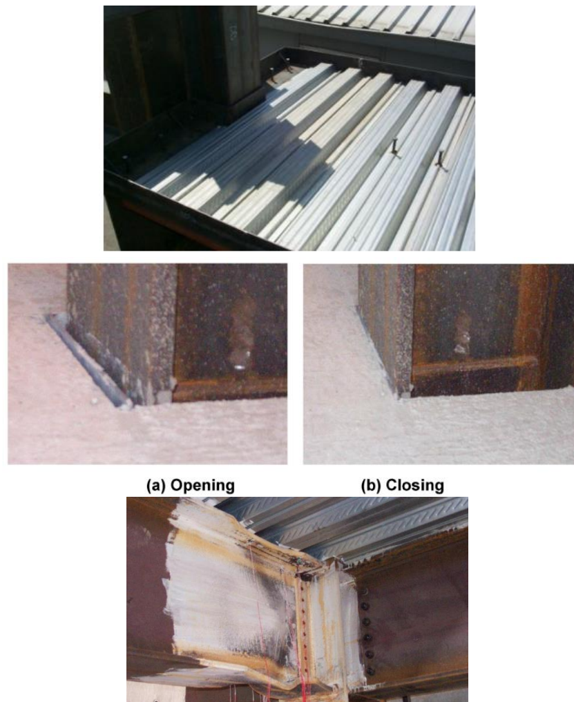
Figure 2.15: Composite RBS connection, before, during and after the test (Lee et al., 2016)
