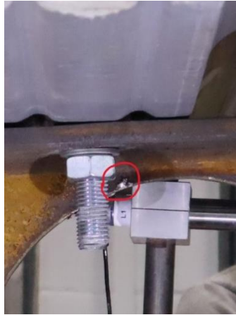
a) Steel peeling off during 4% rotation.
