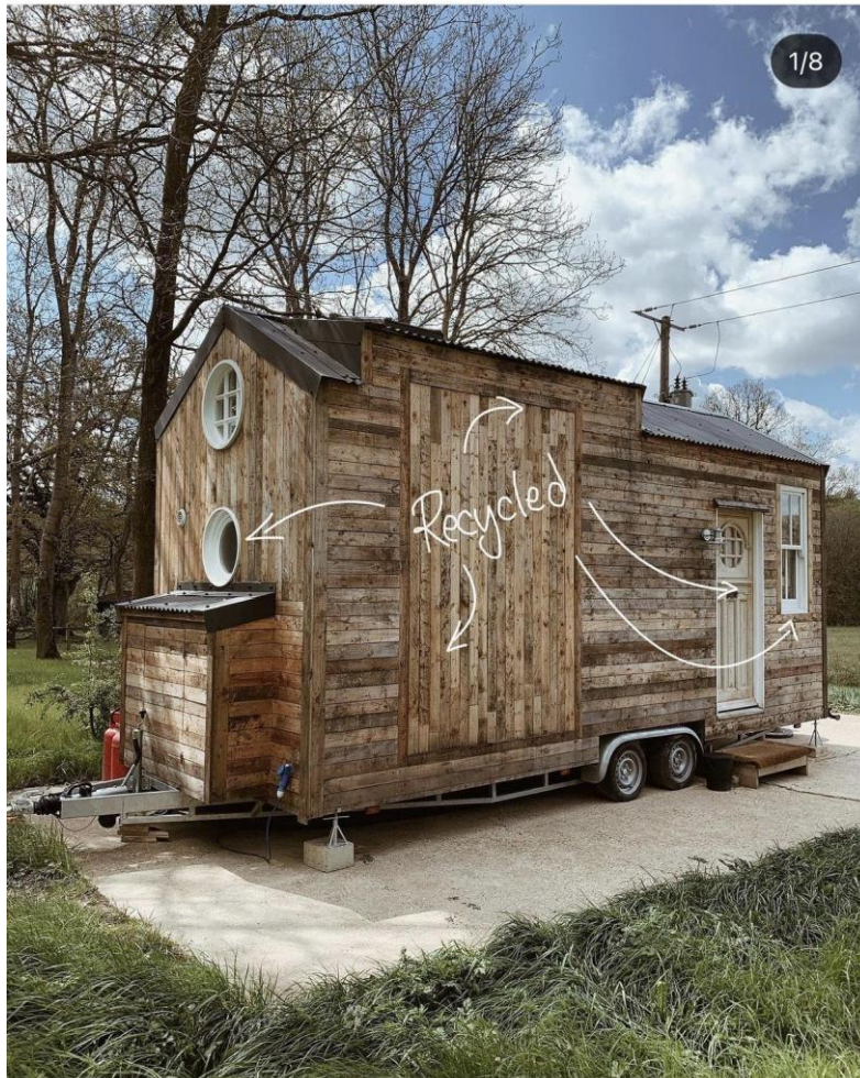
Figure 6: An image taken by one of my participants. This style of tiny home is a classic example of a timber framed tiny on wheels, or THOW.
