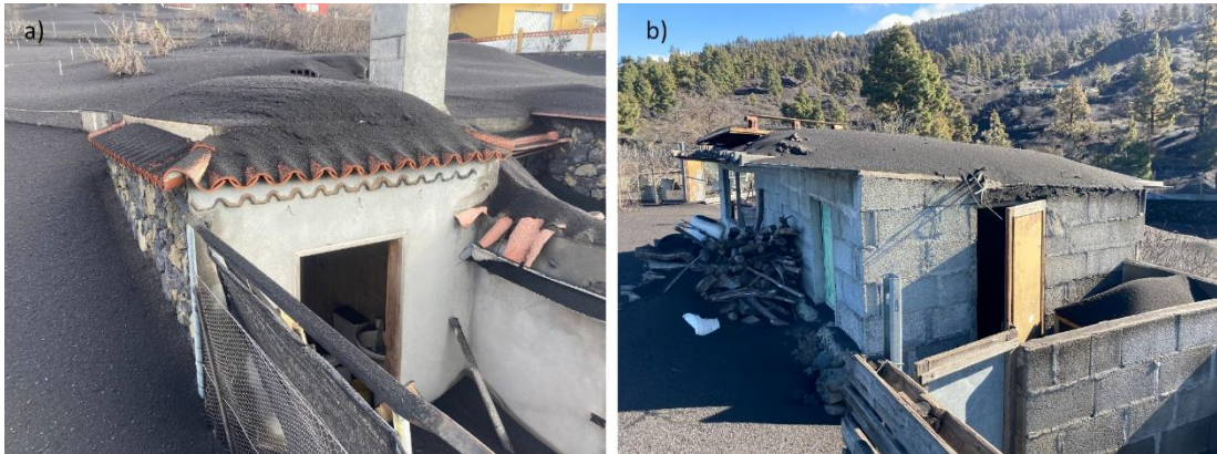
Fig. 3-9 Low pitched roofs in a) Las Manchas and b) Tacande, La Palma following the Cumbre Vieja 2021 eruption, showing no evidence of the deposit sliding except at the deposit edges where the angle of repose has been formed
