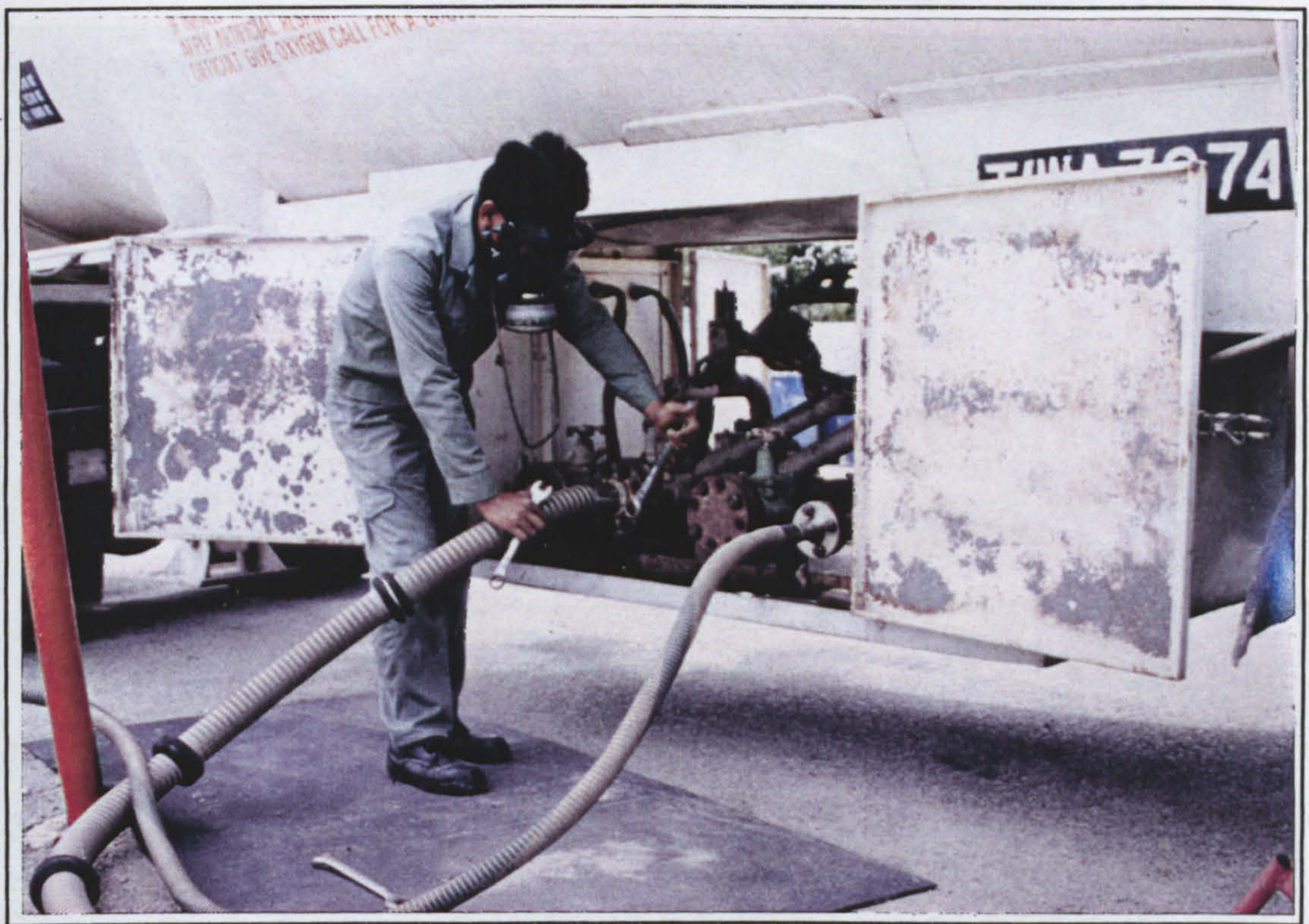
Figure A8.1. Connecting flexible hoses for ammonia road tanker loading at Site A
