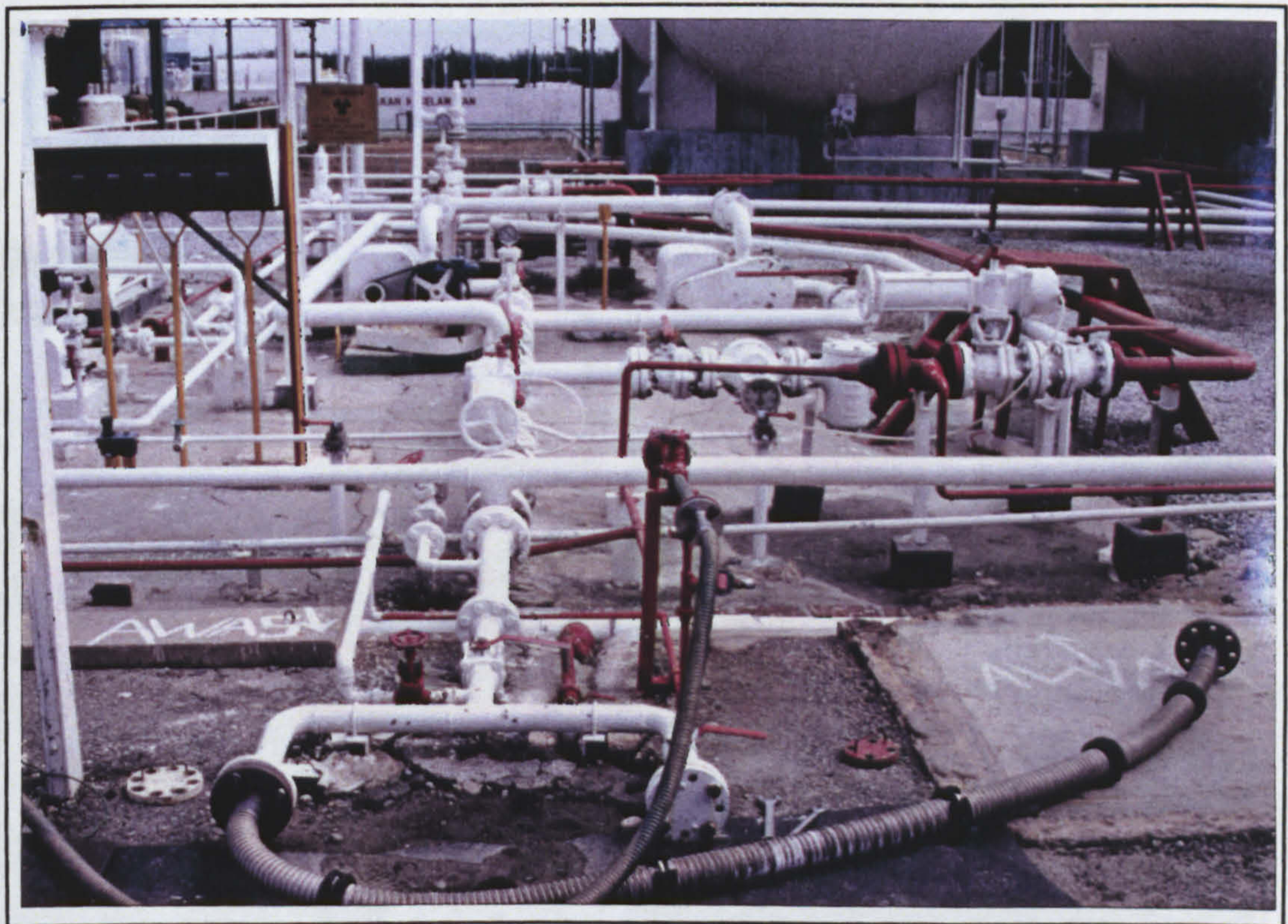
Figure A8.2. Piping arrangement for ammonia road tanker loading at Site A
