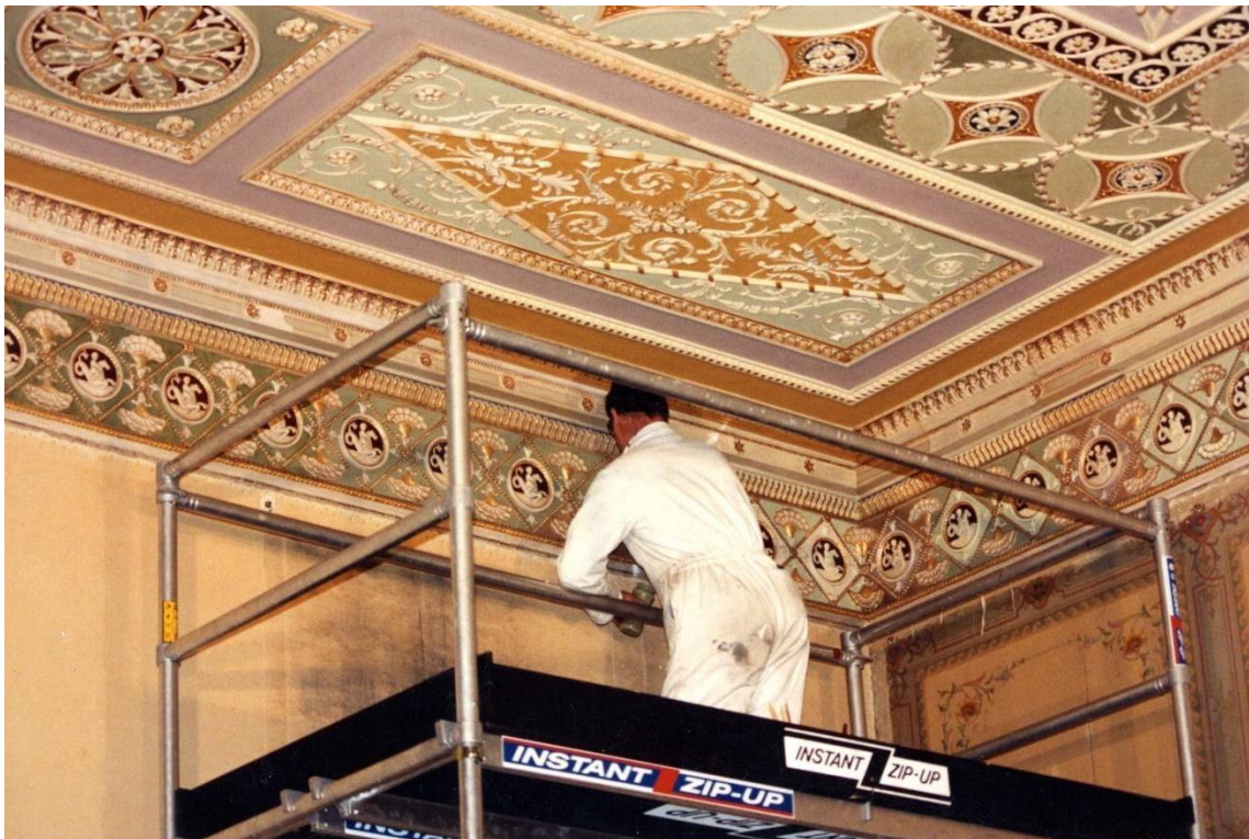
Figure 17: Yellow Drawing Room, Harewood House, during the restoration of the room in the 1990s (HHPA). The Victorian painted canvas has been uncovered on the wall to the right.
