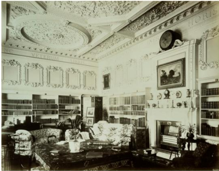
Figure 11: Library, Chesterfield House, by Bedford Lemere and Company, 17 August 1886 (Historic England Archive, BL06608).
