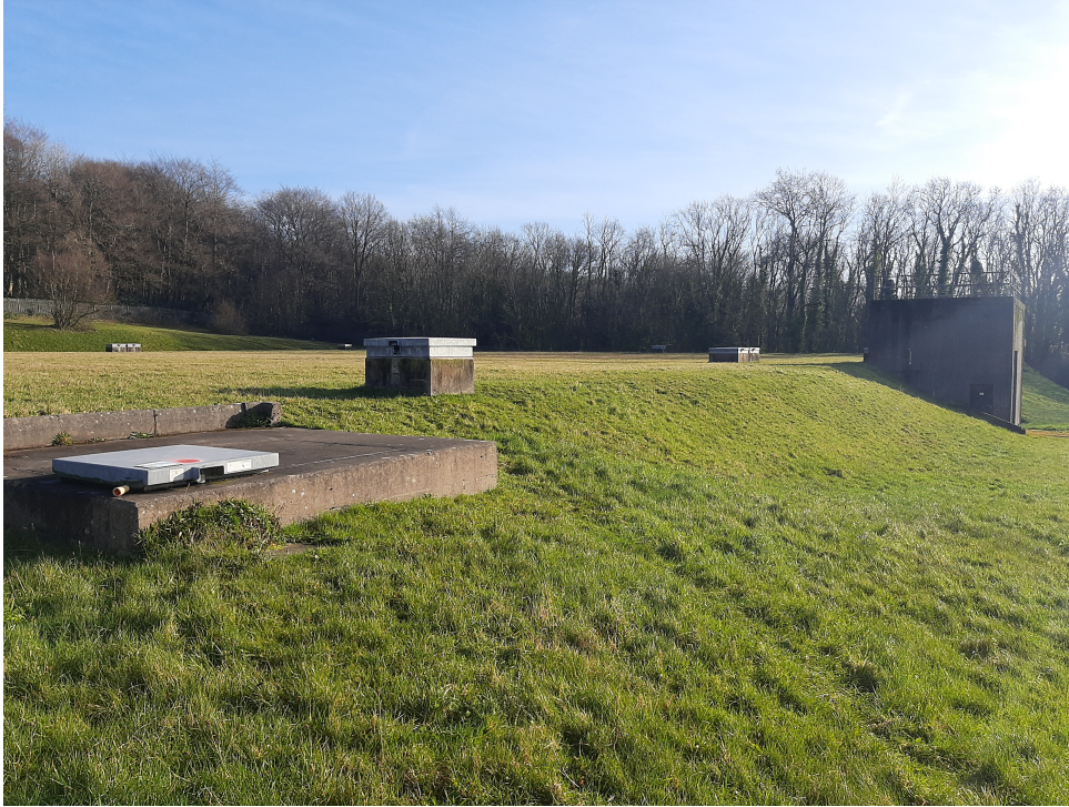
Figure 2.1: Example of a grass covered underground service reservoir in the UK.
