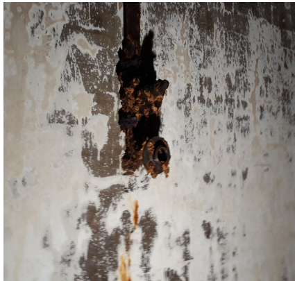
(c) Corrosion problem on a SR wall.
