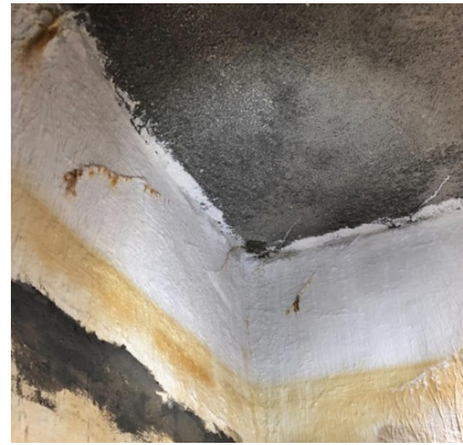
(b) SR top wall leak.
