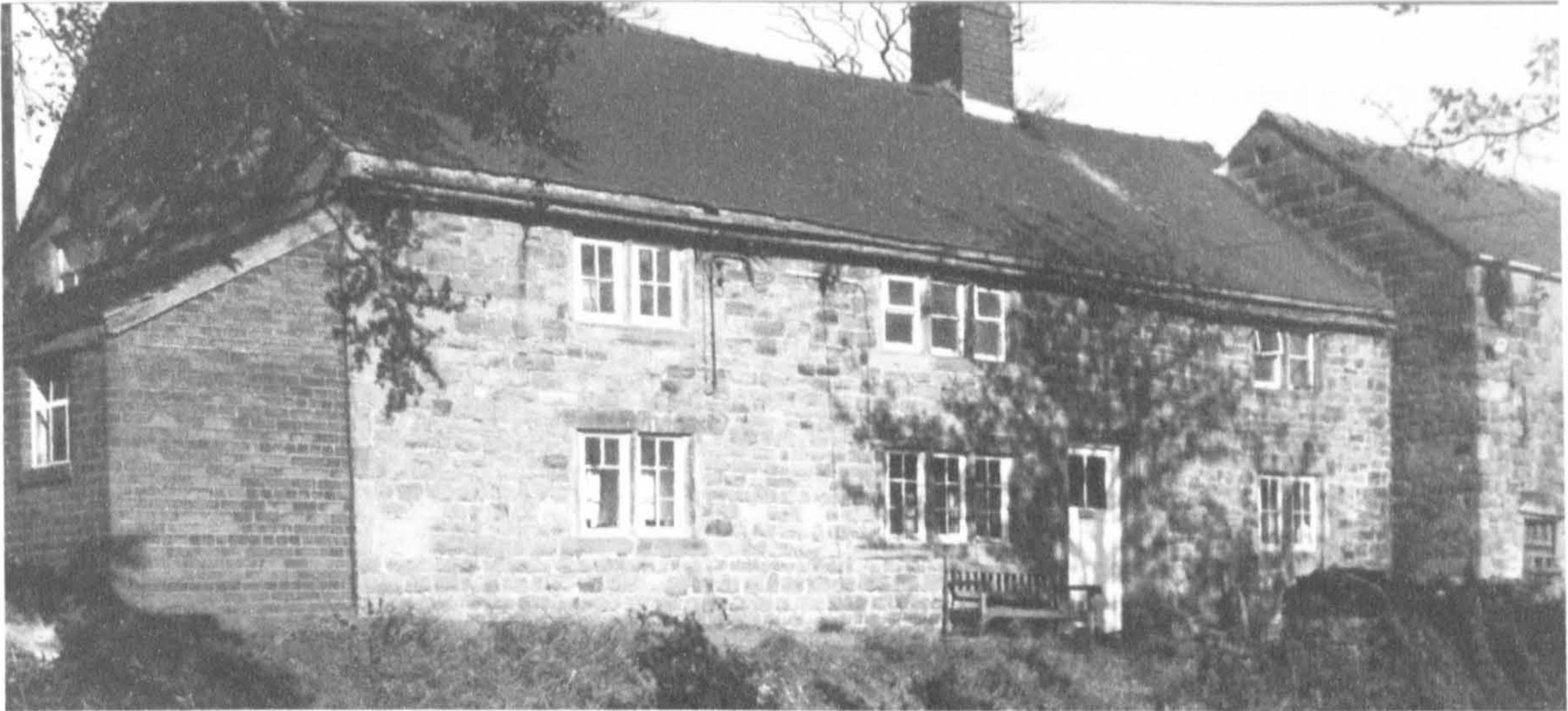
Fig. 50 Brownege from the south east.
