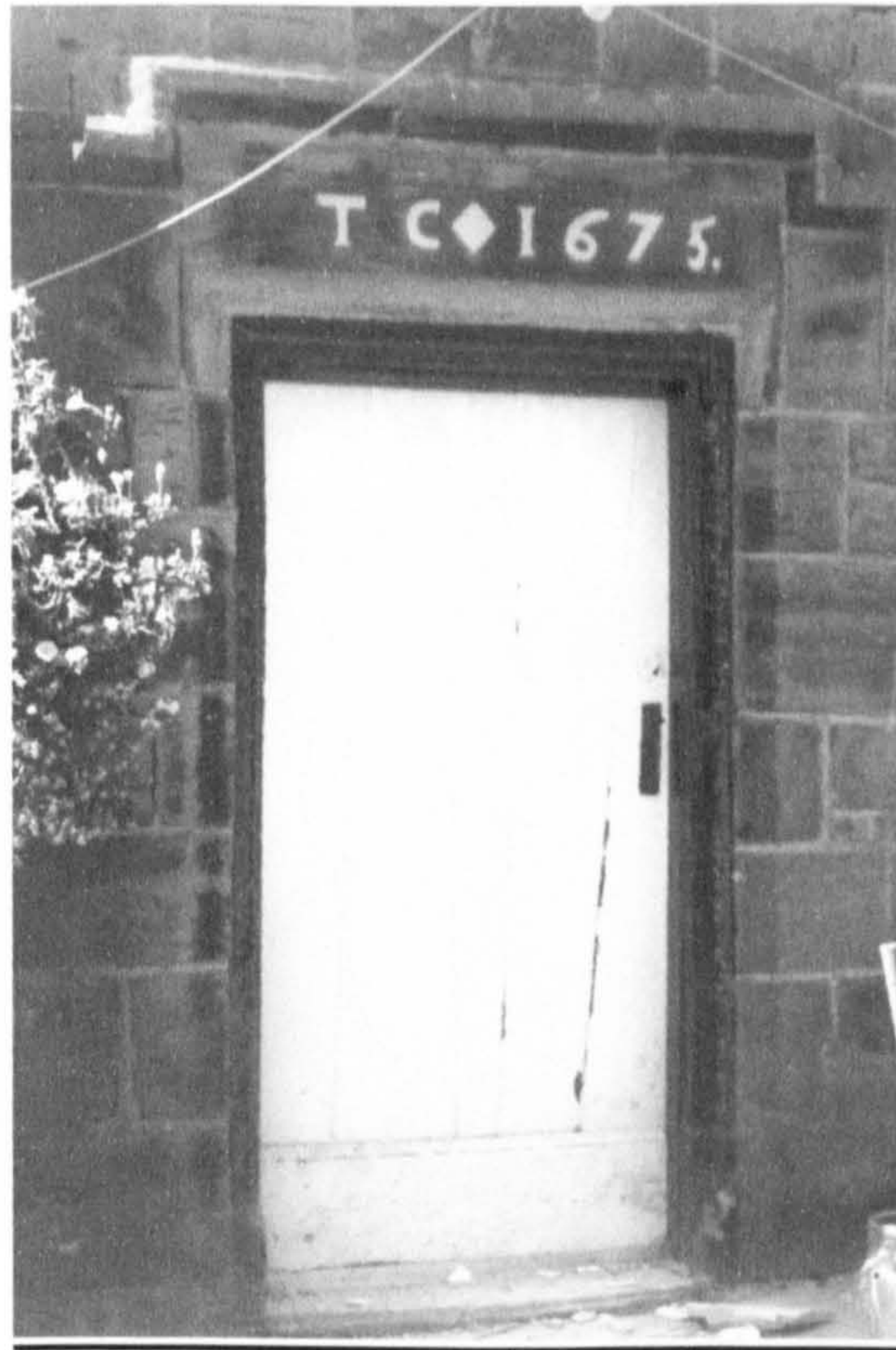
Fig. 84 Jackhaye: moulded doorway of 1675
