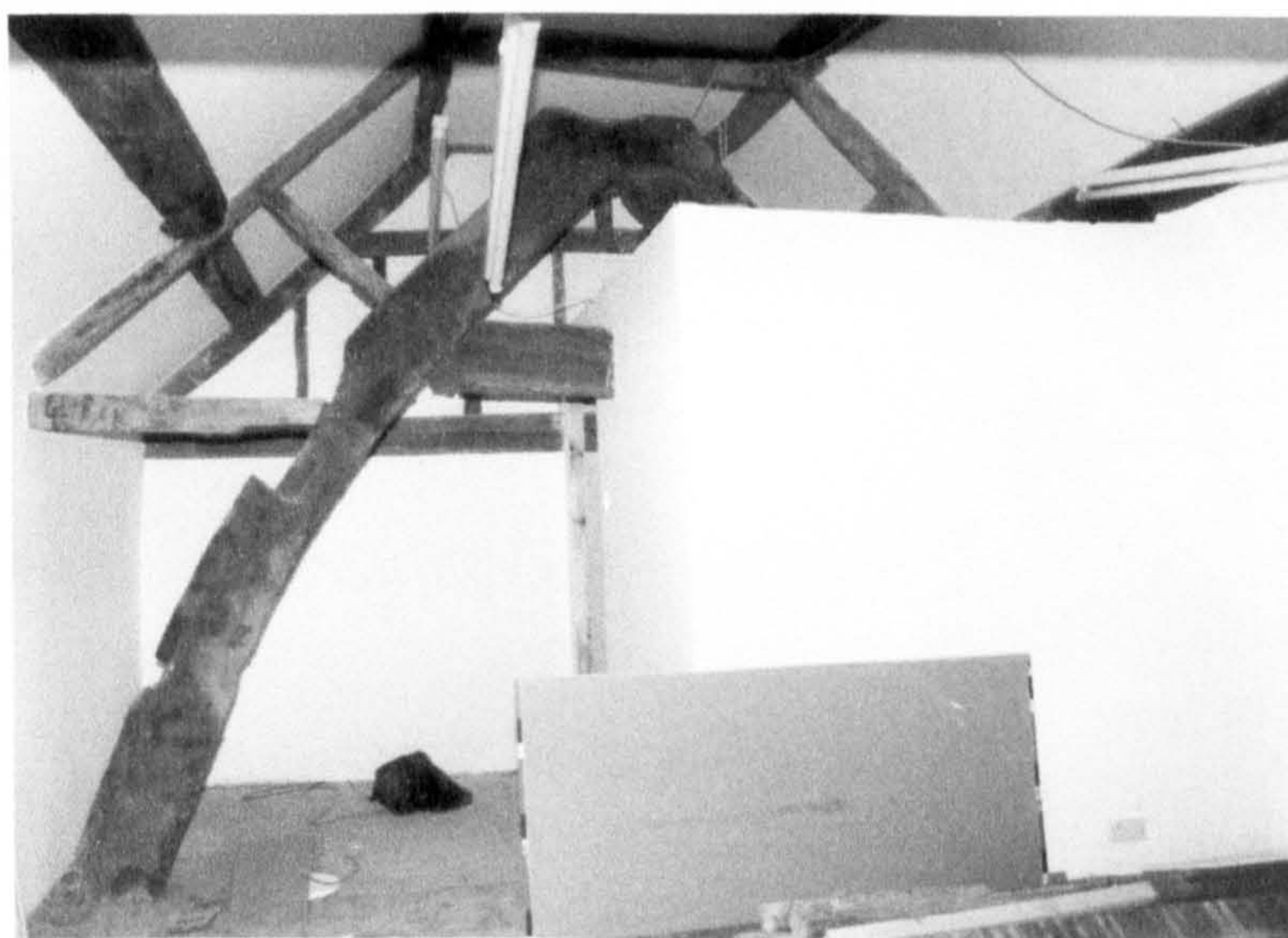
Fig. 60 Gunside: during building work in 1999.
