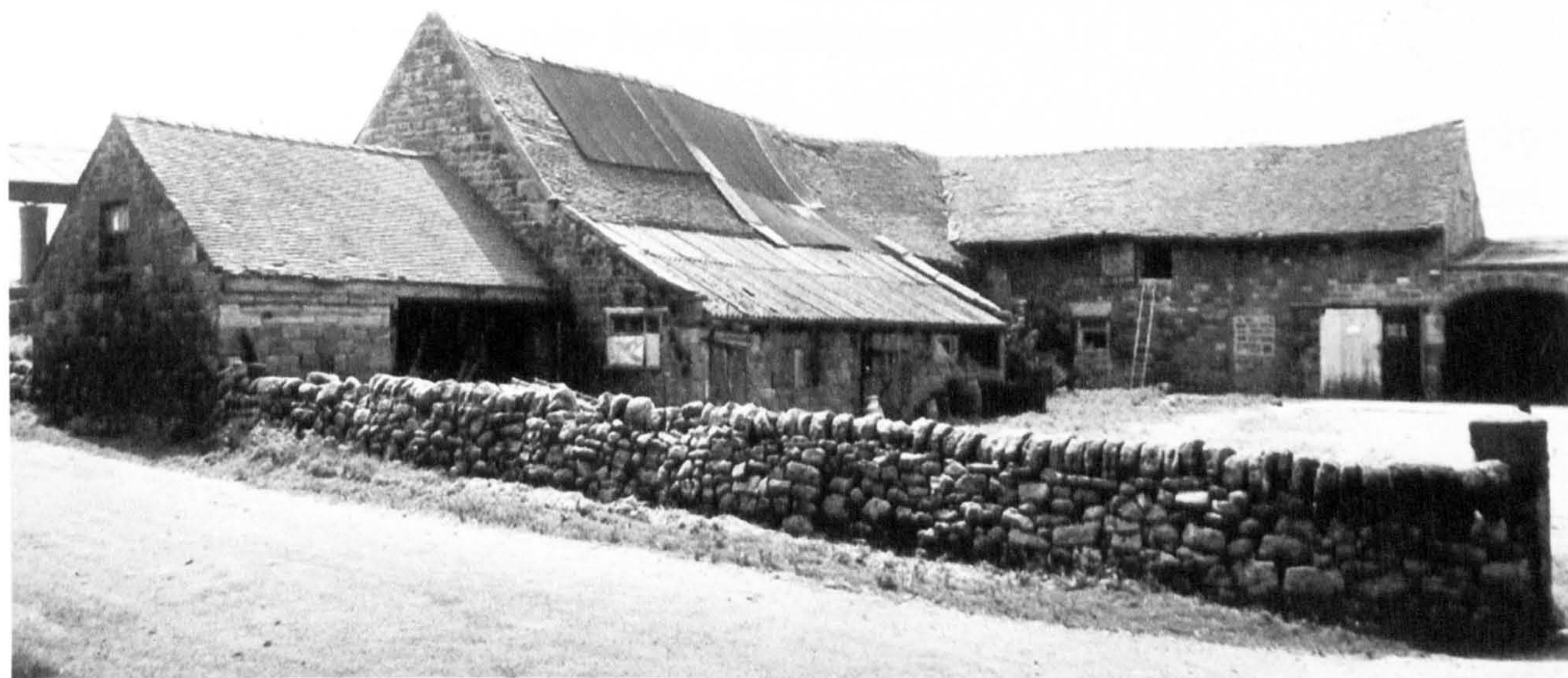
Fig. 72 Little Longsdon: the cruck barn before demolition in 1985. Photographs loaned by A.G. Busfield
