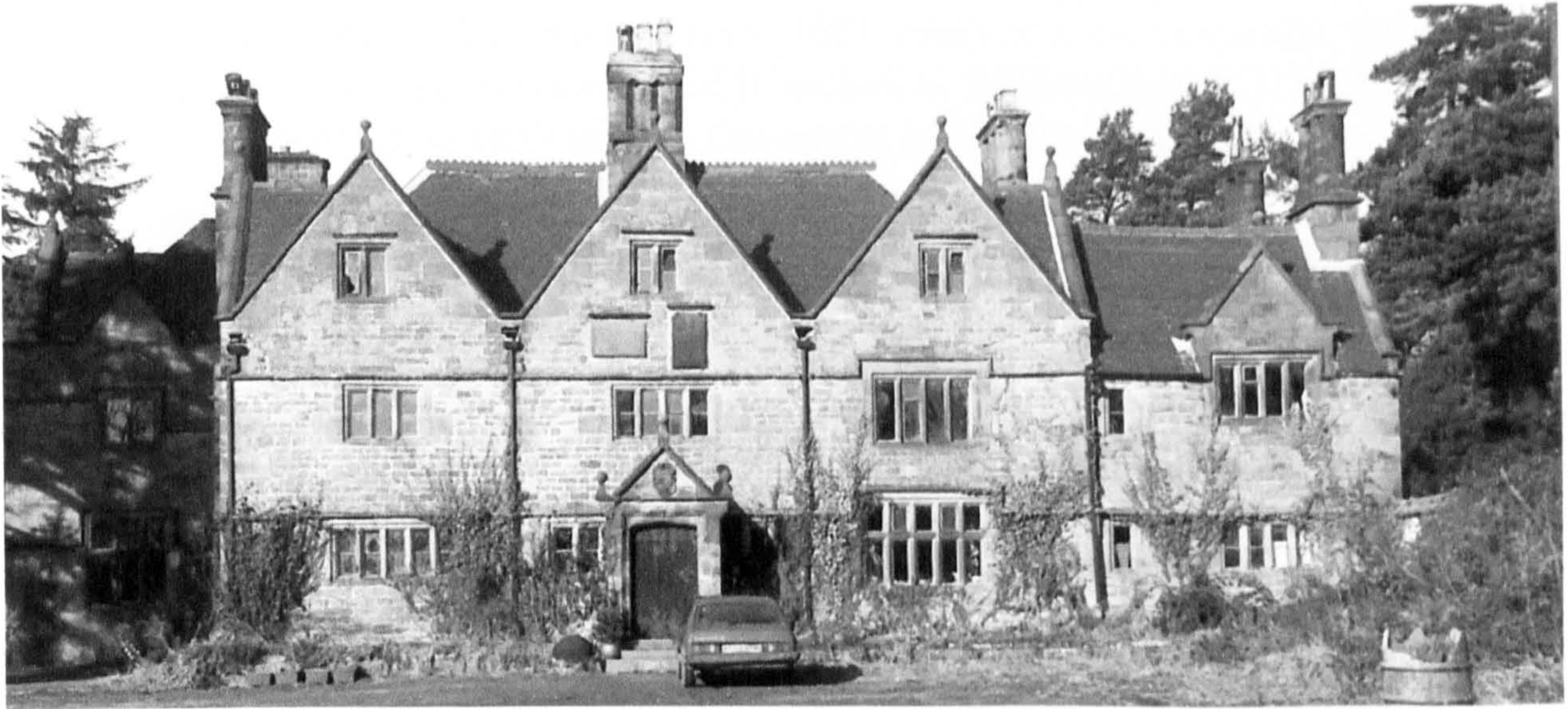
Fig. 55 Sharpcliffe Hall: from the south east showing the altered roofline.
