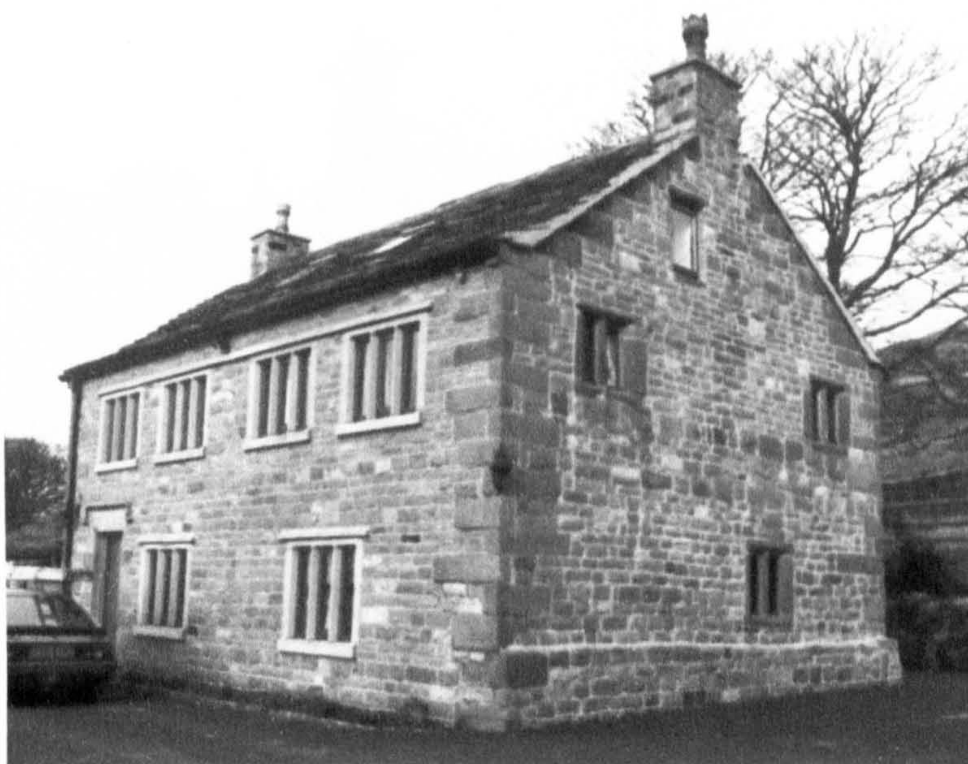
Fig. 36 Hangingstone: from the south west showing the reconstructed front and original gable
