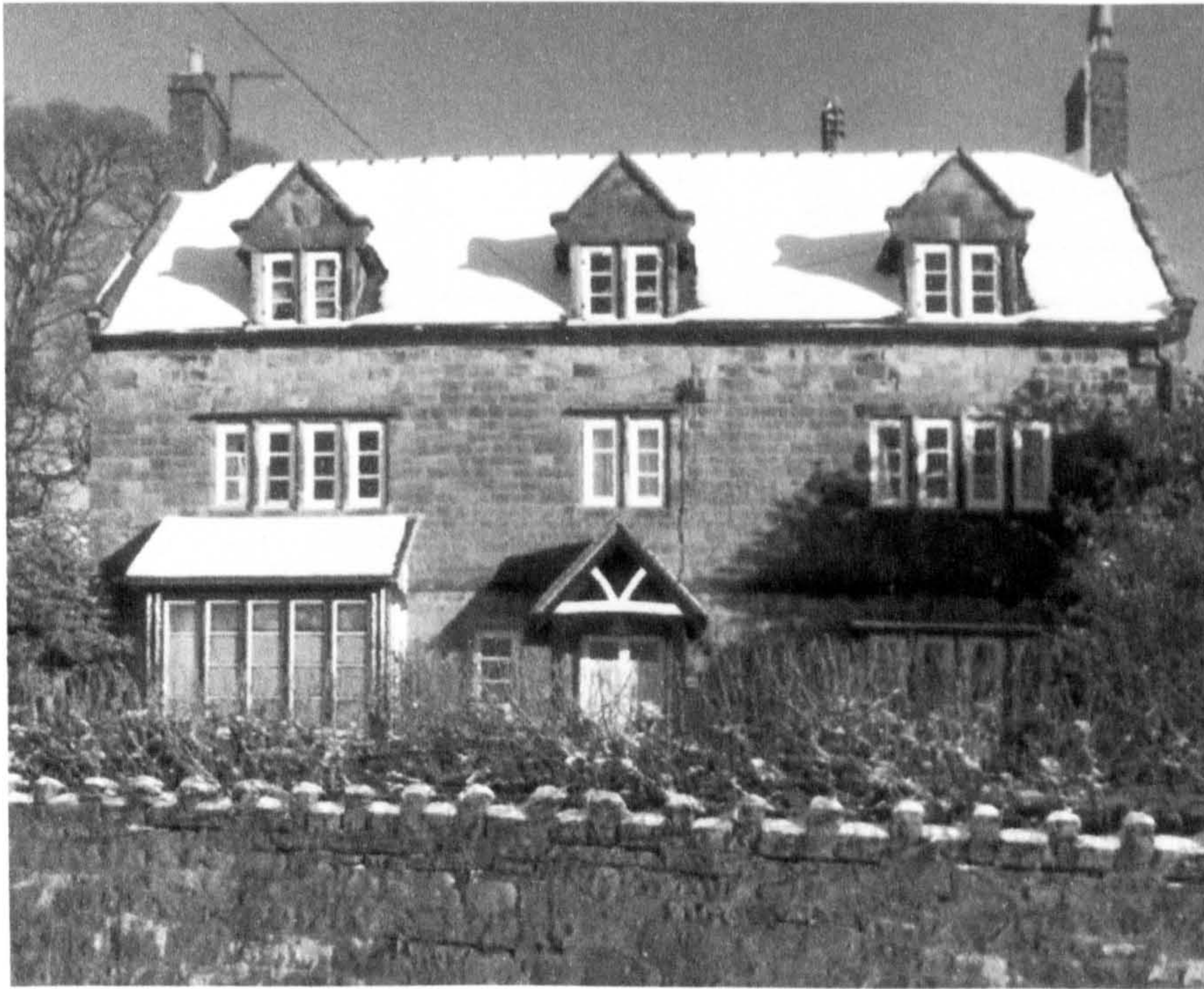
Fig. 69 Dunwood House Farm
