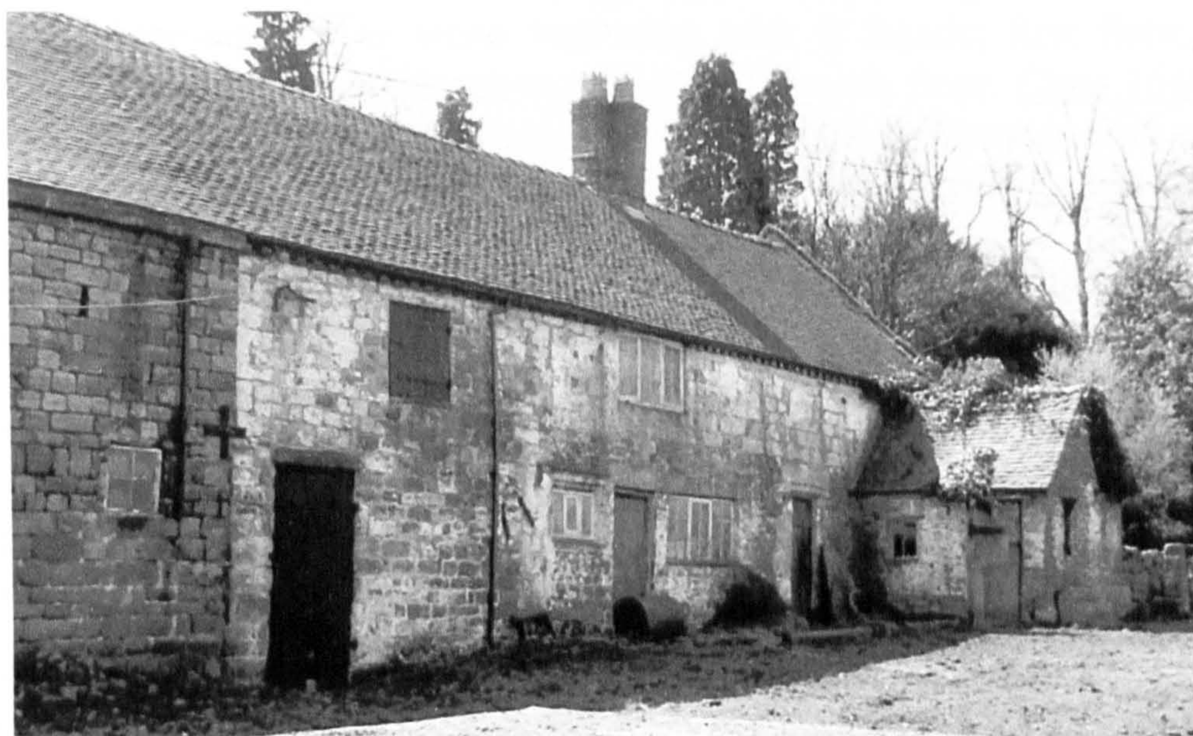
Fig. 22 Felthouse: from the northeast
