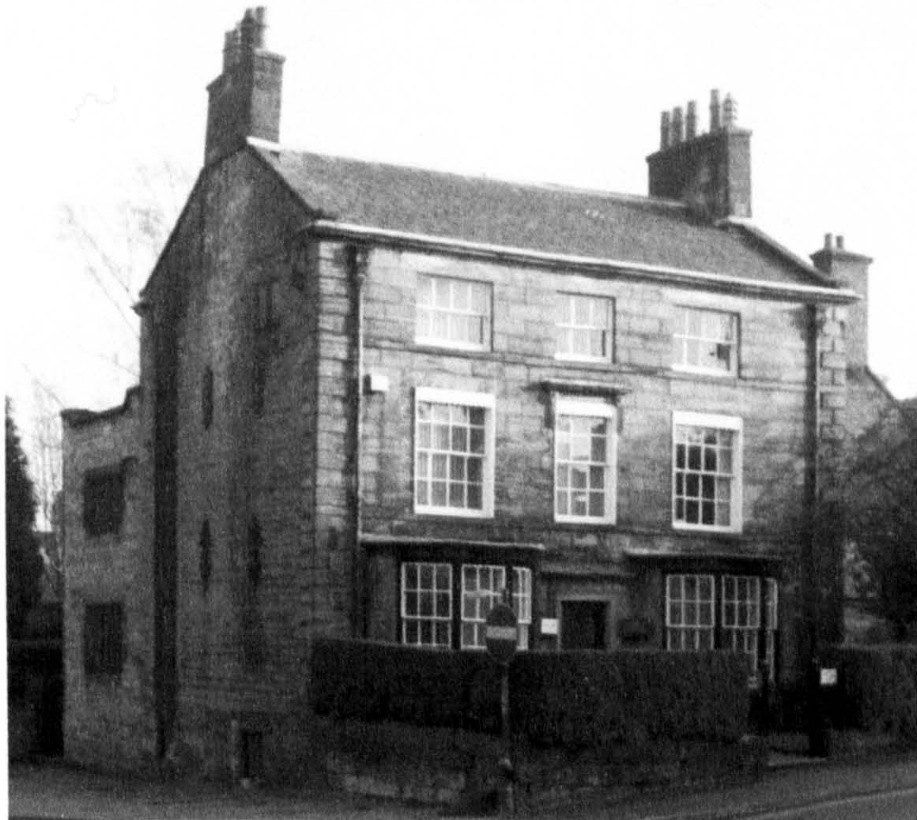
Fig. 3 Ford House from the north west
