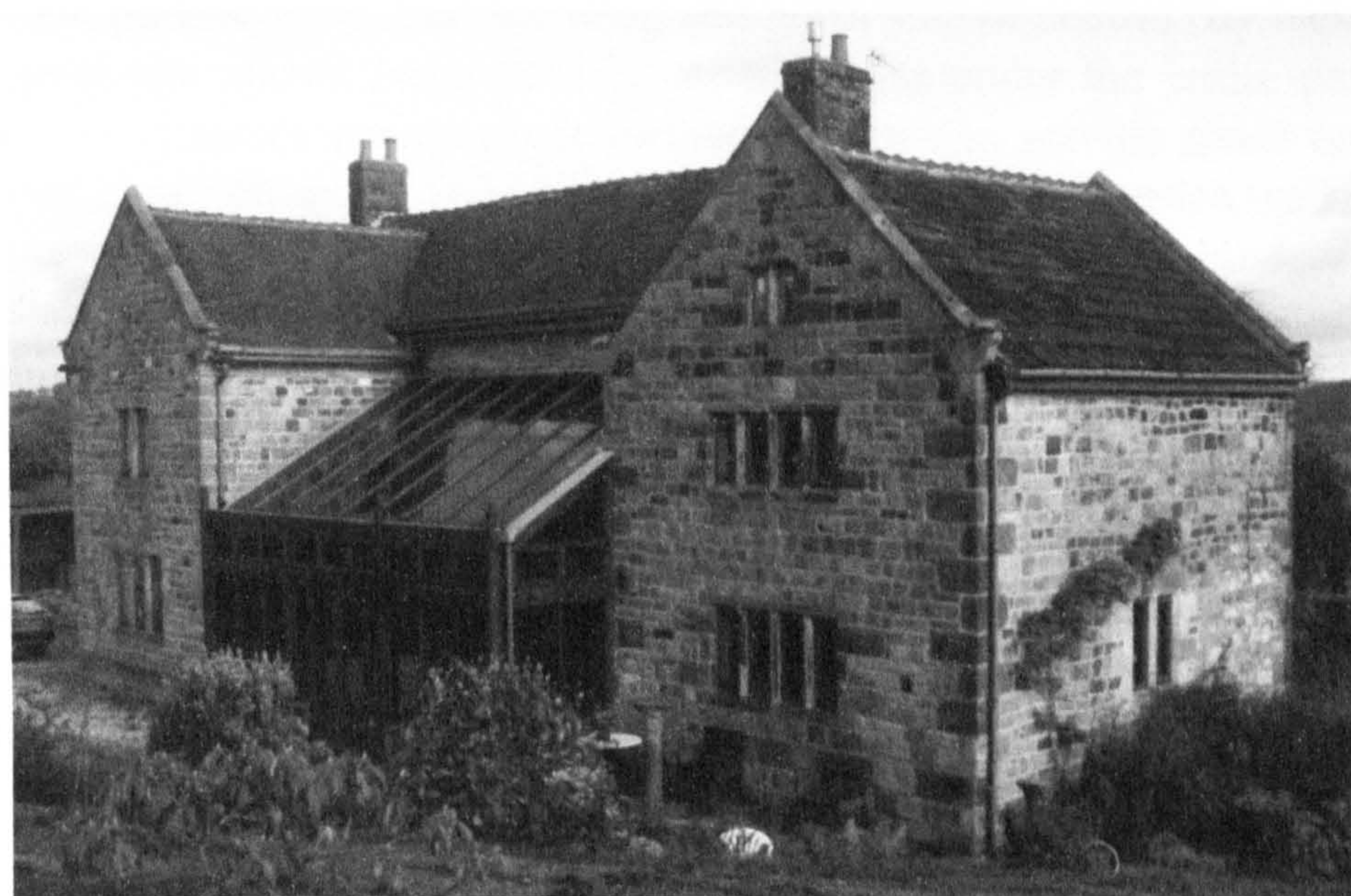
Fig. 43 The Fields : (above) the front of the main range. (below) the rear with the original crosswing in the foreground.
