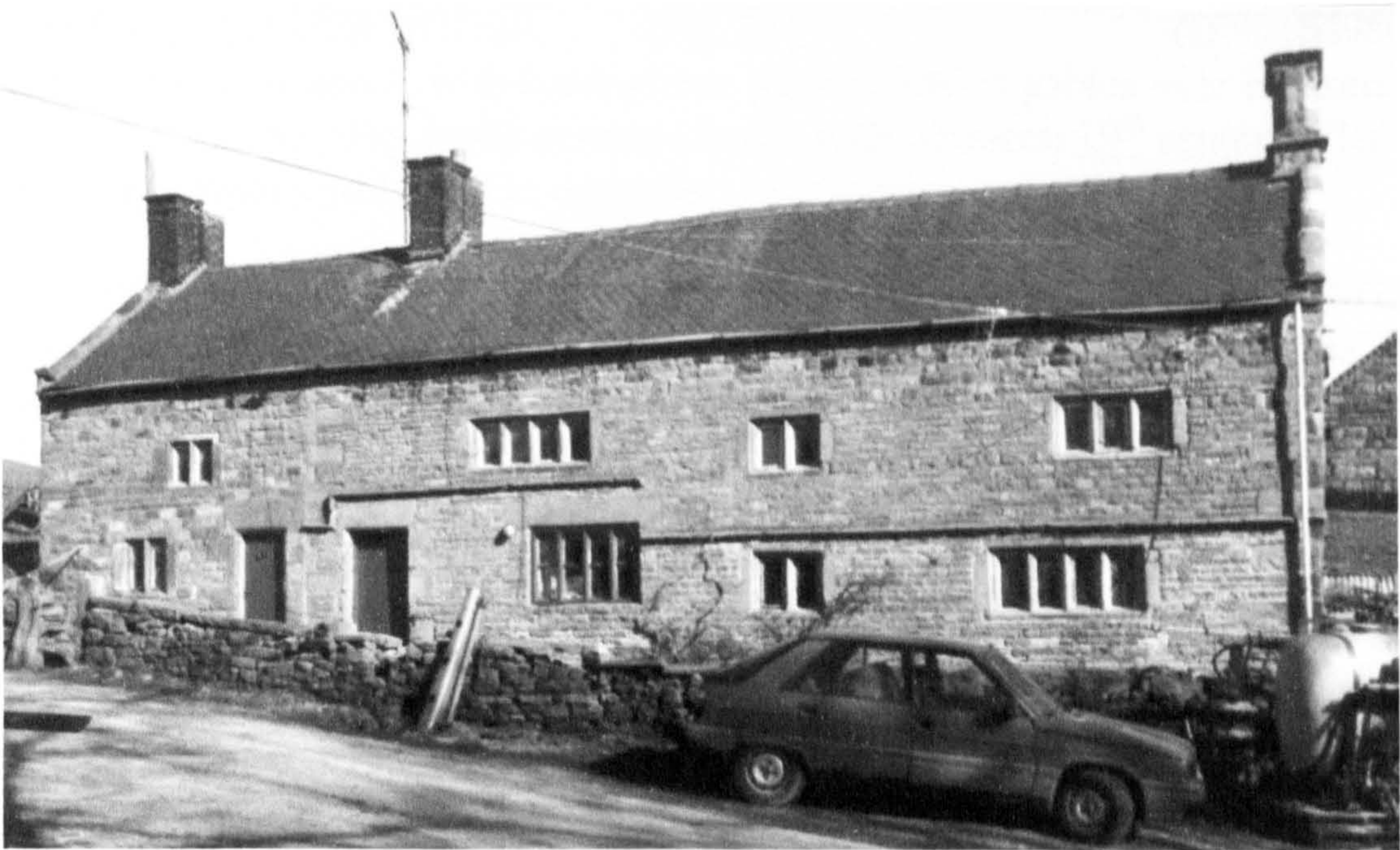
Fig. 17 Basford Bridge: from the south
