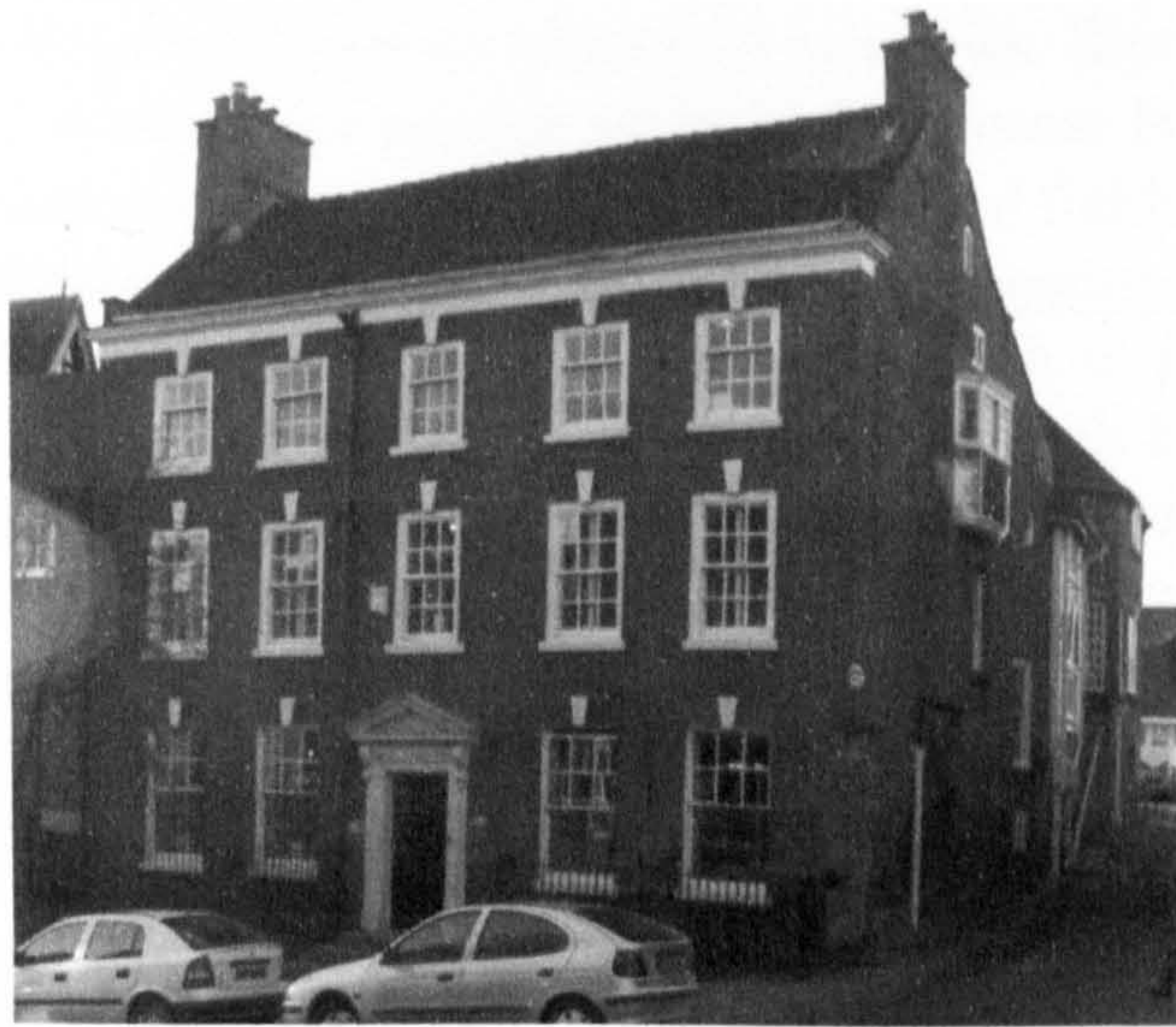
Fig. 9 54 St. Edward's Street: from the north
