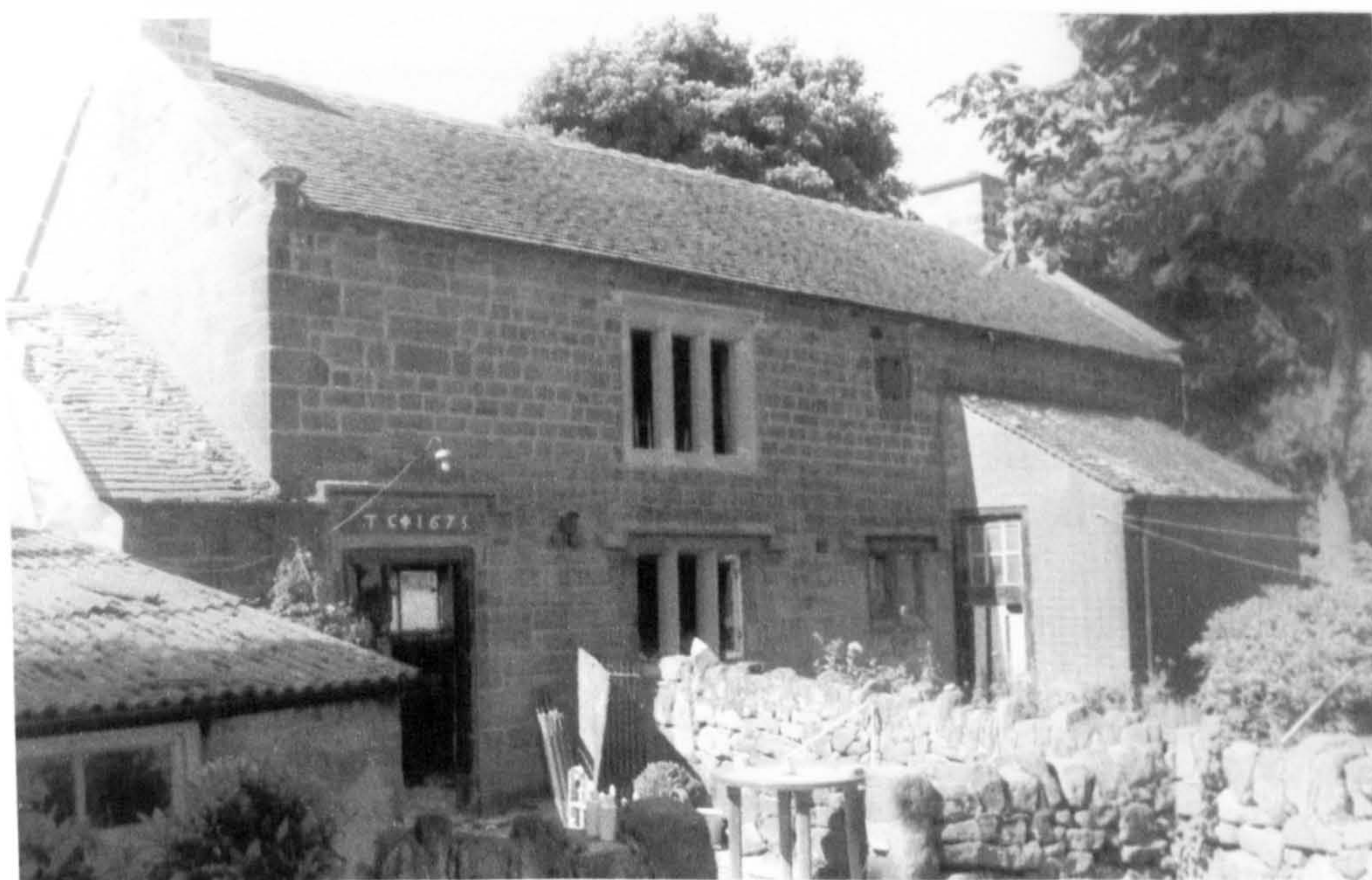
Fig. 6.68 Jackhaye, Bagnall: from the north
