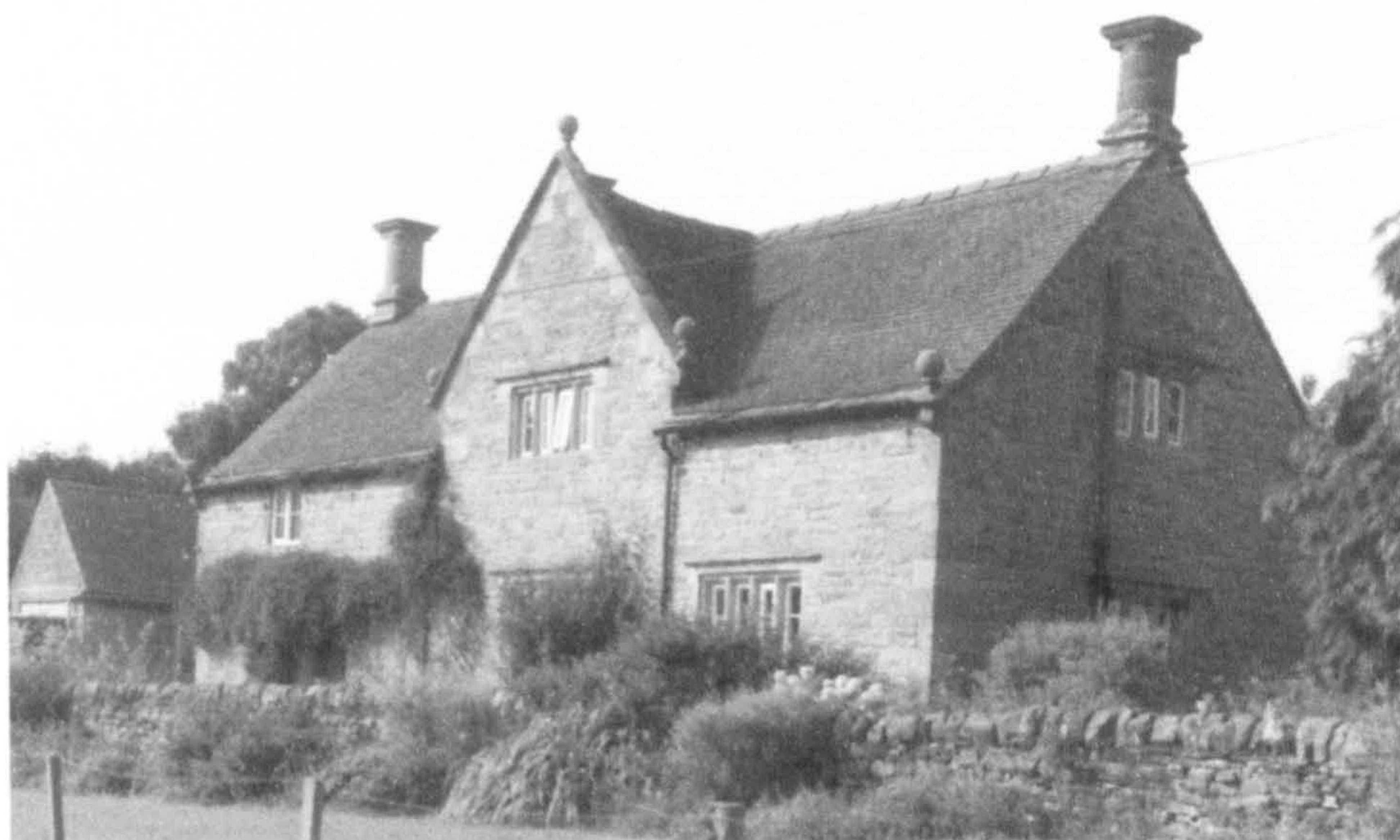
Fig. 6.75 The Old Hall, Ford (above) from the south east. (below) the ground plan.
