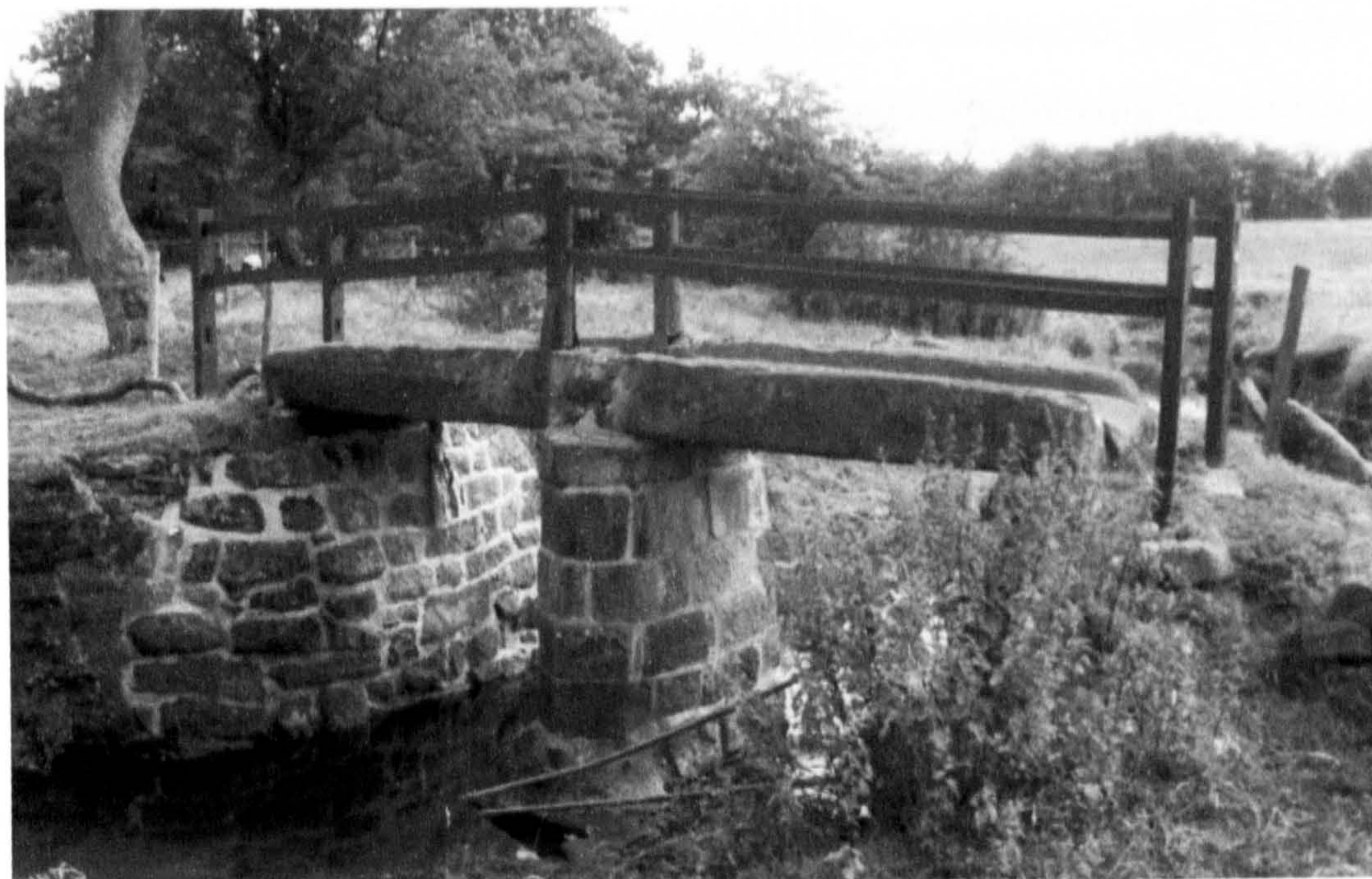
Fig. 4.4 The clapper bridge between Horton and Gratton
