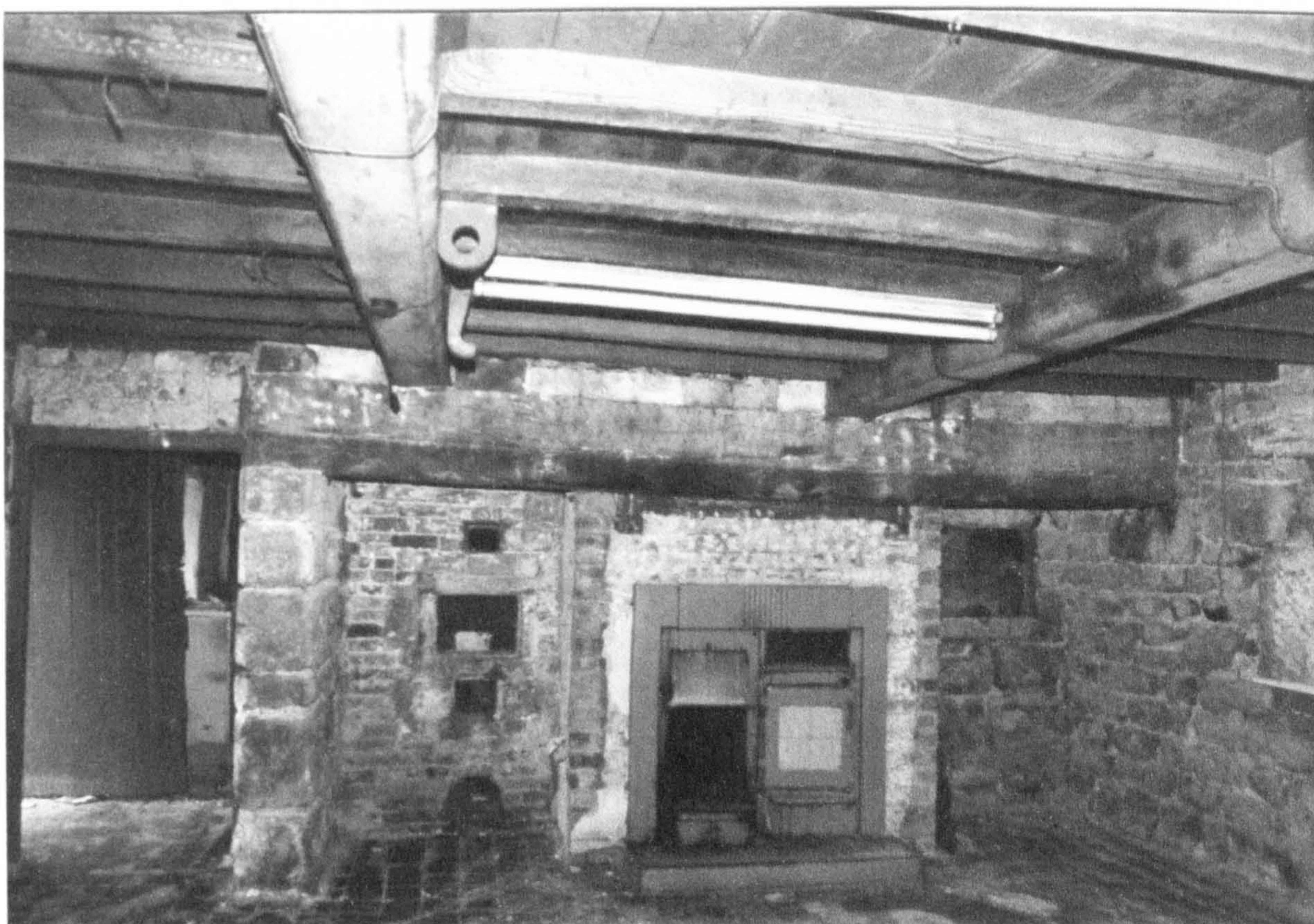
Fig. 6.130 Rownall: the houseplace during restoration work in the 1990s.
