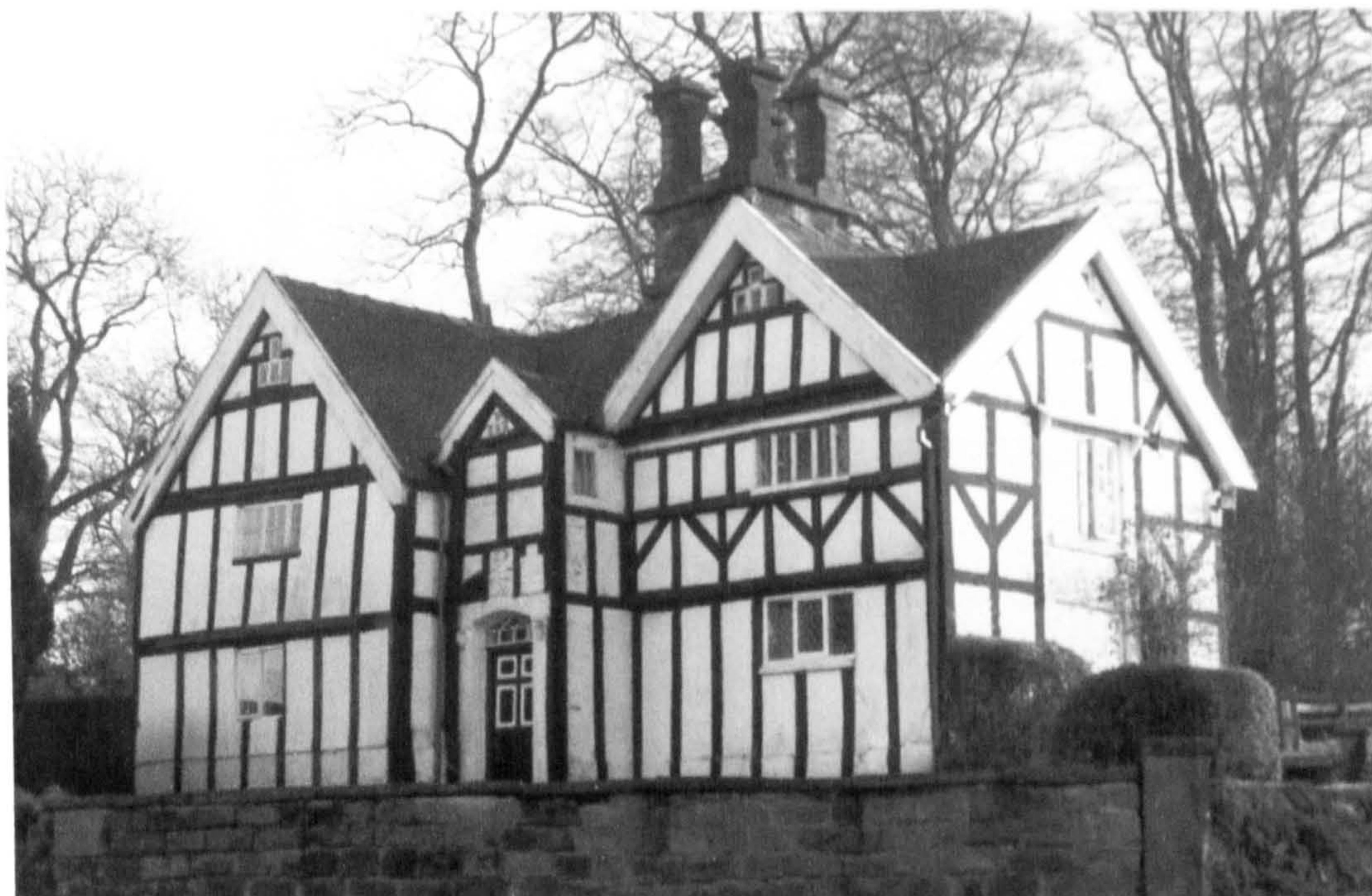
Fig. 6.39 Wallhill, Rushton Spencer: from the north west. Render and paint covers the majority of the timber-framing.
