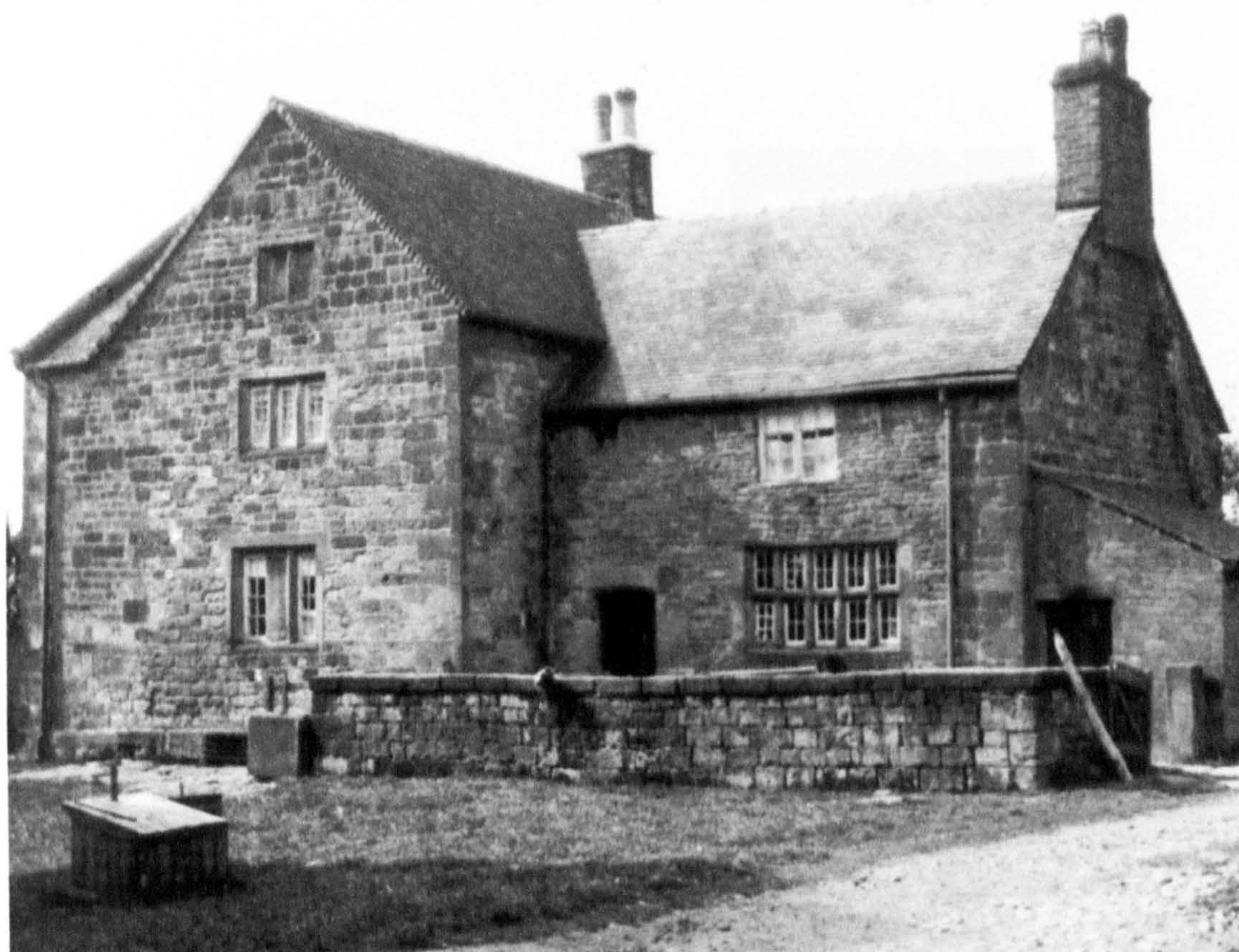
Fig. 6.12 (below) Fairboroughs from the east showing the added 'backhouse'. The ragged joint on the left of the service wing is the result of nineteenth century extension.
