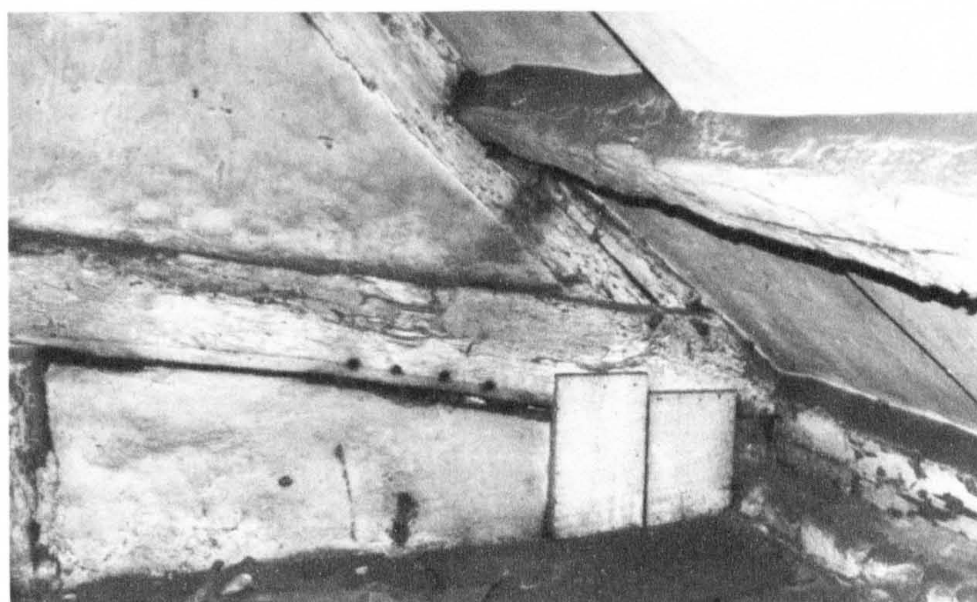
Fig. 6.98 Detail of an open truss in 2-4 Church Street.
