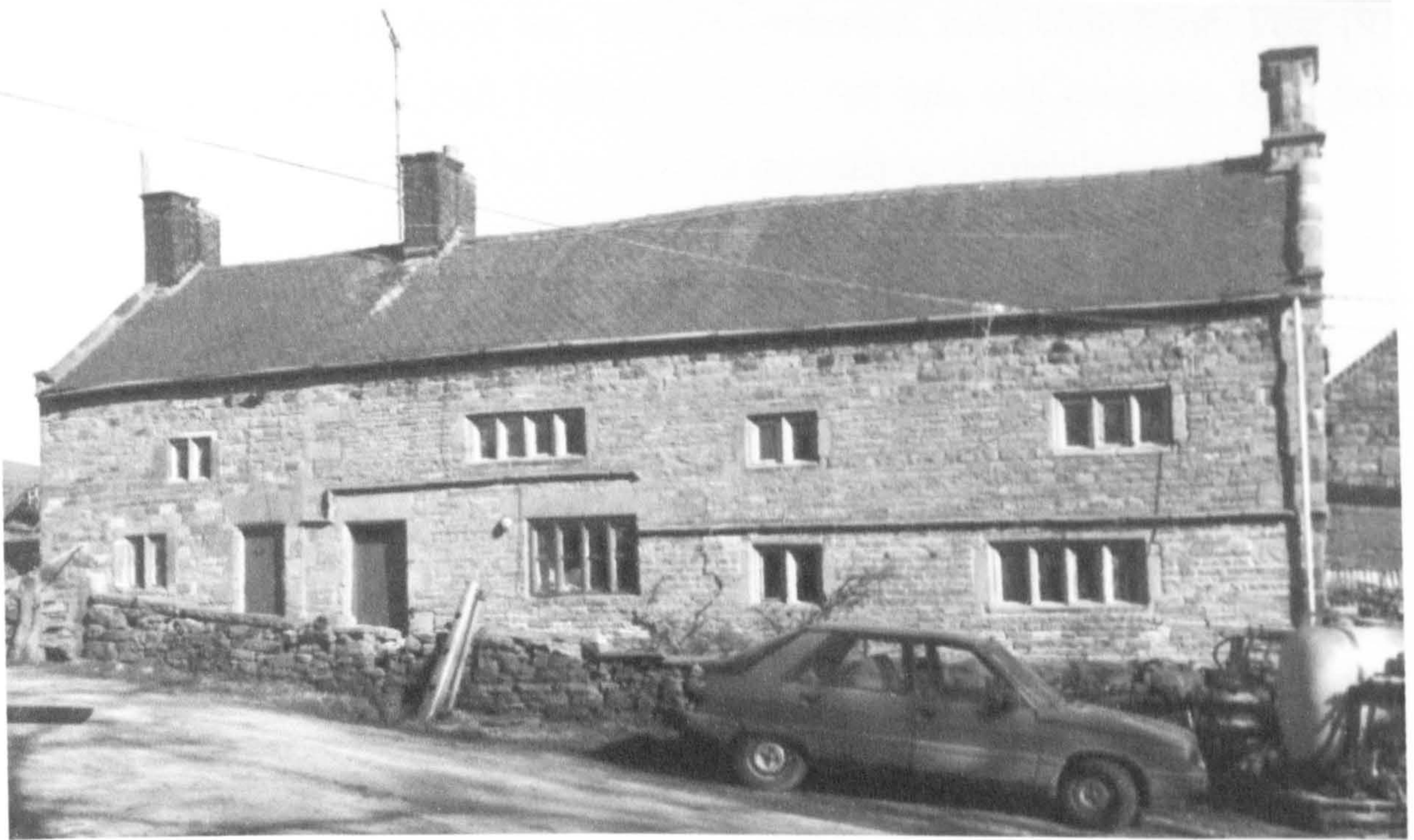
Fig. 6.73 Basford Bridge, Cheddleton: (above) from the south
