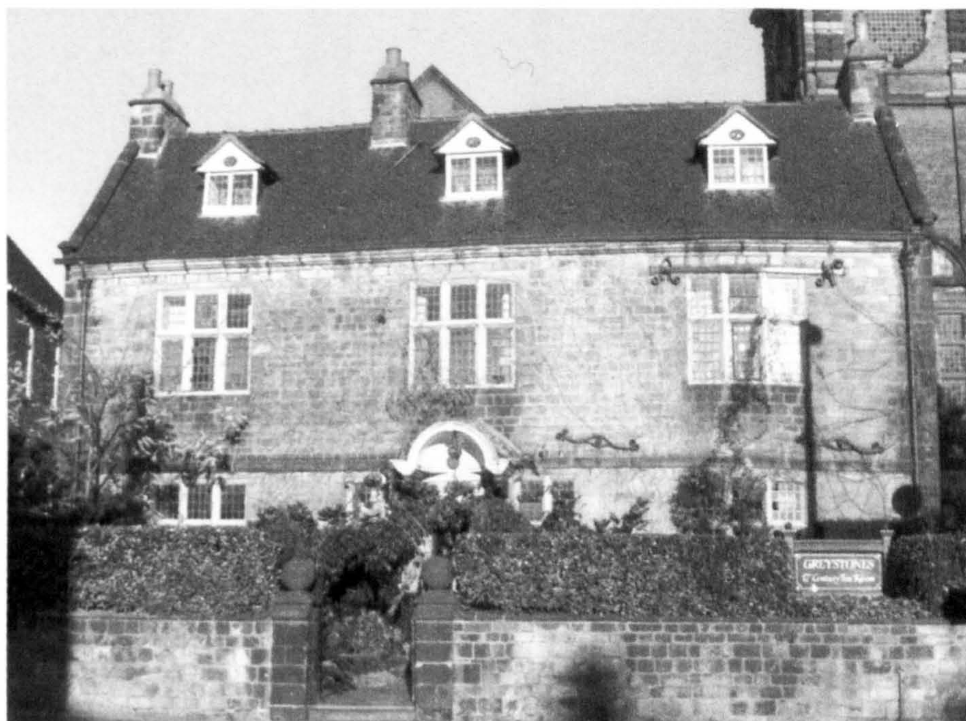
Fig. 6.115 Greystones: from the south
