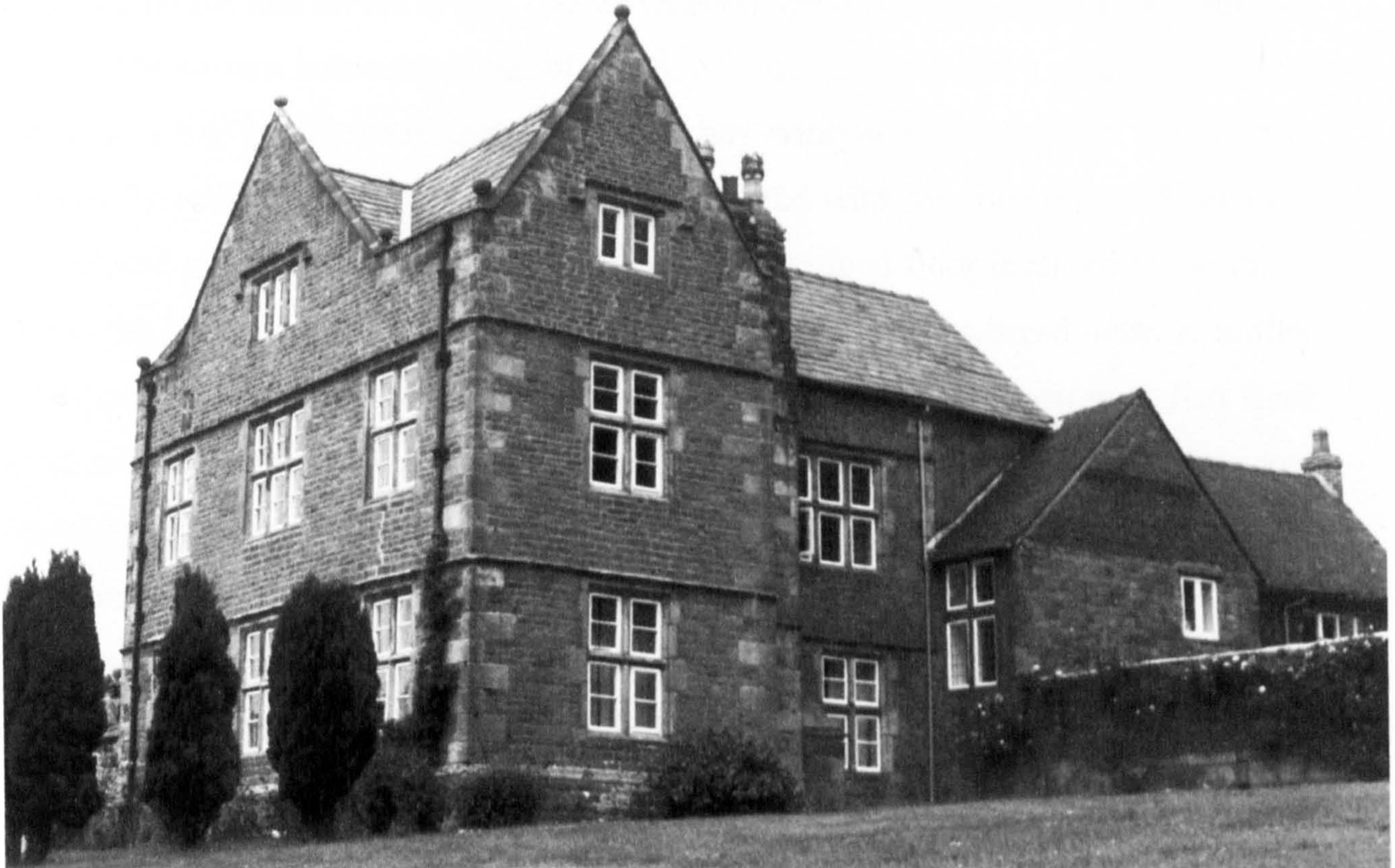
Fig. 6.26 Rudyard Hall from the southwest. The two-storey gable conceals the truncated remains of a timber-framed house whose plinth continues as the base of the garden wall. The hall and parlour wing were built towards the end of the seventeenth century.
