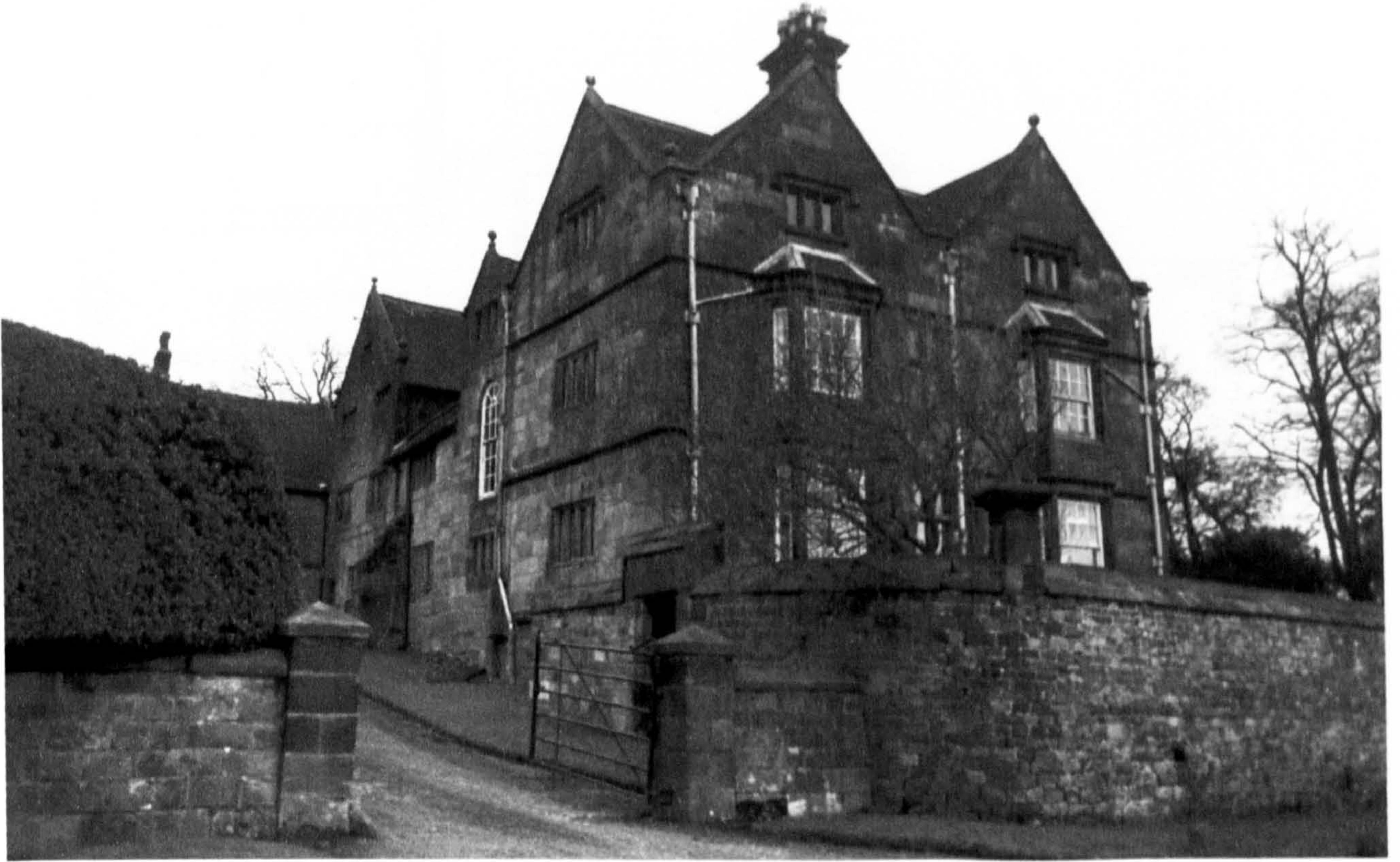
Fig. 6.25 Horton Hall from the west showing the slope of the land.
