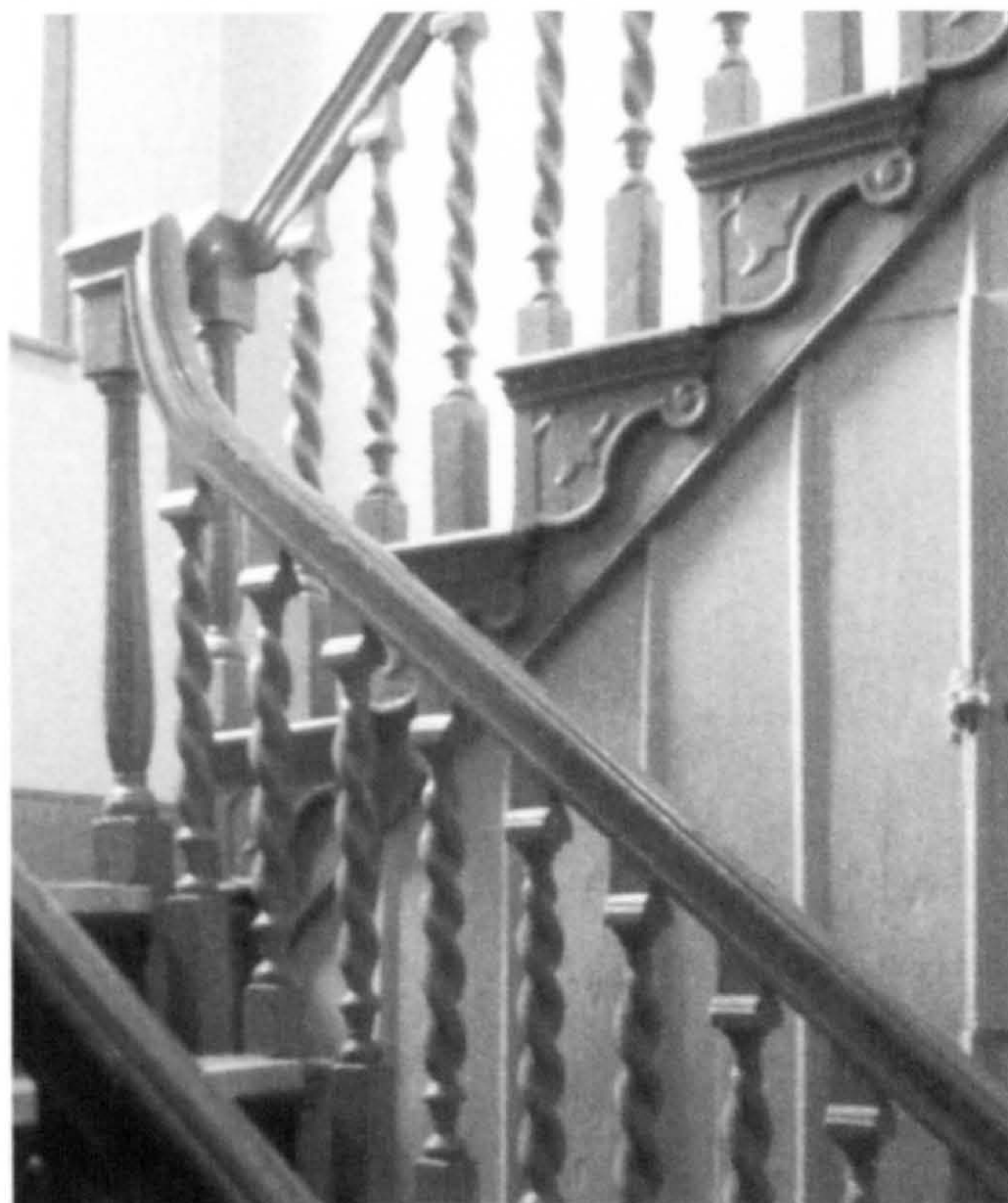
Fig. 6.138 The staircase at 62 St. Edward's Street.
