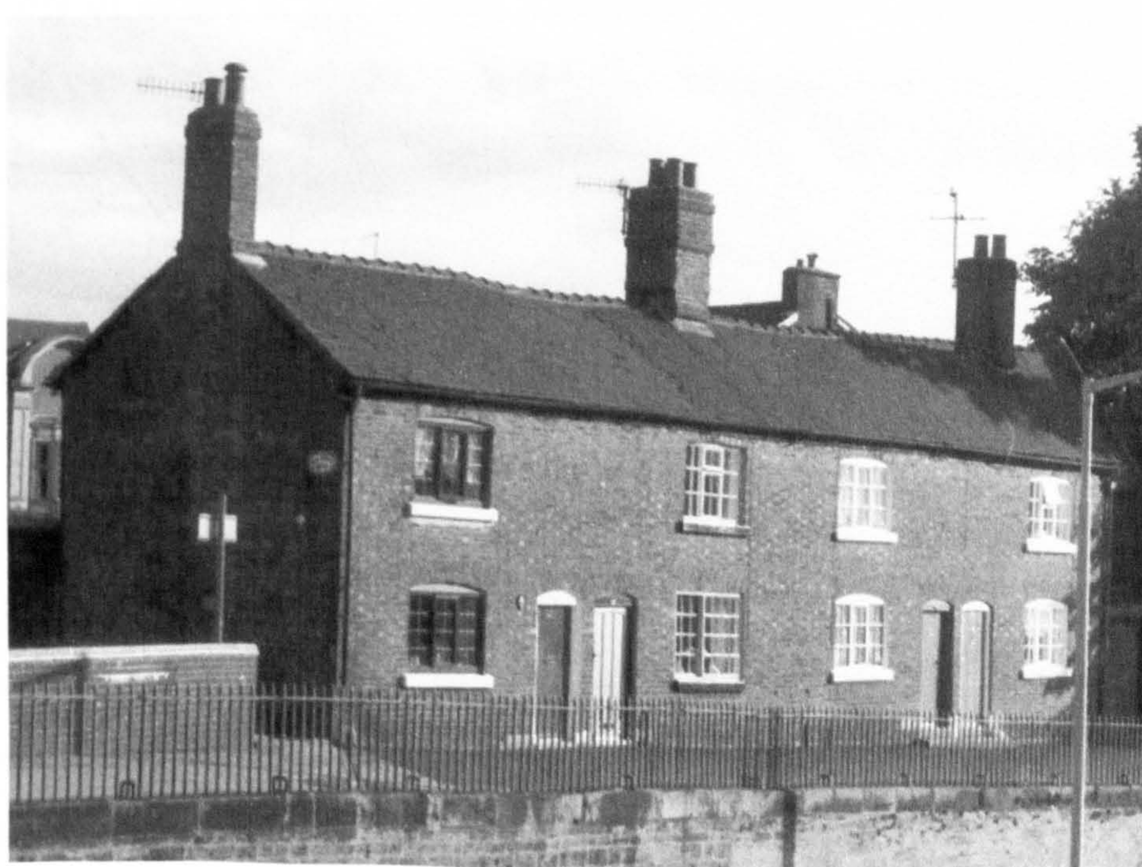
Fig. 6.128 5-8 Overton Bank, the 'Quaker cottages'
