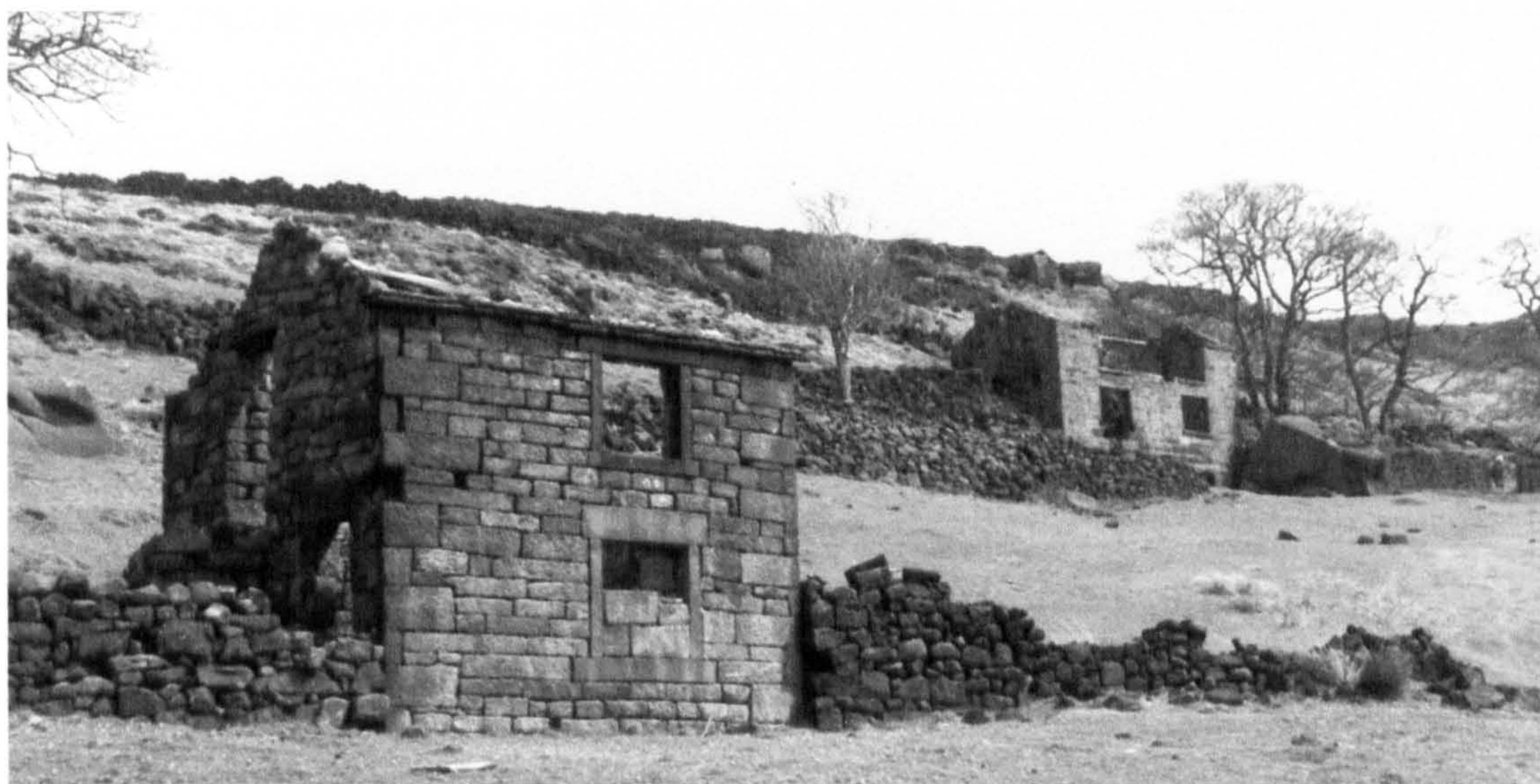
Fig. 6.89 Roche End, Leekfrith: a single cell cottage in the foreground. Behind it is the house of Henry Mills with housing for cattle below it. The roofs were removed before 1975 at the order of Sir Philip Brocklehurst in order to deter squatters.
