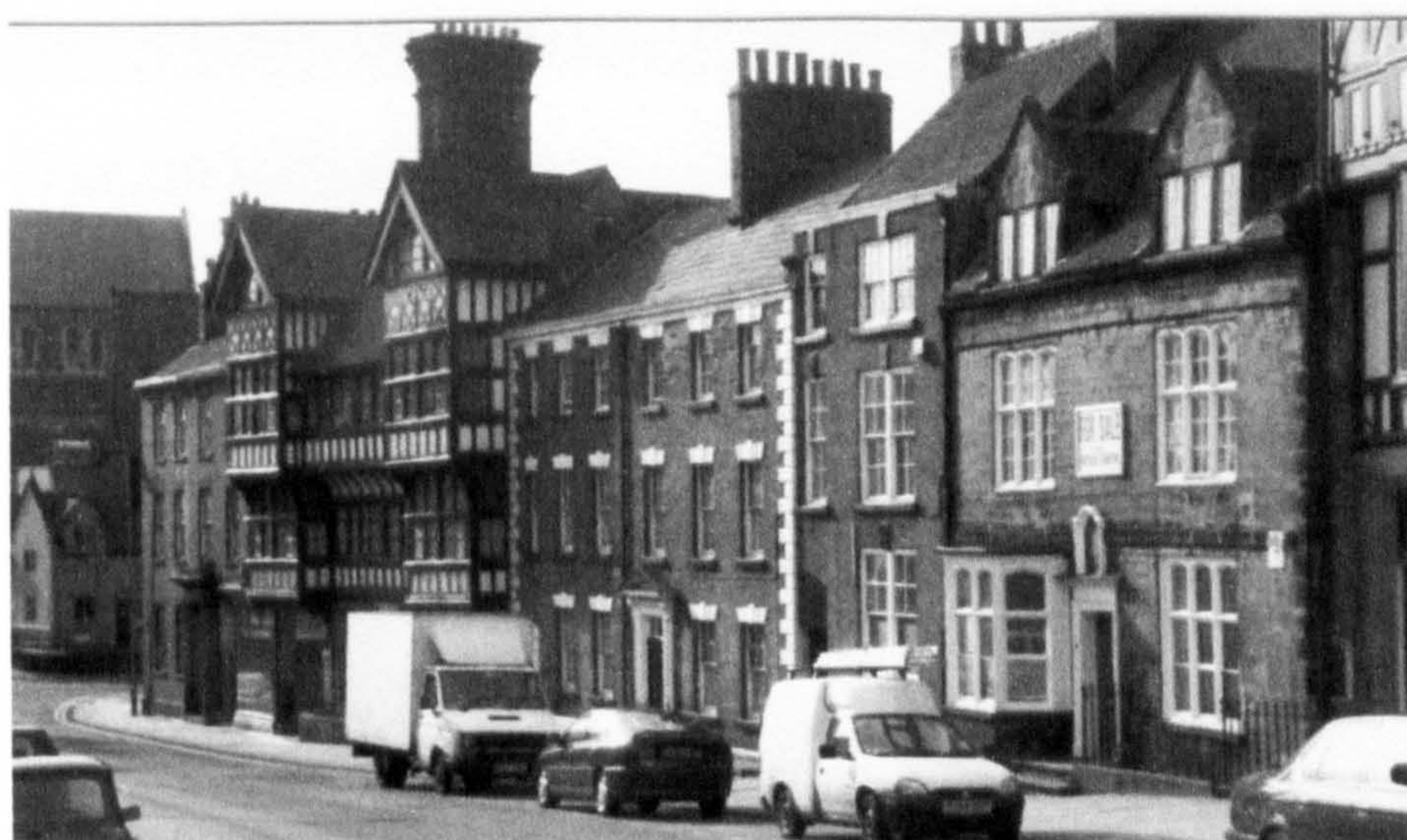
Fig. 6.116 St. Edward's Street with No. 62 to the right and No. 64 in the centre
