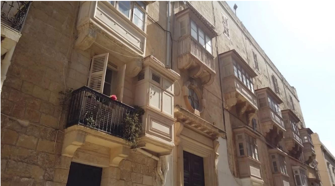
Figure 52 - The 'Gallatrina' - Or Balcony-Toilet - identifiable by its opaque windows and plumbing. (Source: Author's Own)
