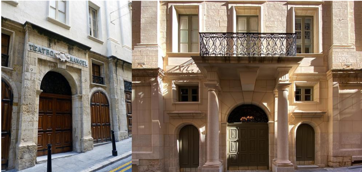
Figure 39 - Manoel Theatre before (left) and after (right) restoration (Composite by author).
