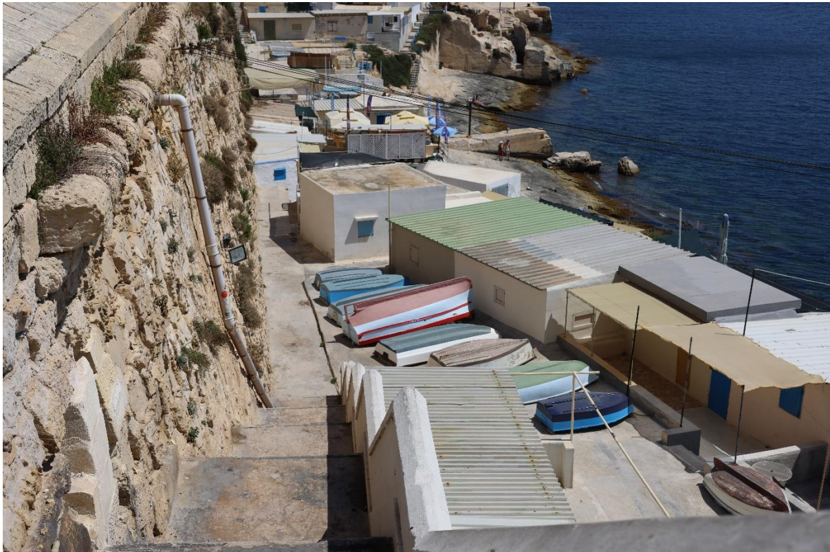
Figure 50 - Boat and summer houses built on the shore under the bastions. These face the Grand Harbour (Source: Author's own).
