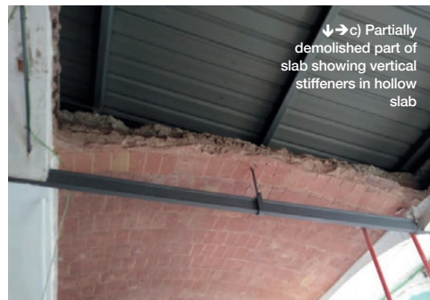
↑FIGURE 5: Catalan vaulted slab system in old weaving mill in Vilassar de Dalt, Spain
