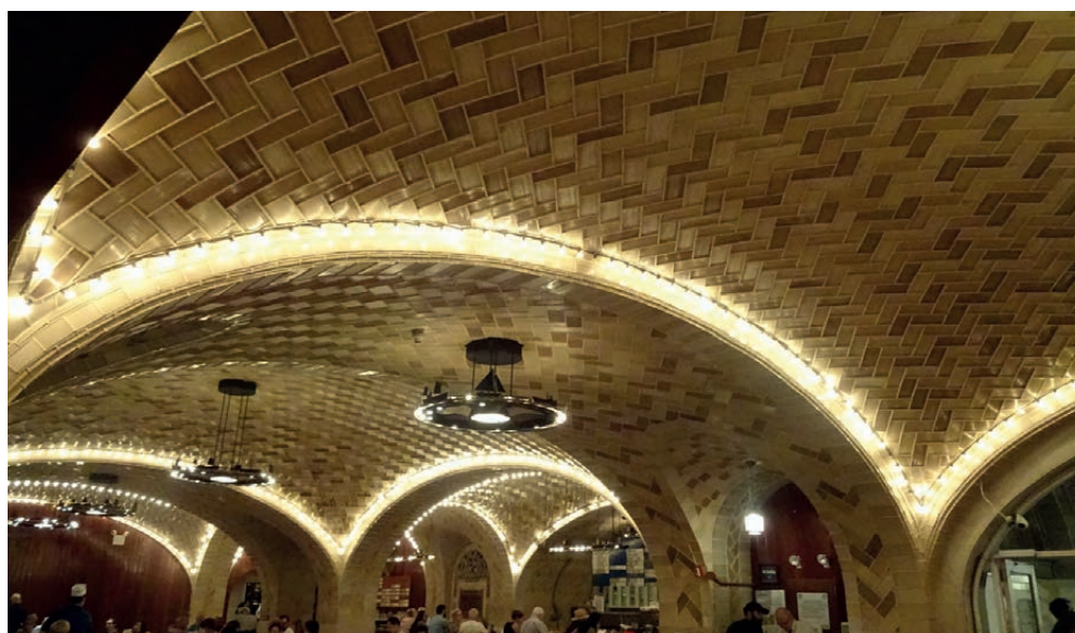
↙ FIGURE 3: Guastavino vaulted ceiling at Oyster Bar in Grand Central Station, New York
