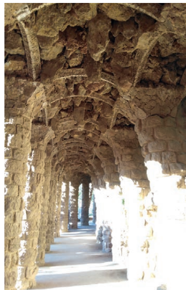
b) Vaulted viaduct
