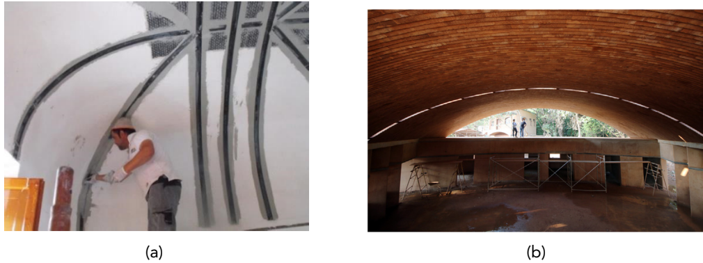
Figure 1.1: Way forward for building and construction industry; (a) restore and strengthen existing structures—application of CFRP strips to strengthen a masonry vault (after [5]); (b) build efficiently with efficient structural forms and low carbon materials—15m span earthen shell roof (after [6]).
