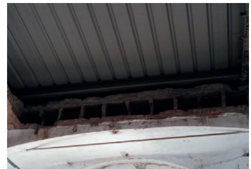
↑FIGURE 5: Catalan vaulted slab system in old weaving mill in Vilassar de Dalt, Spain
