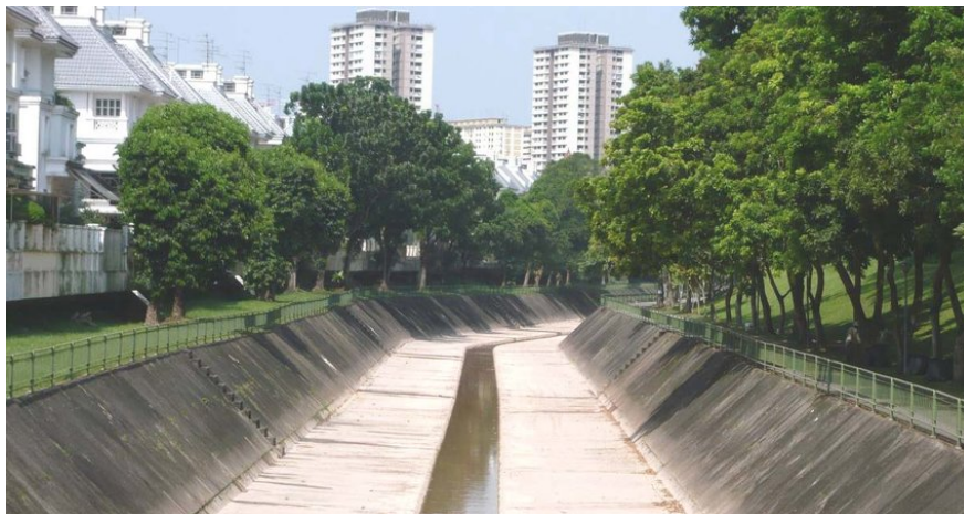
Figure 2.2: Typical open channel drainage with the cunette visible. Image of Ulu Pandan ‘Canal’ in Singapore (Tan and Yeo, 2009).
