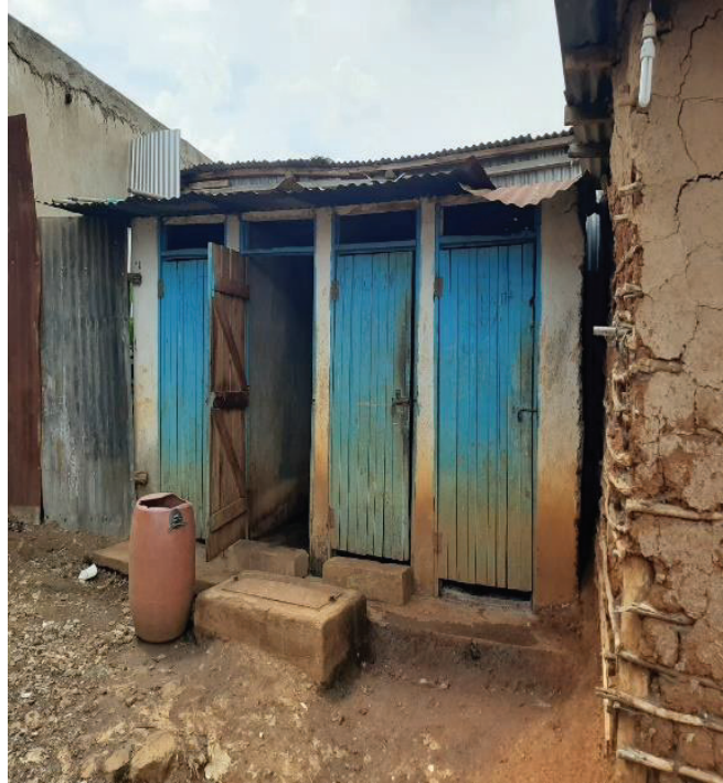
Figure 24: A toilet block in a household compound in Langas (Source: Author)
