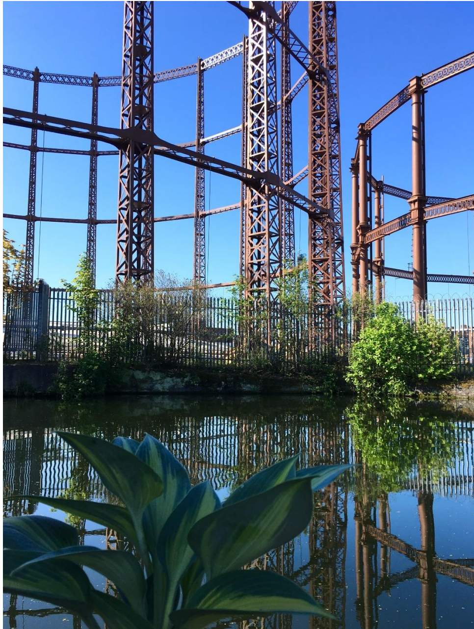
Figure 92. Regent's canal, Broadway market. Gas chambers reflected in the canal surface water. 2020.
