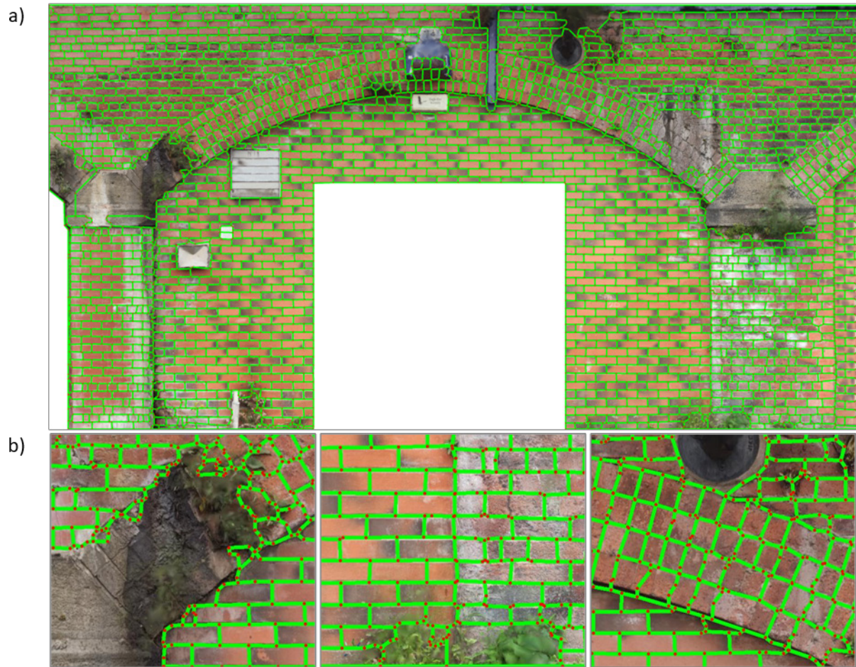
Fig. 4.27: Final generalized-lines (Red-Points: Vertices of the lines); a) Overall view; b) Zoomed-in view.
