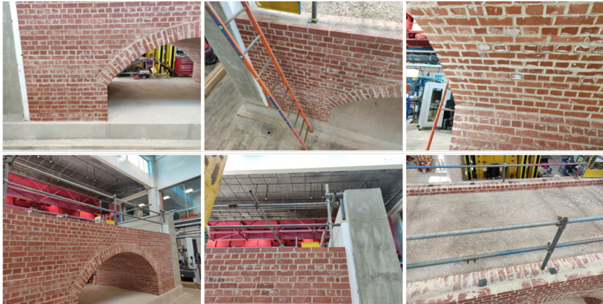
Fig. 6.1: Sample images used for photogrammetry of the full-scale masonry arch bridge constructed in the laboratory.
