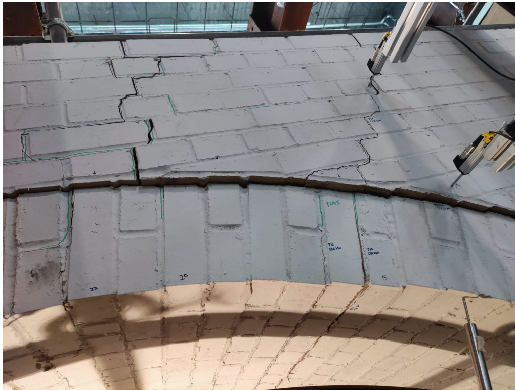
Fig. 6.11: Recorded crack pattern after multiple tests on the experimental arch-bridge.
