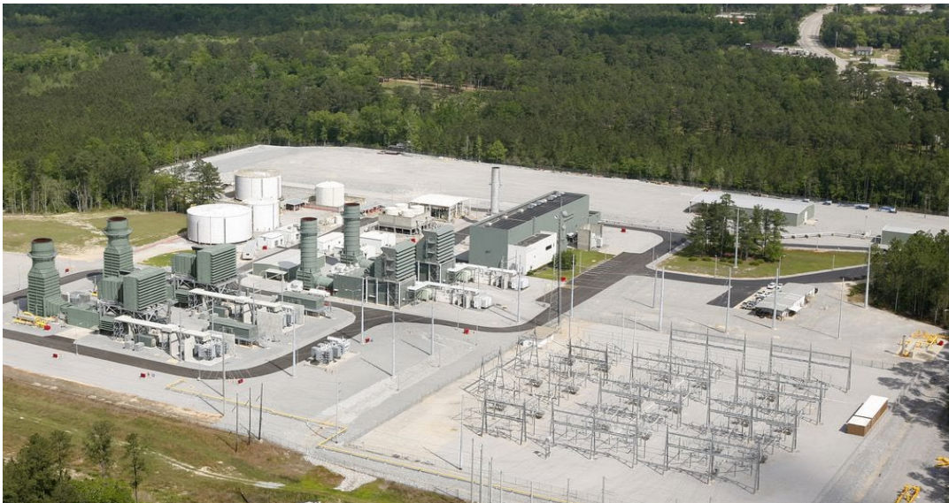
Figure 2-2 McIntosh CAES plant (Venkataramani et al., 2016)
