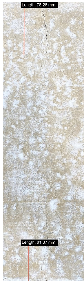
Figure D.19: IC crack length at 24 hours of PFC.
