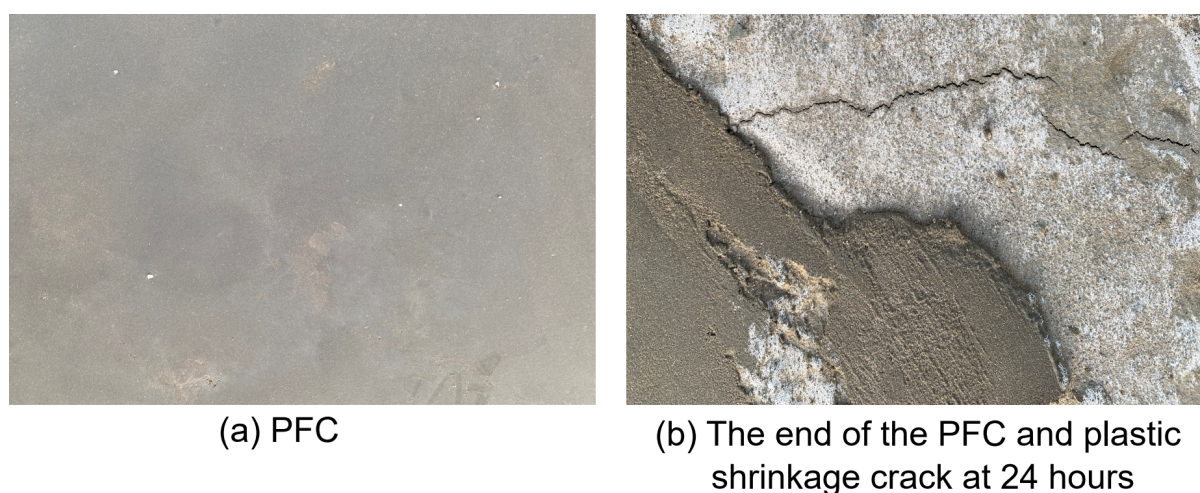
Figure 5.9: Power floating concrete of big scale.
