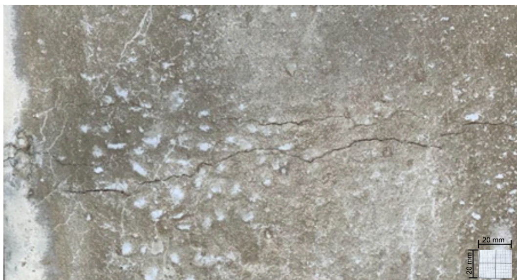
Figure 4.12: Typical crack pattern in plain concrete (PC) specimens of high temperature examined at 24 h.
