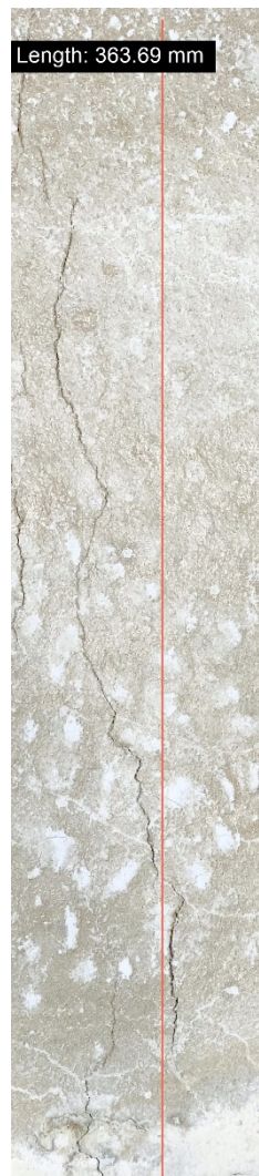
Figure C.7: IC crack length at 24 hours of plain concrete (A).
