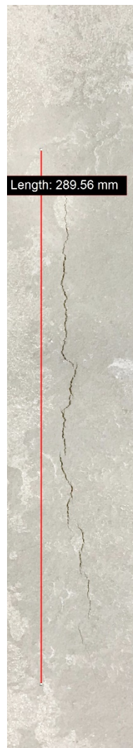
Figure C.28: IC crack length at 24 hours of HWSRTSFC30.
