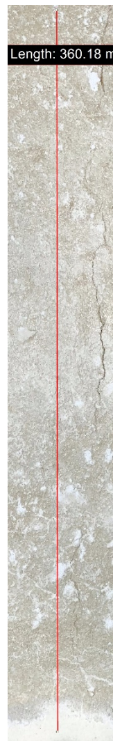
Figure C.10: IC crack length at 24 hours of plain concrete (B).
