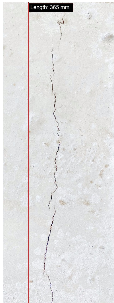
Figure B.8: IC crack length at 24 hours of plain concrete.
