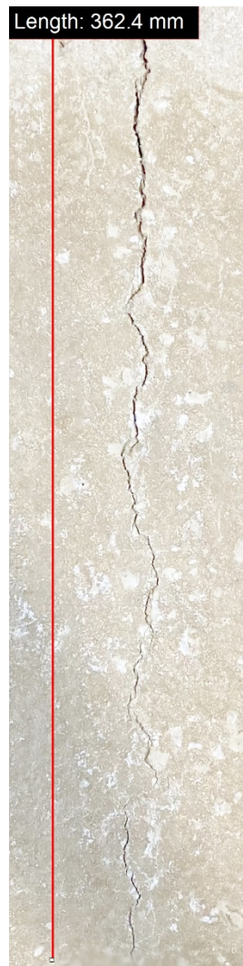
Figure D.25: IC crack length at 24 hours of CWC.
