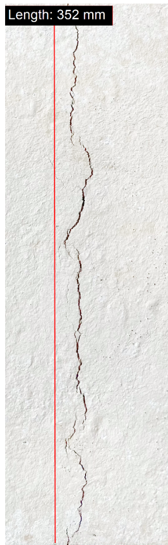
Figure B.20: IC crack length at 24 hours of MSFC10.
