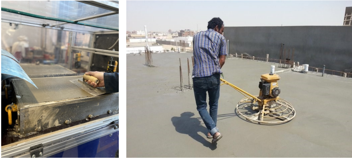
Figure D.3: Power floating of both scales (lab and in-situ)
