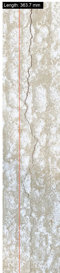
Figure D.16: IC crack length at 24 hours of plain concrete.
