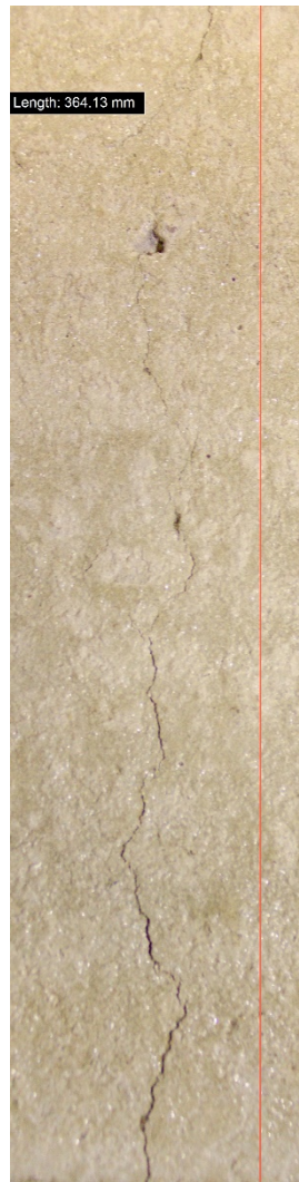
Figure C.34: IC crack length at 24 hours of plain concrete.
