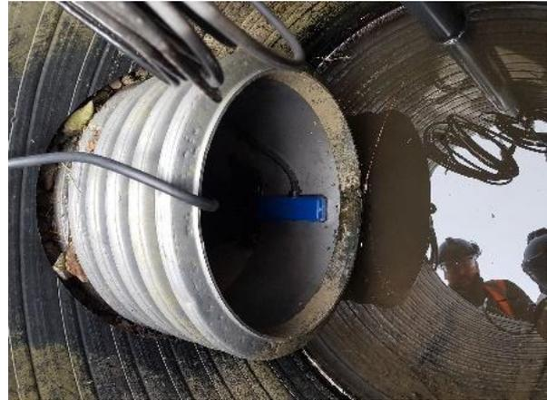
(b) Flow meter between catchpit 4 and 5
