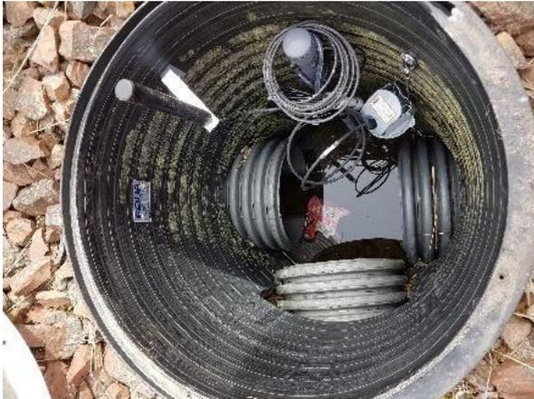
(a) Water depth sensor at catchpit 4
