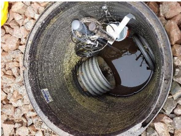
(c) Water depth sensor at catchpit 5
