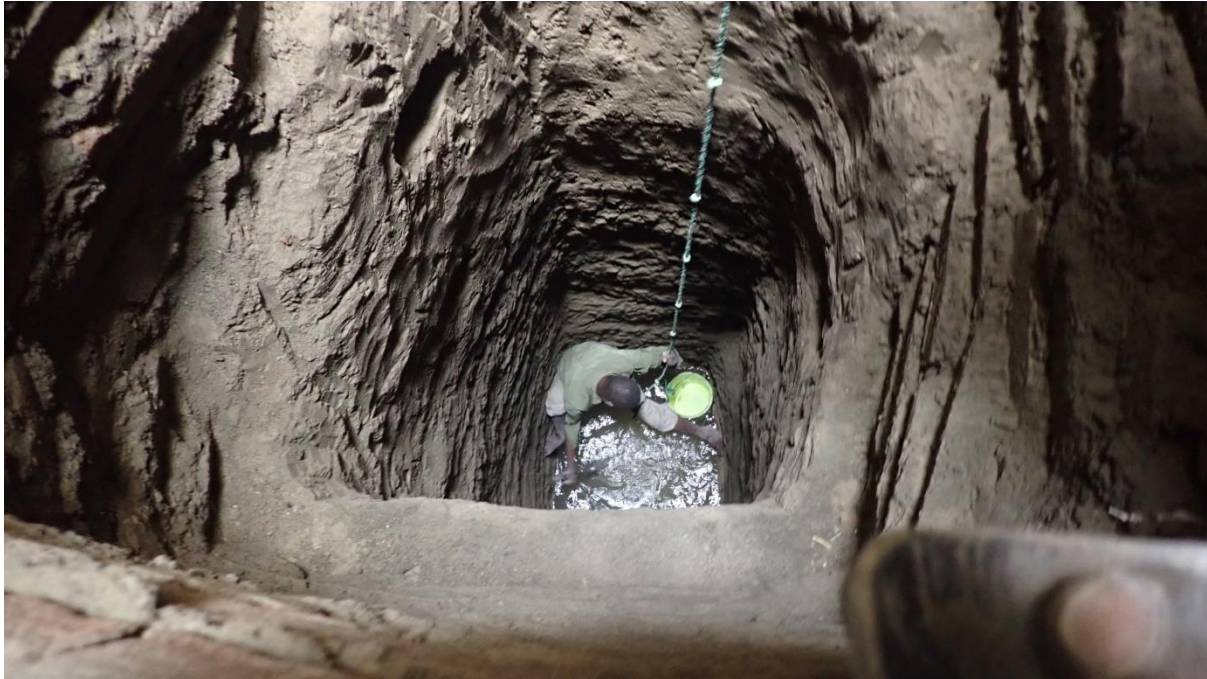
Figure 2 – A well digger engaged in the kuzibua process holding the safety rope
