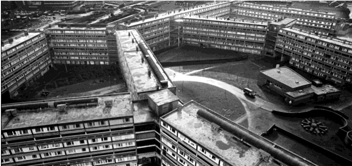
Figure 70. the Divis Flats complex, 1982. Photograph by Judah Passow.
