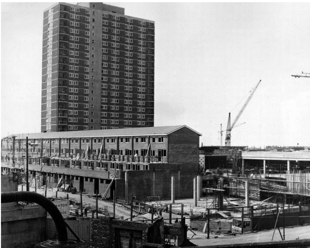
Figure 34. Building work on the New Strand June 1967.
