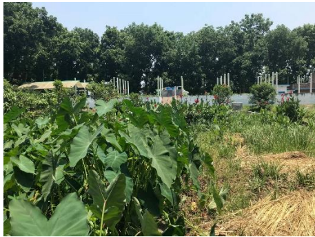
Figure 10: Jhenaidah Faecal Sludge Treatment Plant
