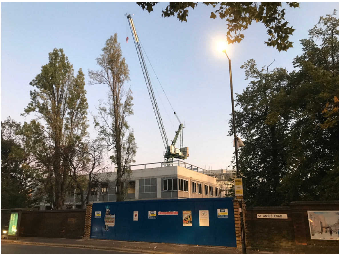
Image 19: Construction of new NHS facilities, St Ann's Hospital, Autumn 2019
