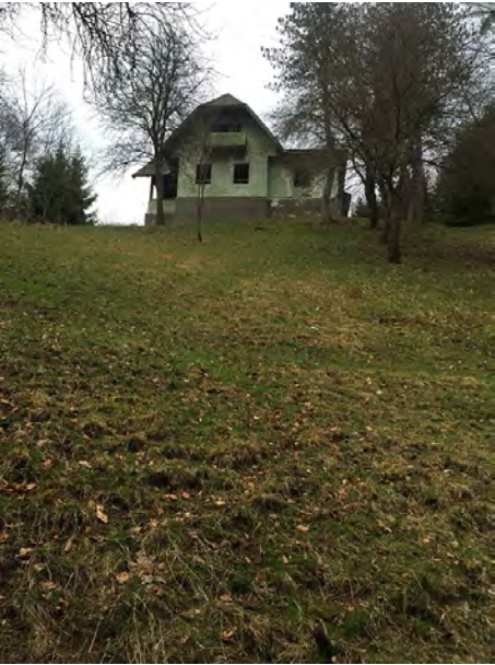
18 Living in the forest, formerly occupied by forestry engineers and their families.
