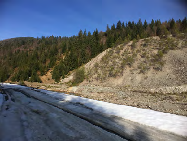
20 Ecological restoring of a former landfill
