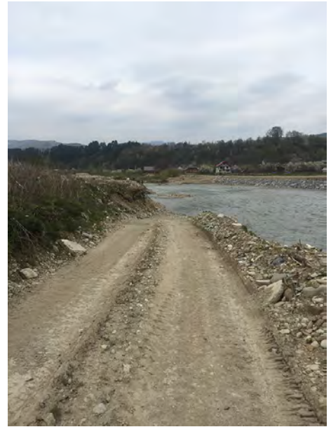
2 Extraction road for sand from the Vișeu river, Vișeu de Sus
