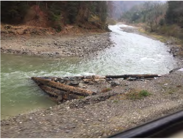
8 Vaser river, wooden dam structure
